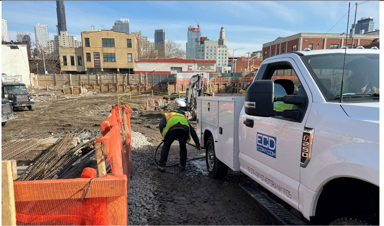
Photo 4 – Representative photo of cleaning the tires of a car onsite on track pad.
