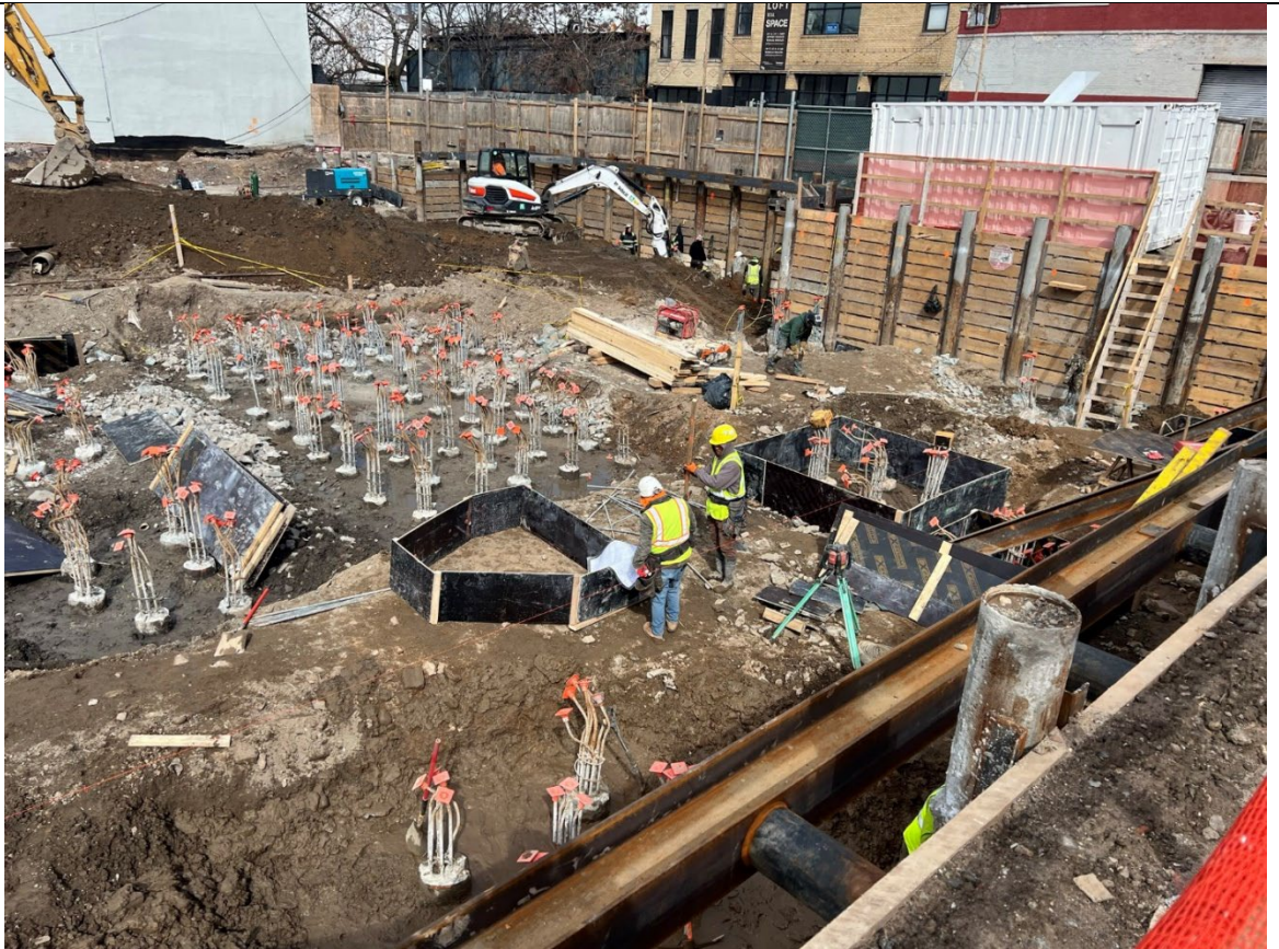
Photo 2 – Representative photo of workers installing boxes around pile caps for concrete.
