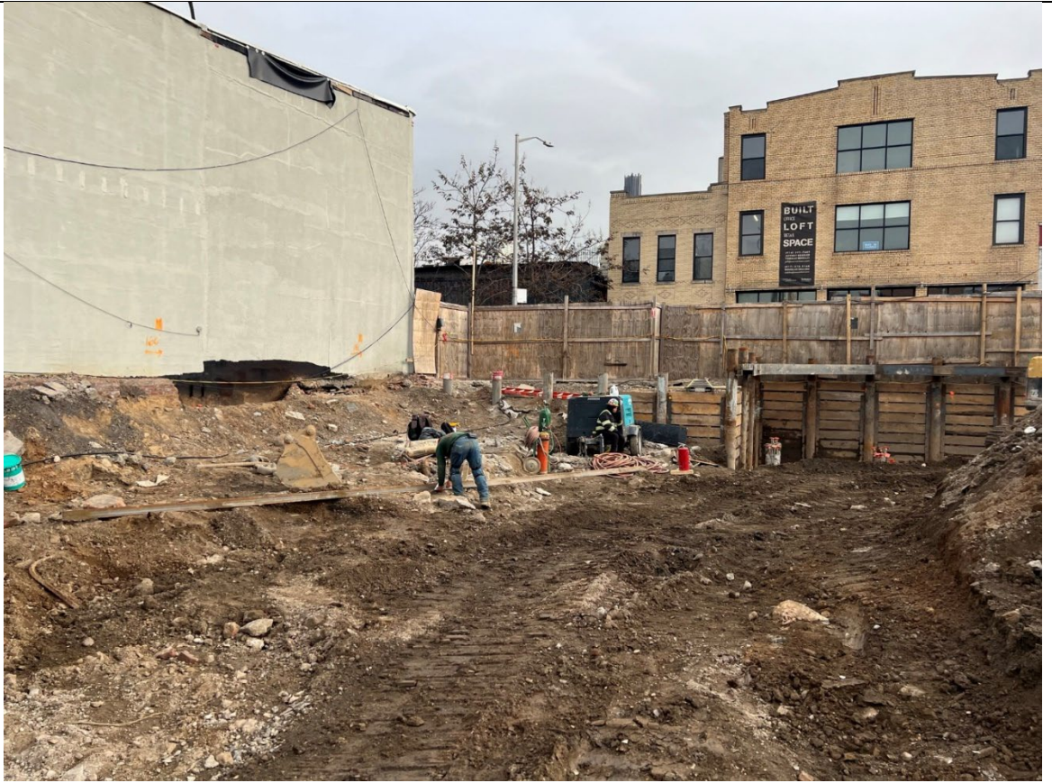
Photo 1 – Representative photo worker cutting a piece of metal for lagging.
