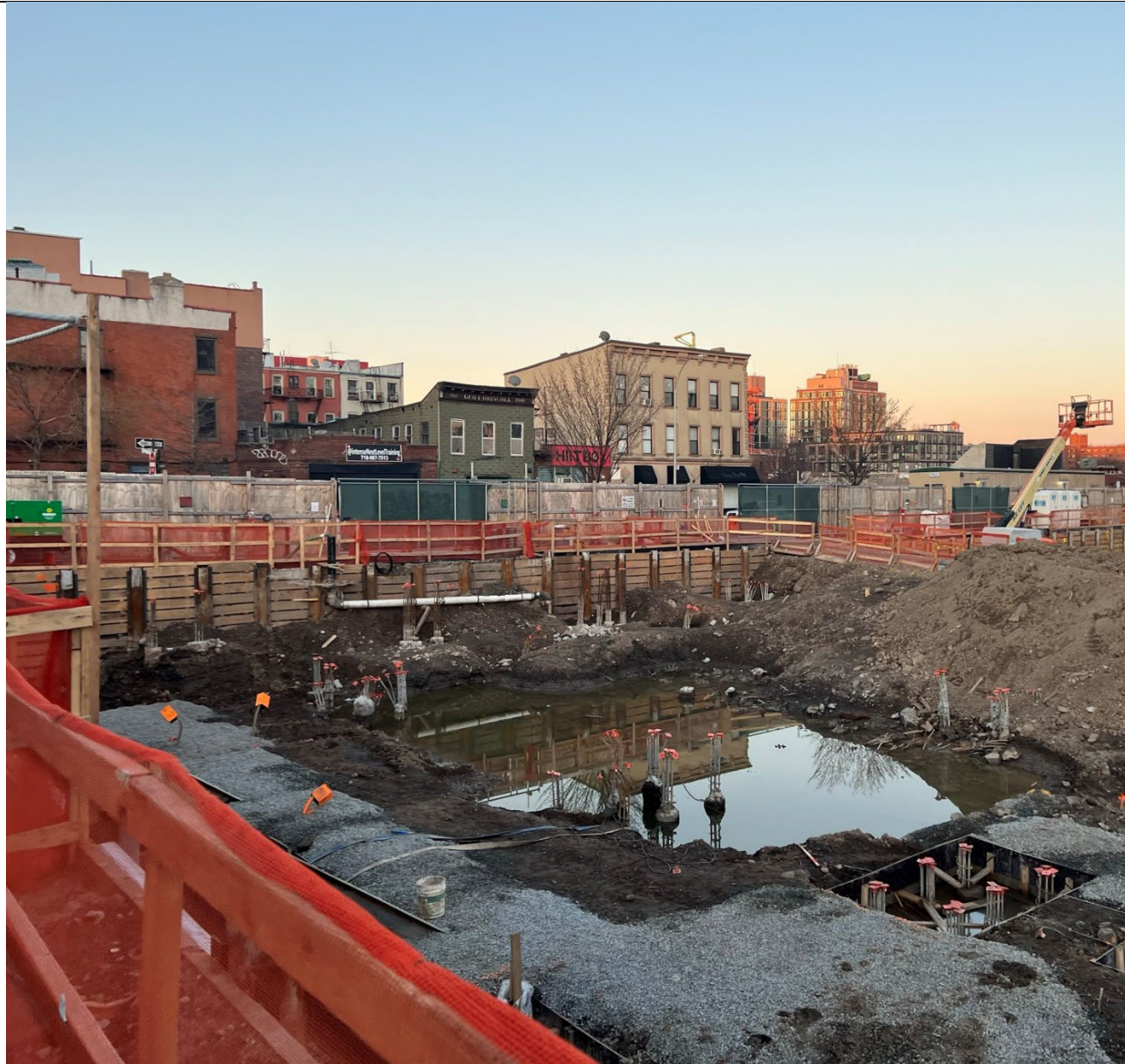
Photo 1 – Representative photo of the Site before work activities begin.
