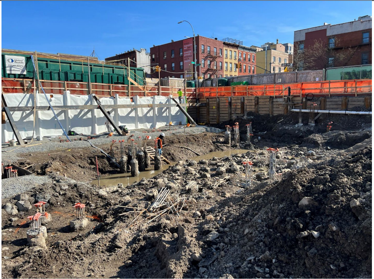
Photo 2 – Representative photo of water drained from elevator pit, via dewatering process.
