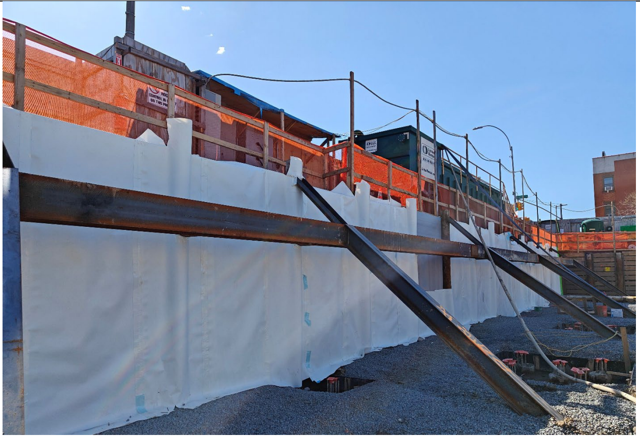
Photo 6 – Additional view of Preprufe waterproofing installation.
