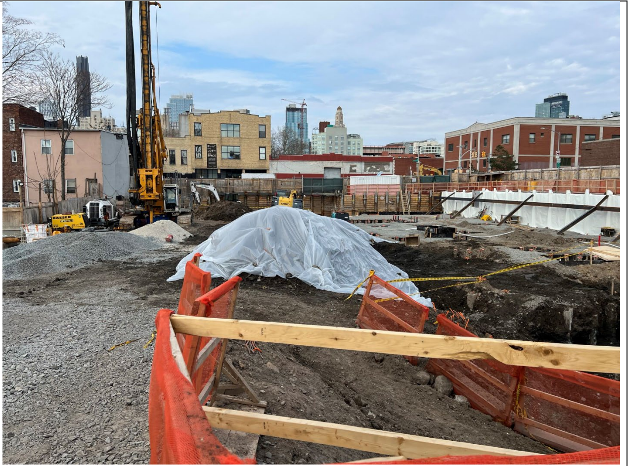
Photo 4 – Representative photo of stockpiled material from within the petroleum impacted area covered with poly at the end of the days activities.
