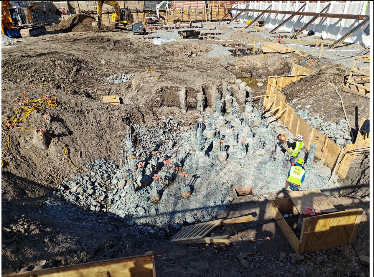
Photo 3 –View of ongoing pile work.
