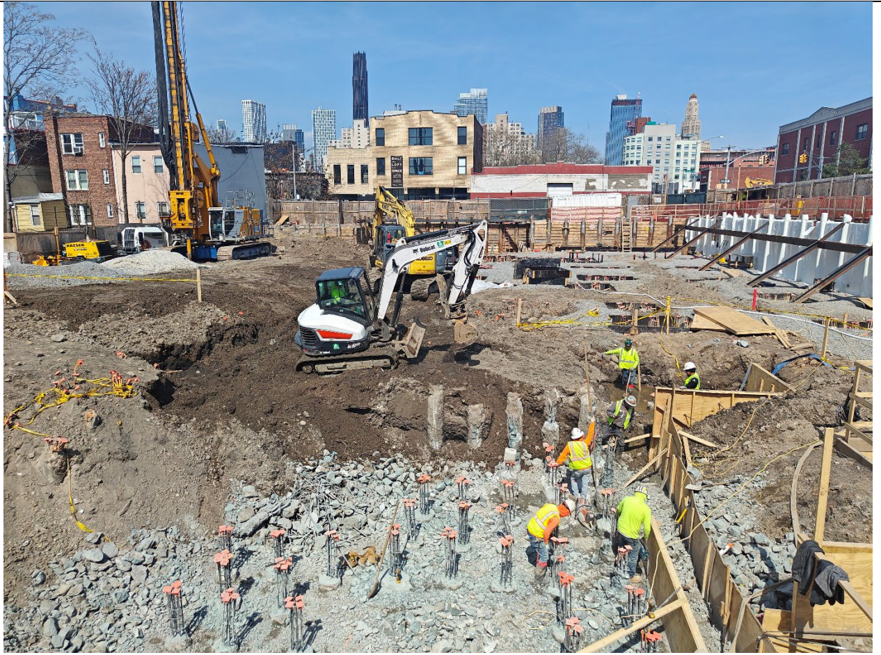
Photo 3 – Representative view of excavation within petroleum impacted portion of the Site and pile work.
