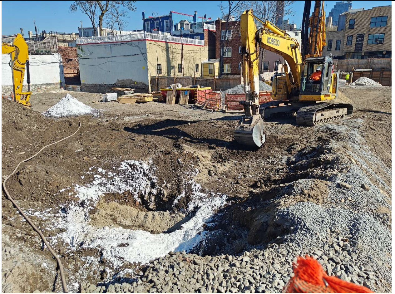
Photo 5 – Representative photo of trucking ramp being moved.
