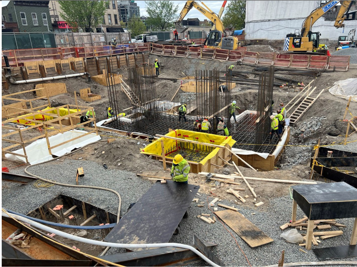
Photo 1 – Representative view of rebar work in the elevator pit.
