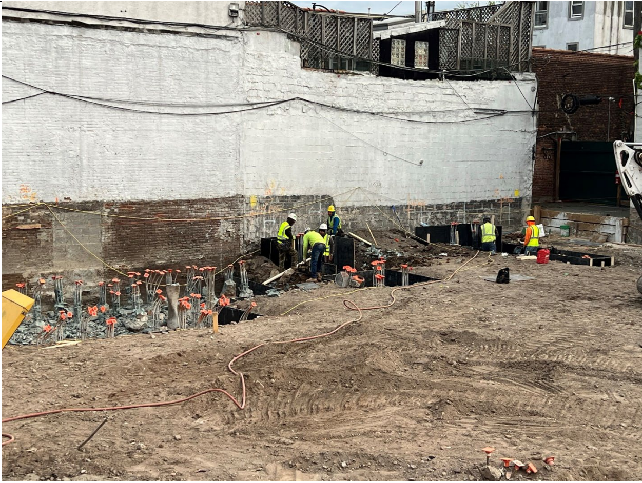
Photo 2 – Representative view of forming piles in WC-1.
