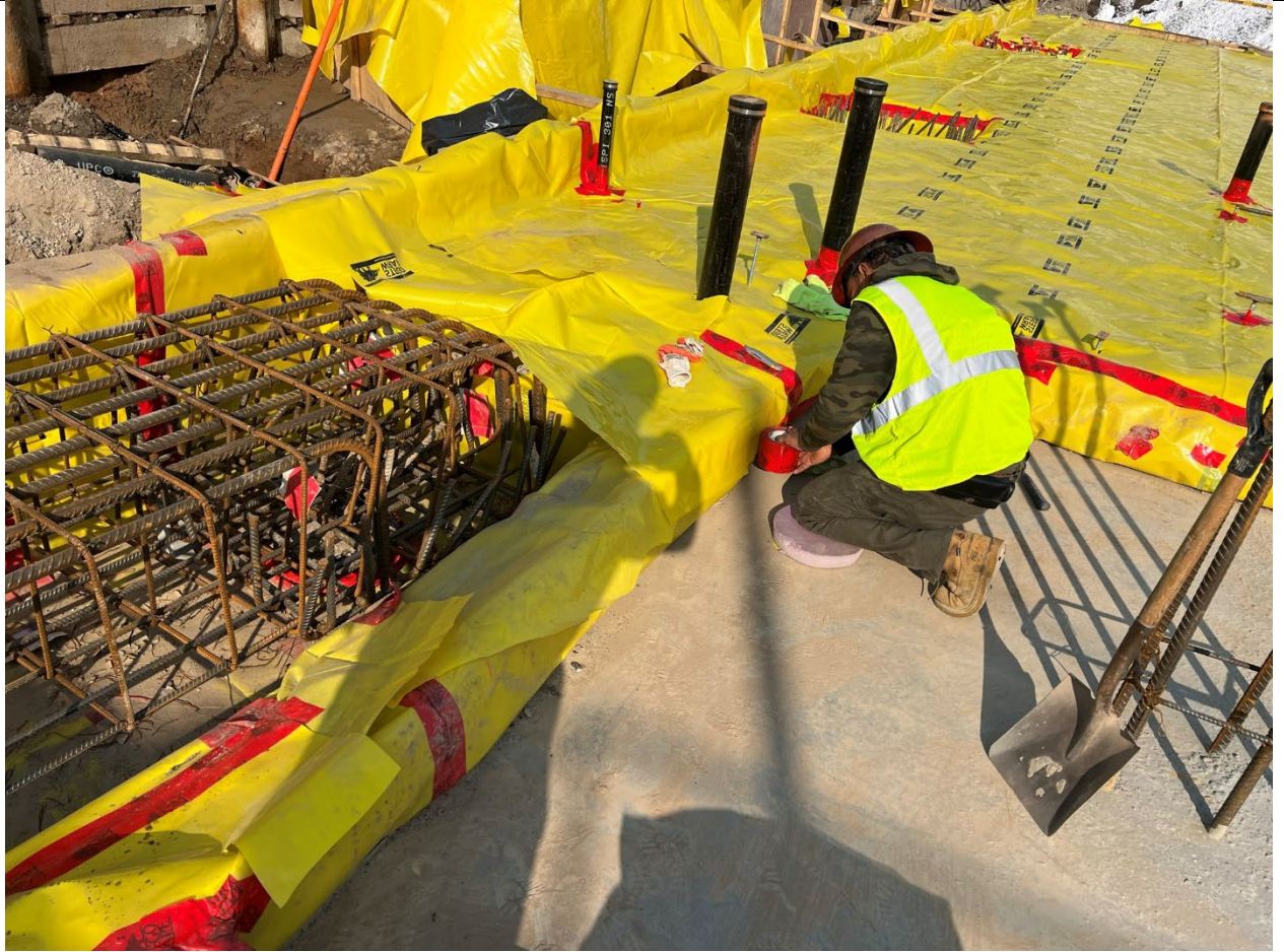
Photo 1 – Representative photo of worker installing STEGO wrap.
