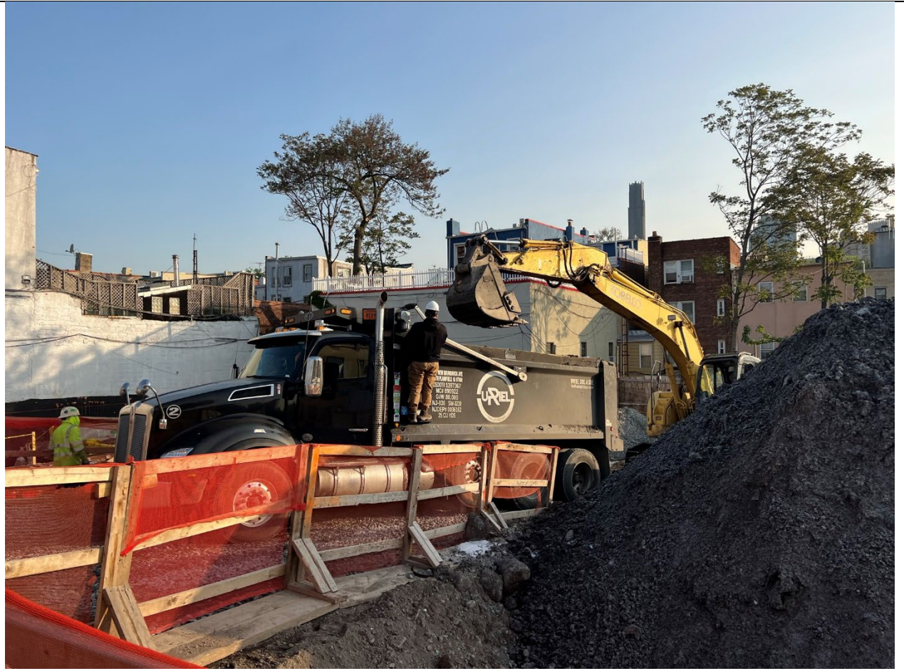
Photo 2 – Representative view of soil stockpile and trucking activities.
