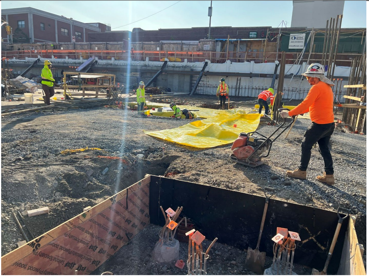
Photo 1 – Representative photo of STEGO wrap being laid in WC-4.
