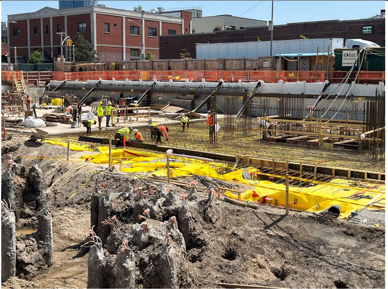
Photo 2 – Representative view of rebar work in WC-4 and WC-5.
