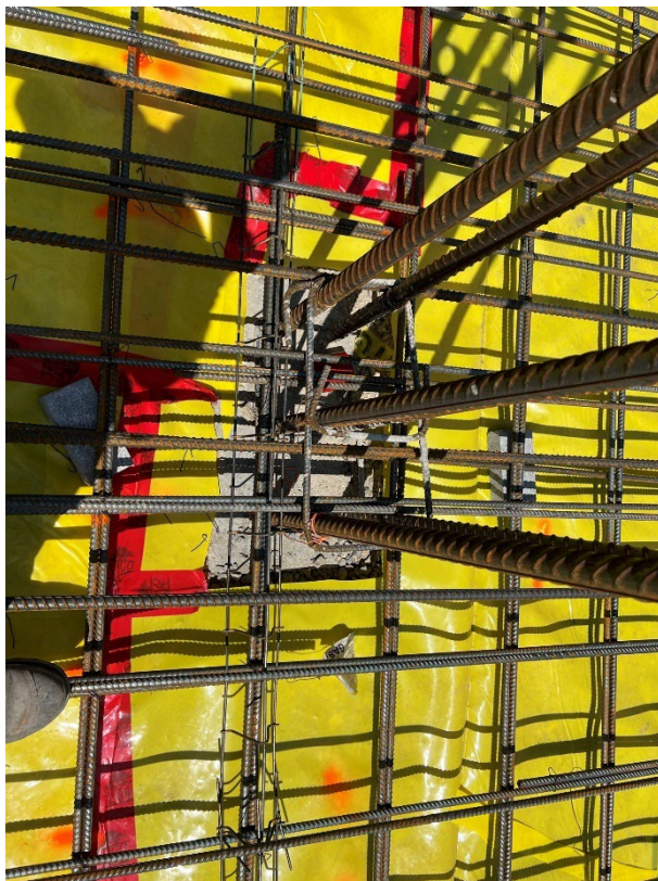
Photo 9- Representative photo of before and after of fixing a seal around a column.
