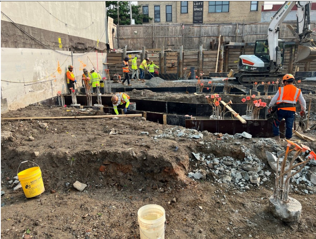
Photo 2 – Representative view forming piles in WC-6.
