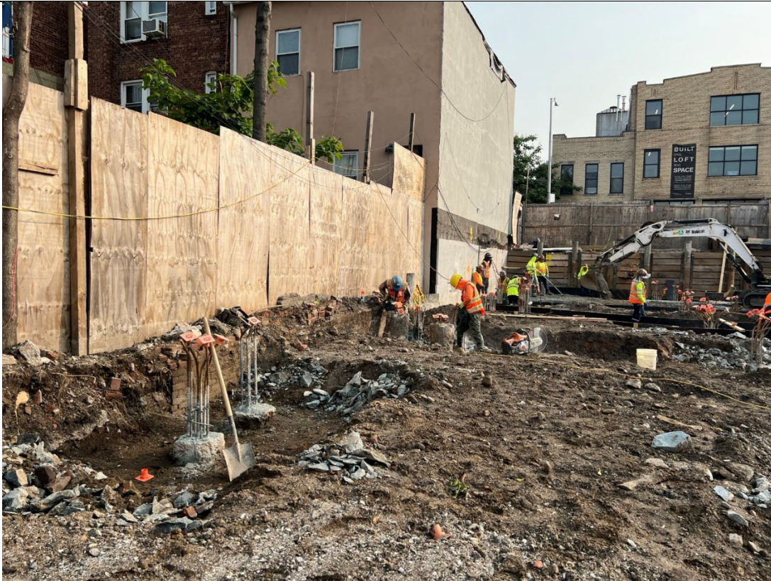
Photo 1 – Representative photo of pile cap work in WC-6.
