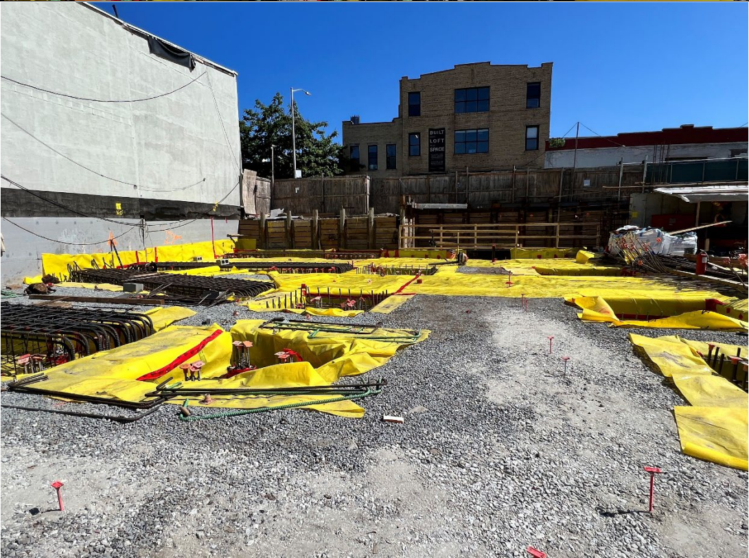
Photo 4 - Representative photo of continued rebar and vapor barrier work.
