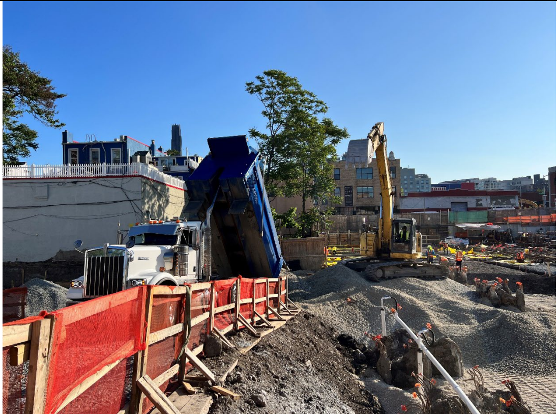
Photo 2 – Representative photo of backfill delivery.
