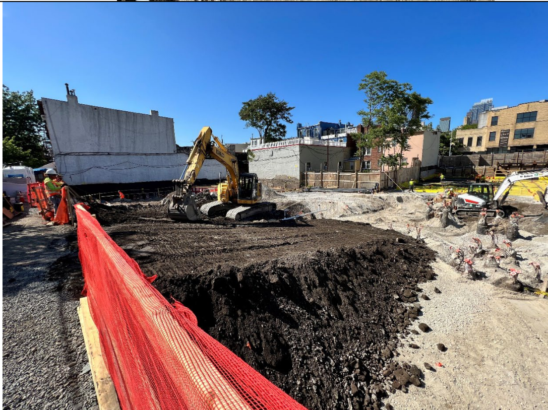
Photo 6 - Representative photo of the relocated construction ramp.
