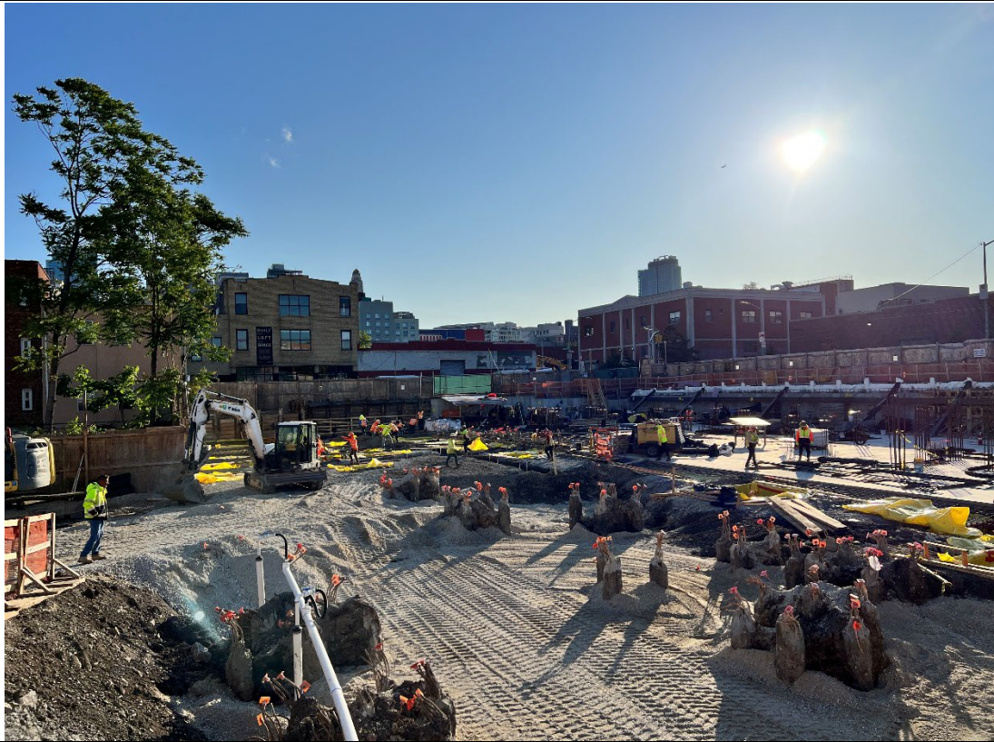
Photo 1 – Representative photo of Site at beginning of work day.
