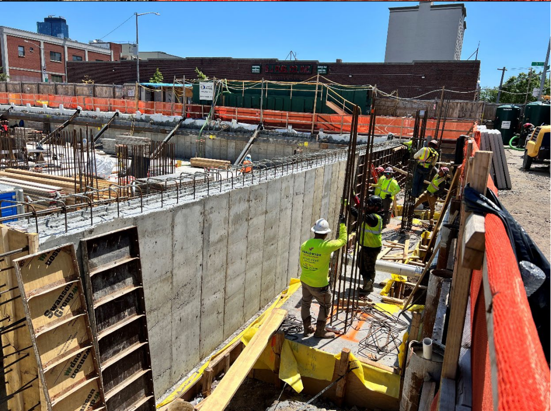
Photo 4 - Representative photo of workers stripping formwork from foundation walls.
