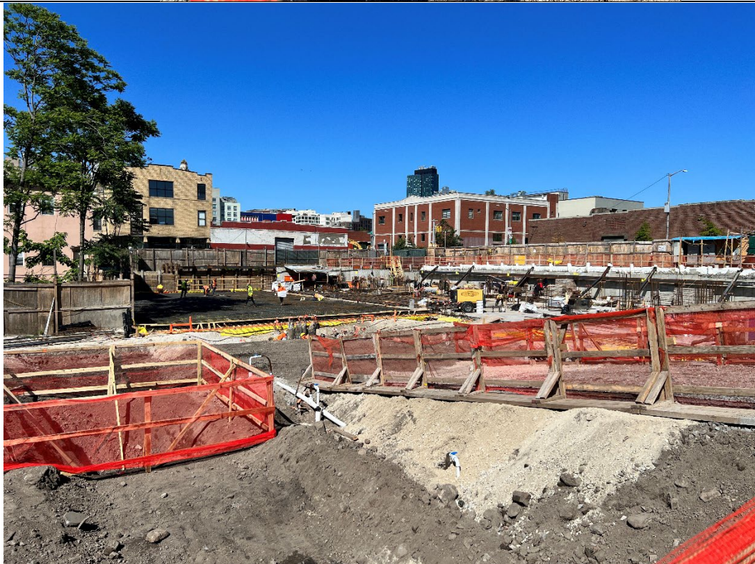
Photo 6 - Representative photo of site at end of day.
