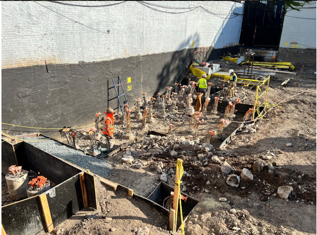
Photo 2 – Representative photo of exposing pile caps in WC-1.
