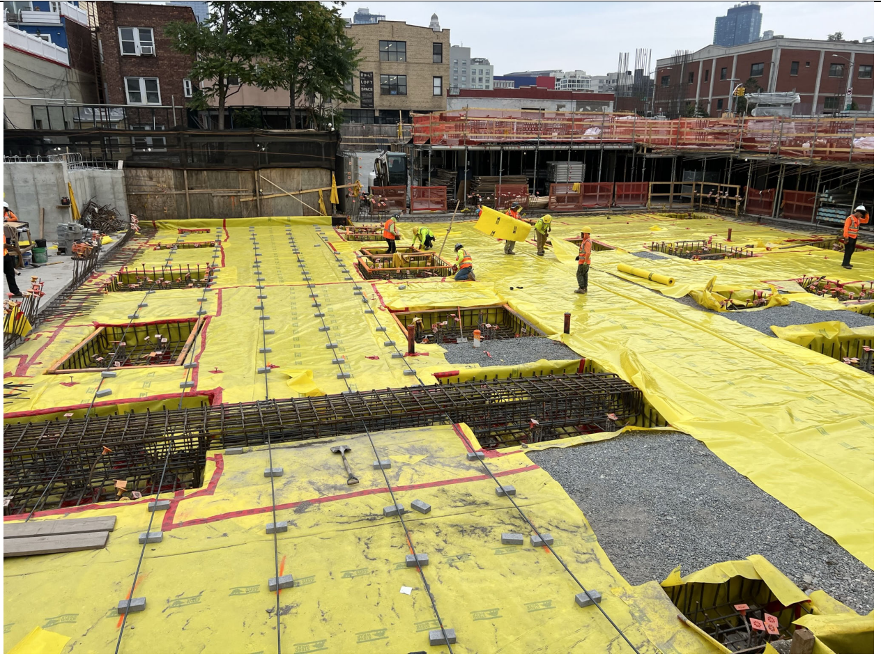
Photo 3 – Representative photo vapor barrier being laid in WC-3.
