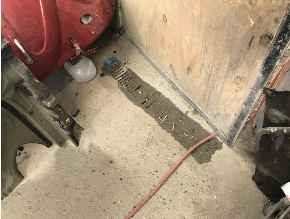
A clogged floor drain that reportedly is connected to the municipal sewer system.
