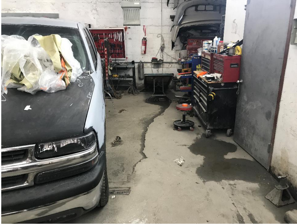
A view of the concrete slab within the auto body shop. Generally, the concrete slab appeared to be in good condition with some puddling and staining.
