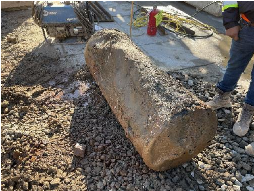
Figure 3: UST002 removed from the ground.
