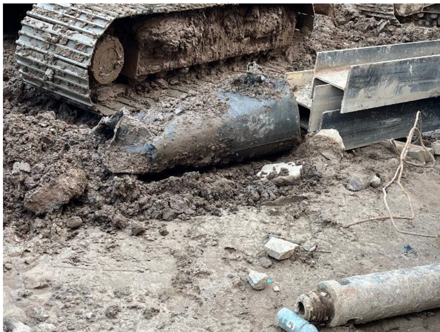
Figure 1: UST001 removed from the ground.
