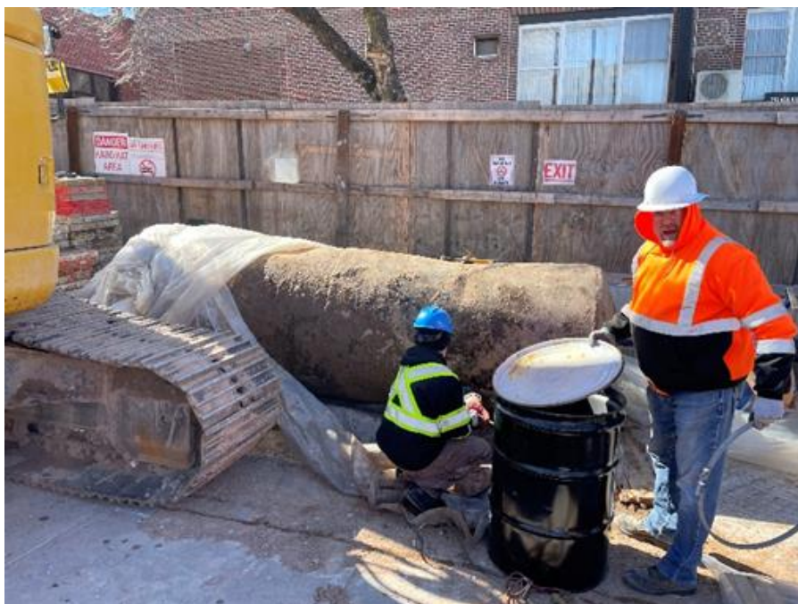
Figure 6: UST003 being cleaned prior to disposal.
