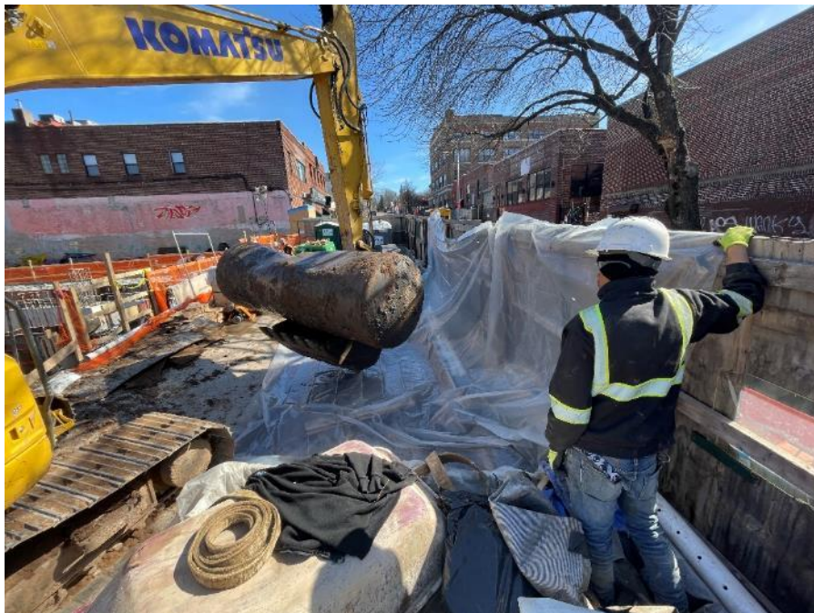
Figure 5: UST003 removed from the ground.
