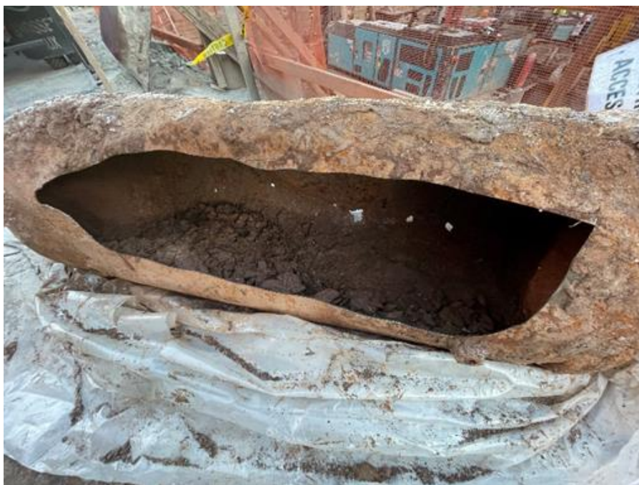
Figure 4: UST002 being cleaned prior to disposal.
