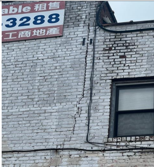
Photo 7: CRACK PROPAGATION AT EAST ELEVATION BETWEEN 262 AND 207
