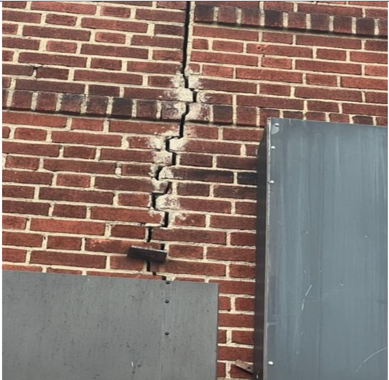
Photo 9: EXTENT OF CRACK AT SOUTH FAÇADE OF 207/209 BUILDING
