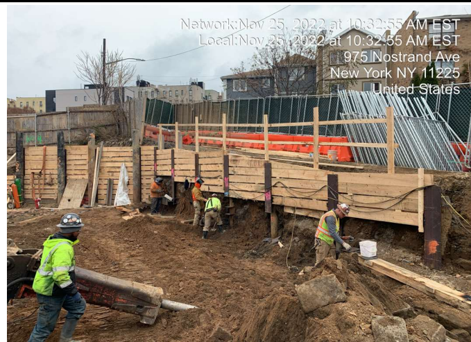
Photograph 3 - Lagging in Grids 2 and 6, facing northeast.
