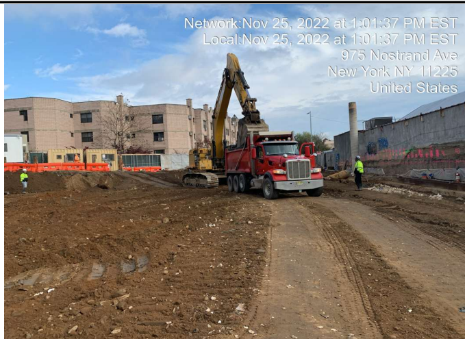
Photograph 2 - Loading soil onto trucks for disposal at BSM facility, facing east.
