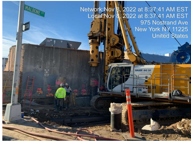
Photograph 1 - Secant pile installation, facing south.
