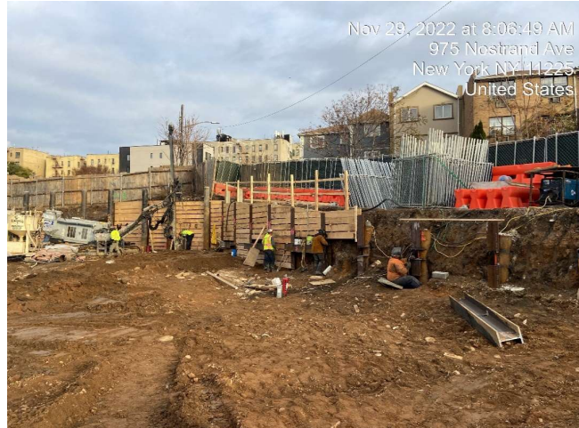
Photograph 3 - Installing lagging for SOE in Grid 6, facing northwest.
