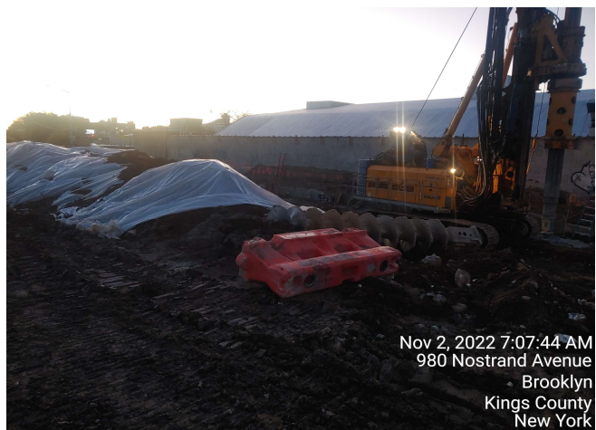
Photograph 3 - Soil stockpiles covered with poly sheeting.
