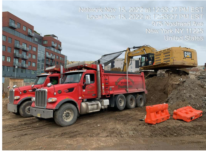
Photograph 1 - Loading of stockpiled material for disposal at BSM facility, facing north.
