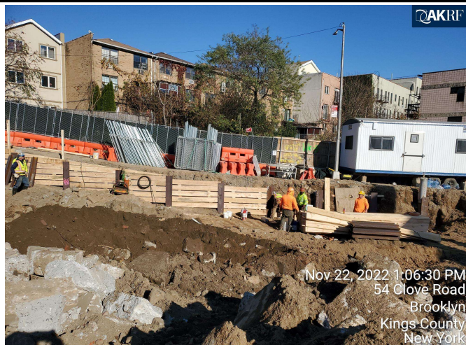
Photograph 3 - Installing lagging in Grid 6, facing northeast.
