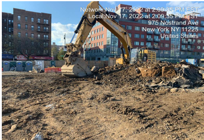
Photograph 2 - Contractor separating concrete from soil for future disposal, facing west.
