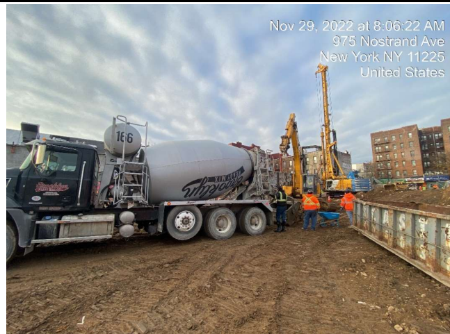
Photograph 2 - Concrete truck on Site for grouting piles, facing southwest.
