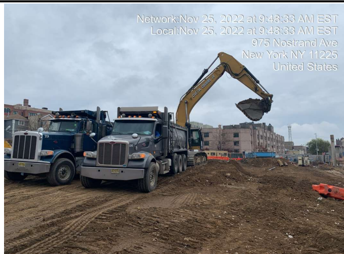
Photograph 1 - Loading soil on to trucks for disposal at BSM facility, facing east.
