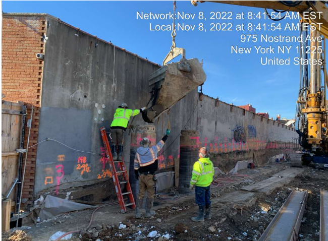
Photograph 2 - Secant pile installation continues (puring concrete), facing southwest.
