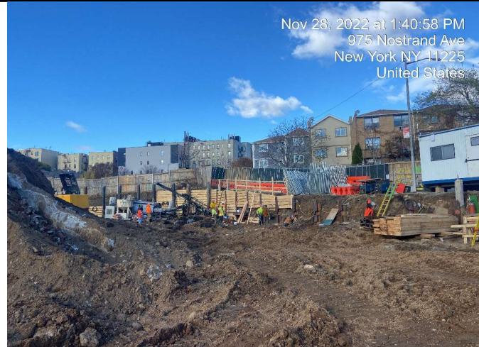
Photograph 3 - Installing lagging for SOE in Grids 2 and 6, facing northwest.
