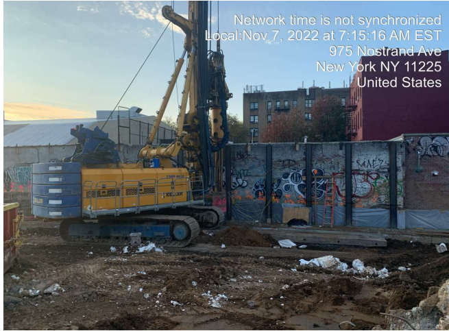
Photograph 1 - Secant pile installation, facing south.
