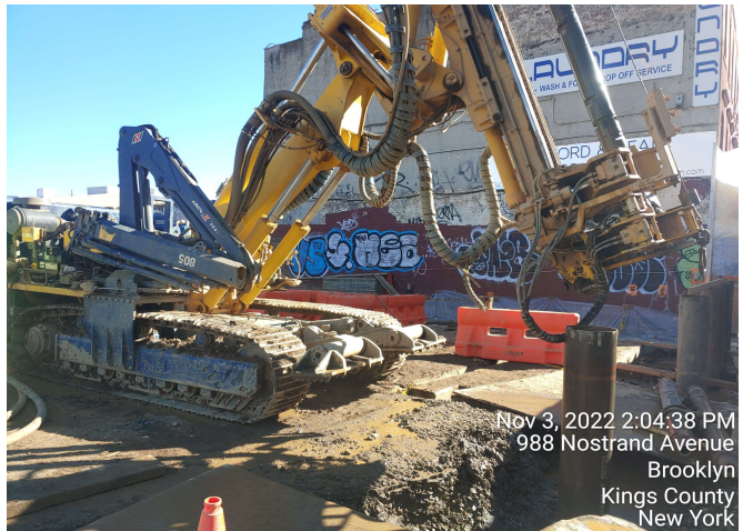
Photograph 2 - Installing soldier piles.
