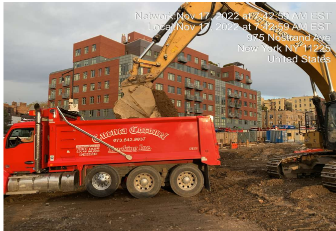
Photograph 1 - Loading of stockpiled material for disposal at BSM facility, facing northwest.
