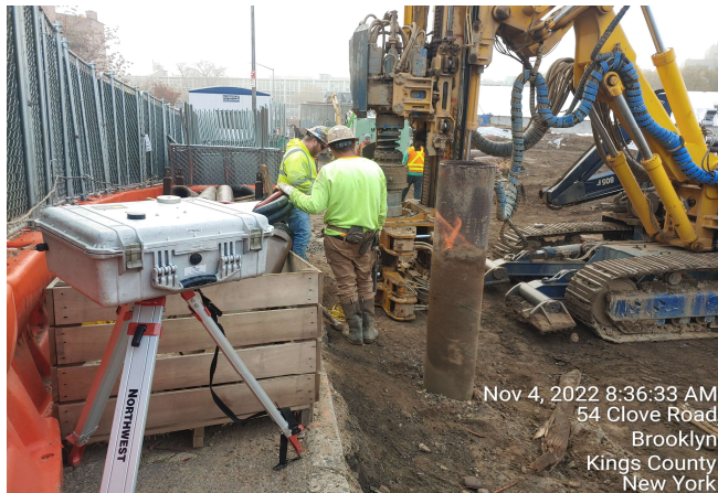
Photograph 2 - Installing soldier piles. Upwind CAMP station (foreground).
