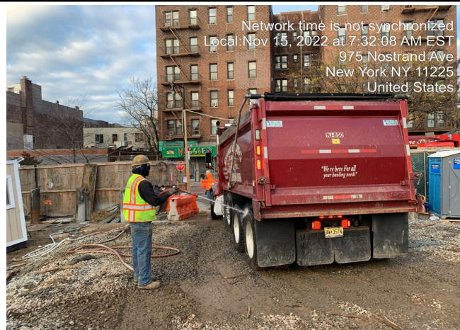
Photograph 2 - Truck tires being washed prior to departure, facing west.
