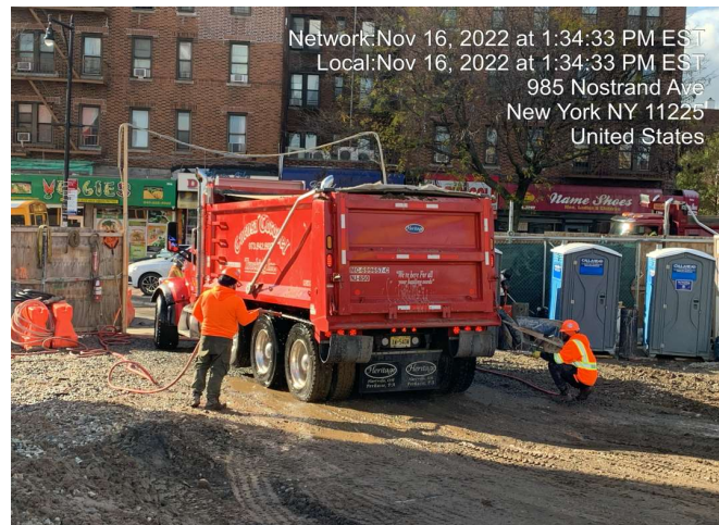
Photograph 2 - Truck tires being washed prior to departure, facing west.
