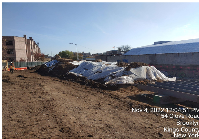
Photograph 3 - Soil stockpiles covered with poly sheeting.
