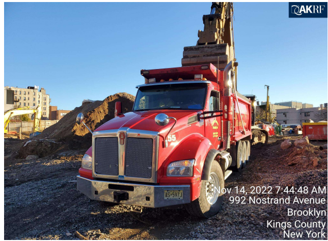
Photograph 1 - Loading of stockpiled material for disposal at BSM facility, facing east.
