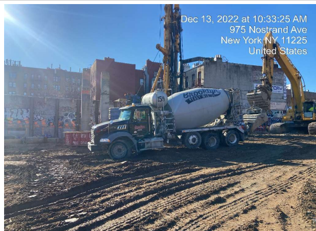
Photograph 3 - Grouting piles in Grid 12, facing southwest.
