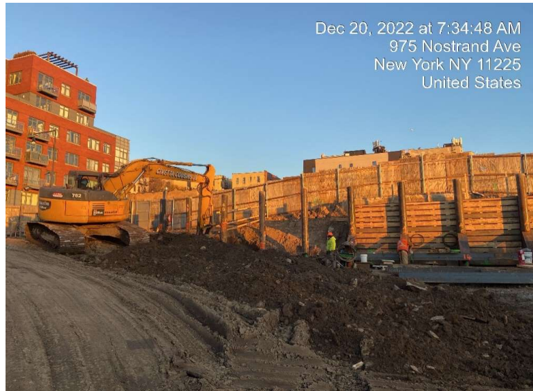
Photograph 2 - Installing SOE in Grid 1 (WC-2), facing north.
