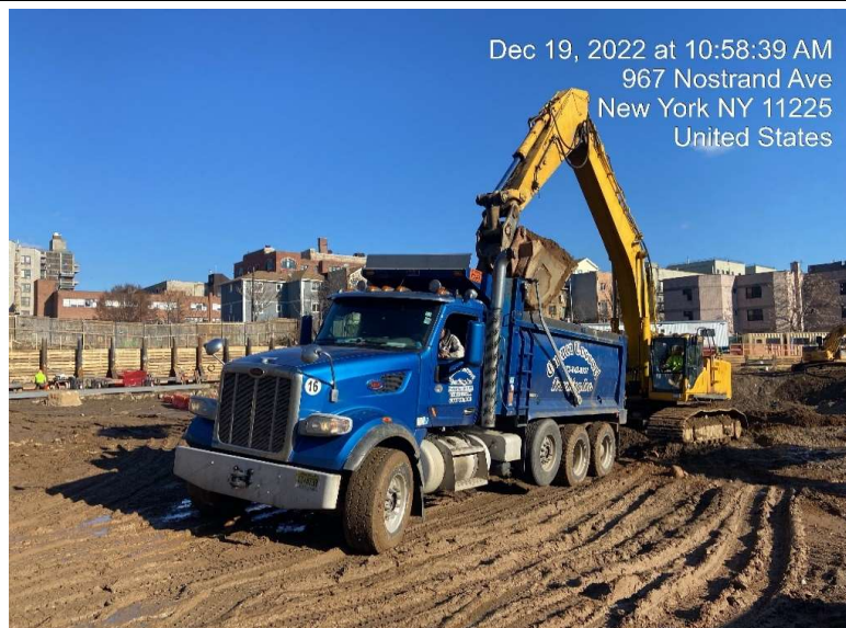
Photograph 1 - Loading soil onto trucks for export and disposal at the Bayshore Soil Management facility. View facing northeast.
