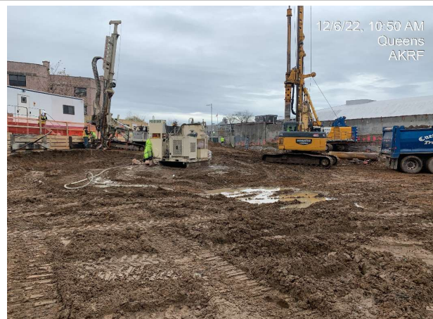
Photograph 3 - Grouting pile in Grid 15, facing southeast.
