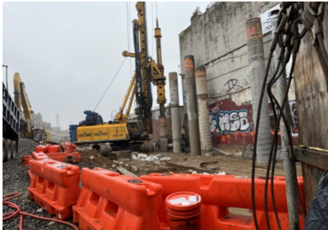
Photograph 2 - Drilling piles into waste grid WC-7 (facing southeast).
