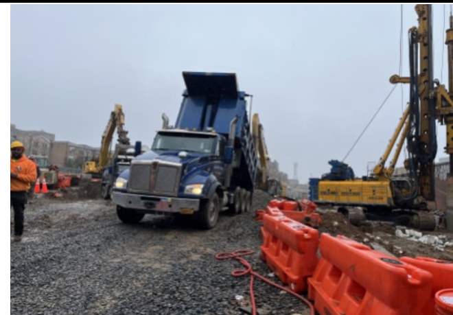
Photograph 3 - Import of stone from IRRC for truck pad (facing east).
