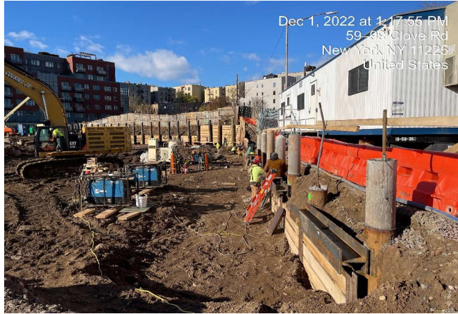
Photograph 1 - Installing lagging for SOE in Grid 6 (WC-5), facing north.
