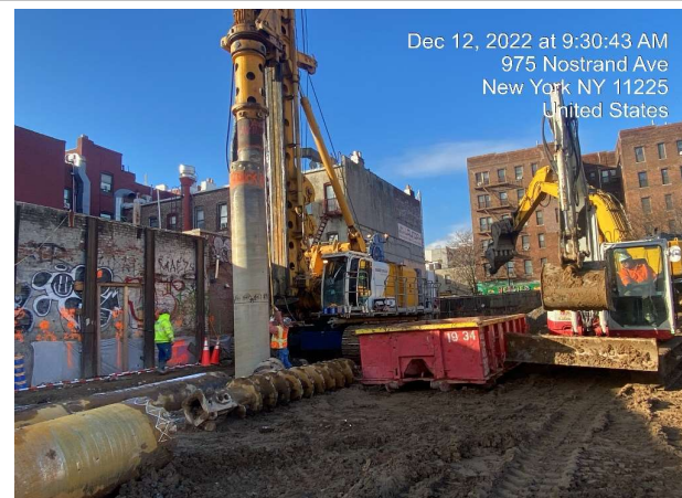
Photograph 3 - Grouting piles in Grid 12, facing southwest.
