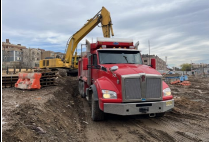
Photograph 1 - Loading soil onto trucks for export at the Impact Reuse and Recovery Center in Lyndhurst, NJ (facing east).
