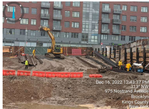
Photograph 2 - Installing SOE in Grid 2 (WC-3), facing northwest.
