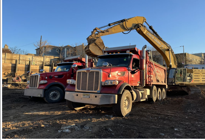
Photograph 1 - Loading soil onto trucks for export at the Impact Reuse and Recovery Center in Lyndhurst, NJ (facing northeast).
