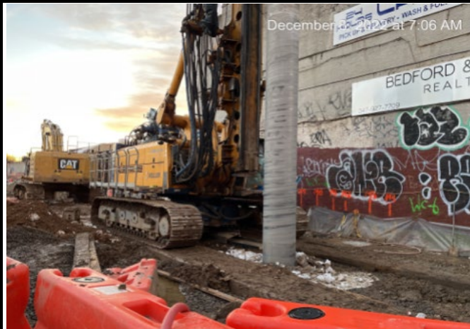
Photograph 2 - Drilling piles into waste grid WC-6 (facing southeast).
