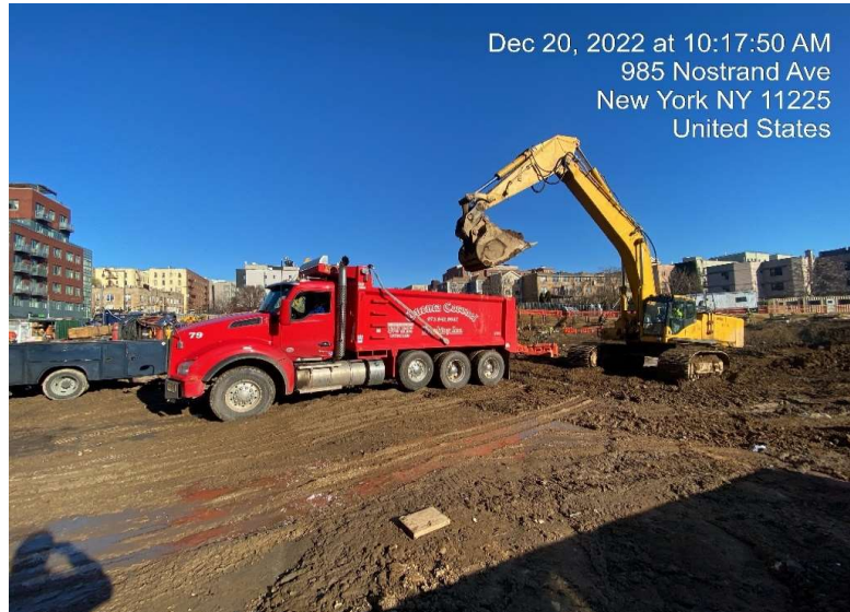
Photograph 1 - Loading soil onto trucks for export and disposal at the Bayshore Soil Management facility. View facing northeast.
