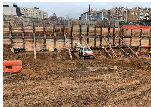
Photograph 3 - Excavation to install lagging for SOE, view facing north.
