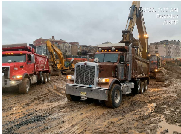
Photograph 3 - Loading trucks with soil/fill from Grids 2, 4, and 5 (waste class grid WC-2/3) and from Grids 13, 14 and 15 (WC-9/10/11) for off-site export.
