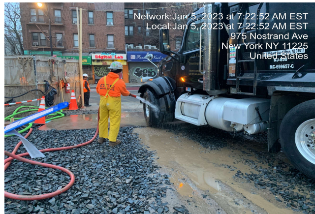
Photograph 2 - Washing truck tires at the Site entrance/exit.
