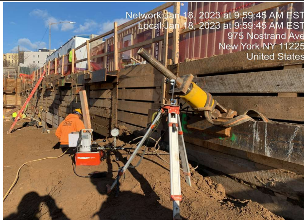
Photograph 2 - Civetta performing testing on a tieback, view facing north.
