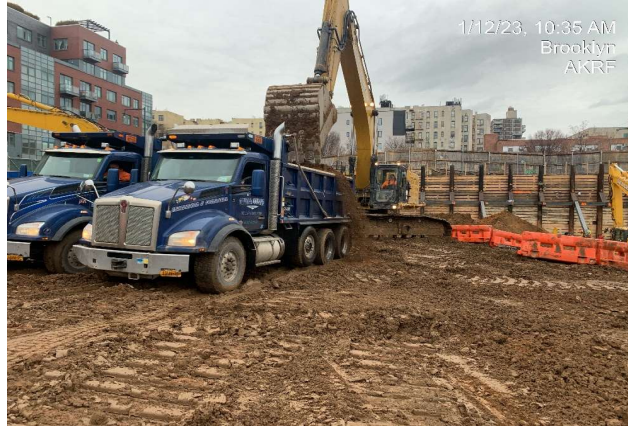
Photograph 1 - Loading truck with soil/fill for export to IRRC facility, view facing north.
