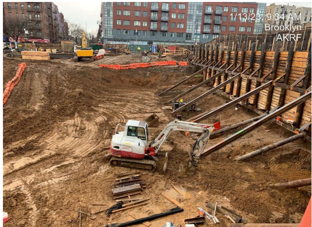
Photograph 2 - Grading around SOE, view facing west.
