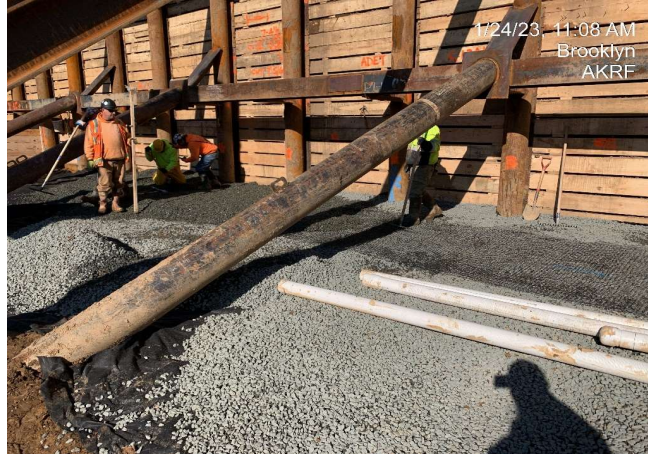
Photograph 1 - Contractor installing geogride above piping trench in grid 2.
