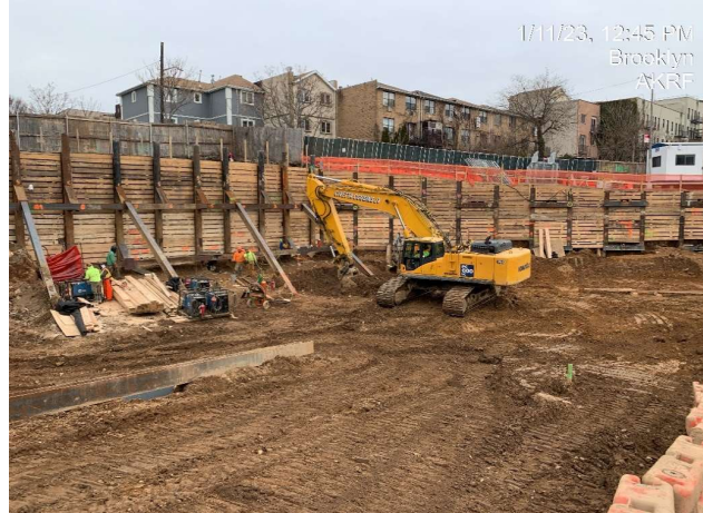
Photograph 2 - Grading associated with lagging and installation of heelblocks.
