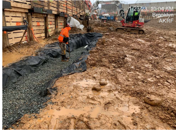
Photograph 1 - Contractor installing slotted SSDS pipe run (SSDS-11) for the SSDS in Grid 6.
