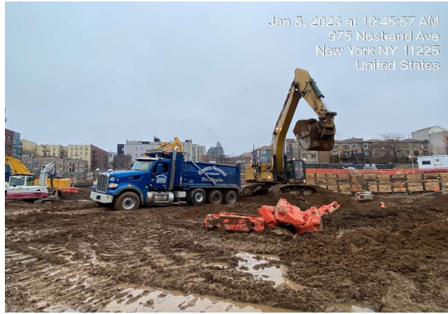
Photograph 1 - Loading soil onto trucks for export to IRRC in Lyndhurst, New Jersey, view facing northwest.
