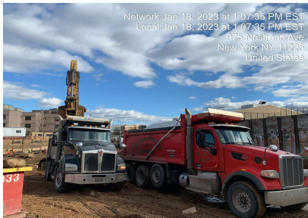
Photograph 3 - Loading soil into trucks from waste class Grids WC-8 and WC-9, view facing southeast.
