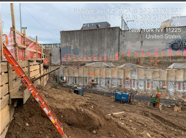
Photograph 3 - Welding for construction of rakers at the secant wall in the southeast corner, facing southeast.
