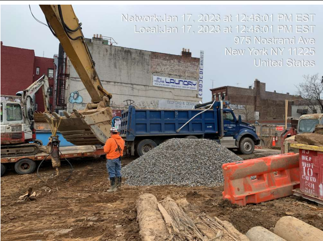
Photograph 2 - Delivery of 3/4" stone for refurbishment of the trucking pad at the southwestern gate, facing south.
