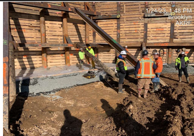
Photograph 3 - Contractor installing poly sheeting over GPA layer before pouring mud slab, Grid 2.
