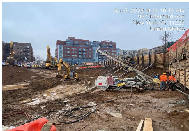
Photograph 3 - Drilling tiebacks in Grid 6 (WC-5), view facing northwest.
