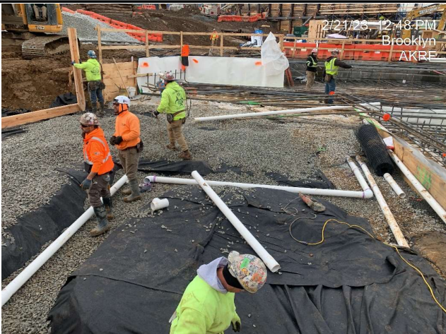
Photograph 3 - Installing components of the SSDS system in Grid 9, view facing west.
