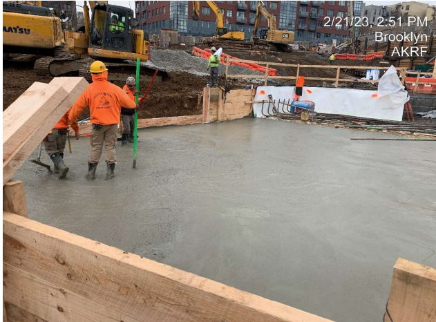
Photograph 2 - Pouring mud slab in Grid 9, view facing northwest.
