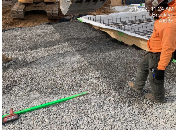
Photograph 1 - Installation of GPA and geogrid in Grid 10, view facing west.
