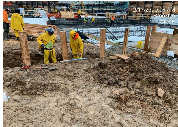
Photograph 2 - Installing concrete forms for mat slab grid 13. View facing northeast.
