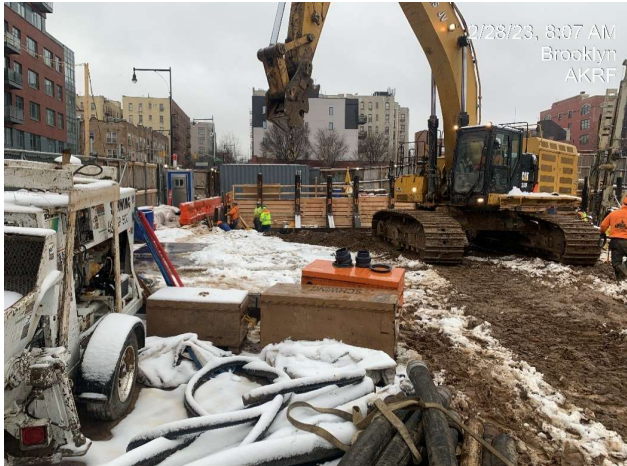
Photograph 2 - Installing SOE in Grid 1, view facing north.
