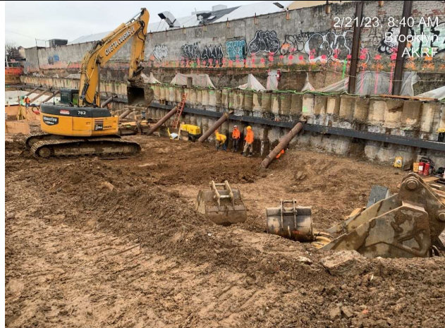
Photograph 1 - Excavation and grading associated with SOE in grids 12 and 13, view facing southeast.
