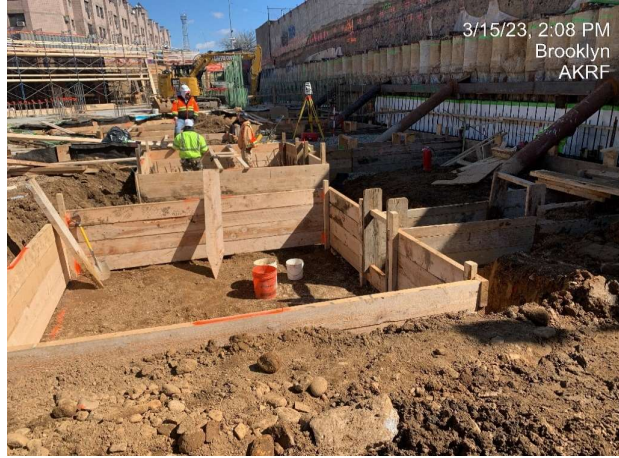
Photograph 1 - Installing forms for footings, view facing west.
