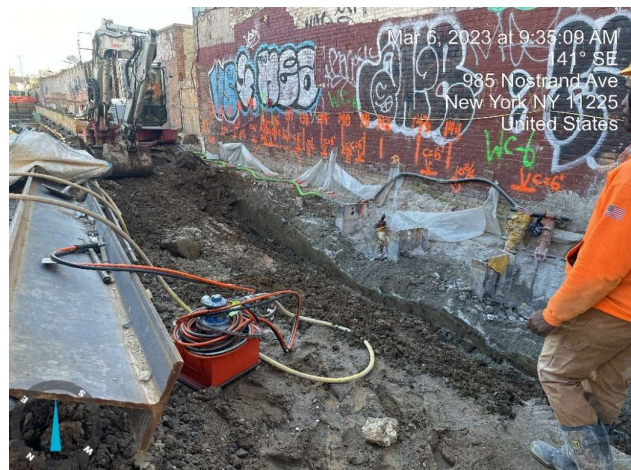
Photograph 3 - Excavation in Grid 11 (waste class WC-7), view facing east.
