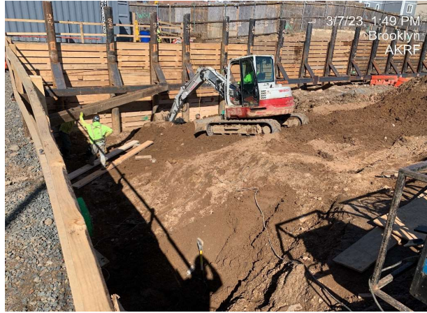
Photograph 1 - Installing SOE and associated excavation.
