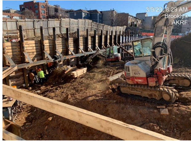
Photograph 1 - Installing SOE and associated excavation.
