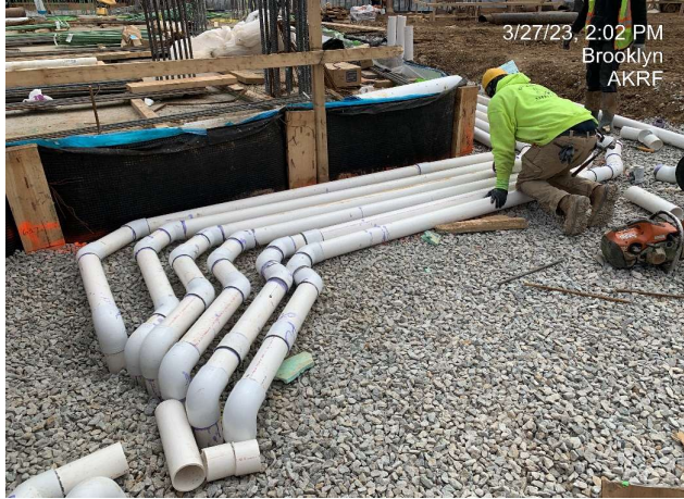
Photograph 2 - Installing SSDS components in Grid 9, view facing south.
