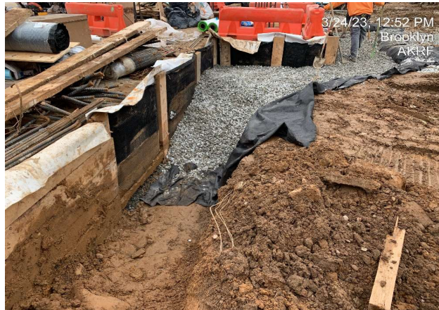
Photograph 2 - Installing SSDS components in Grid 9, view facing south.
