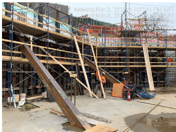
Photograph 3 - Rebar and formwork installation in Grids 2 and 6, view facing east.
