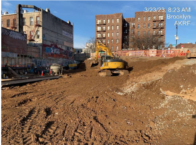
Photograph 3 - Excavation and grading continues, view facing west.
