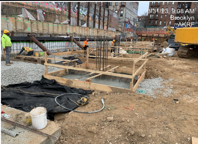
Photograph 3 - Pouring concrete for footings, view facing southwest.
