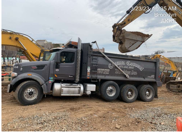
Photograph 1 - Exporting soil/fill to the Bayshore Soil Management facility, view facing northeast.
