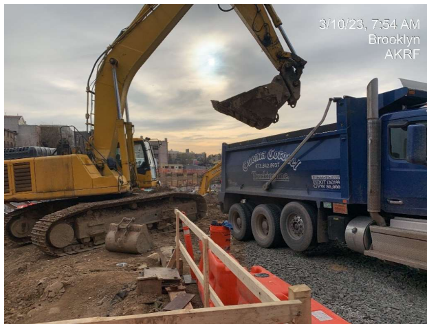
Photograph 3 - Exporting soil/fill to IRRC facility, view facing north.
