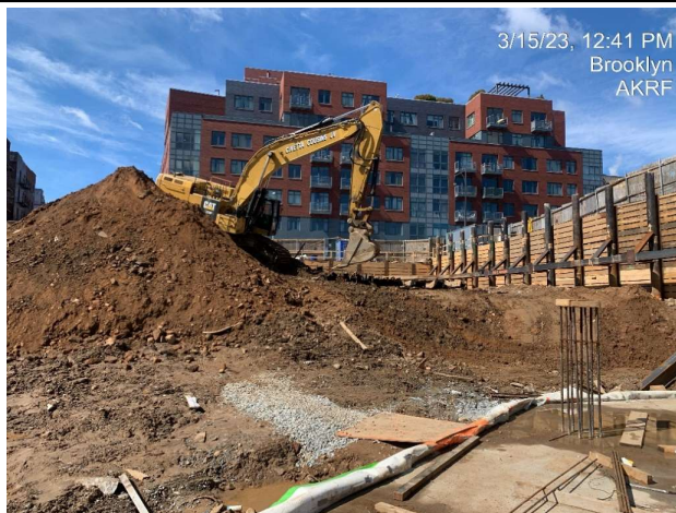
Photograph 3 - Excavating and stockpiling soil/fill for future off-site export, view facing southeast.
