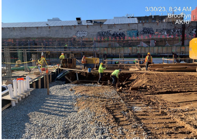
Photograph 3 - Excavation for foundation elements, view facing south.
