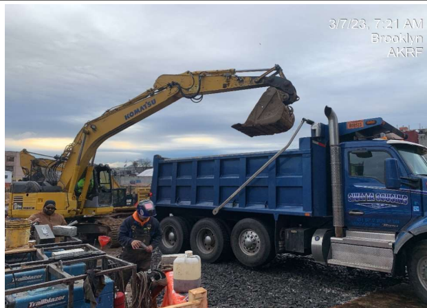
Photograph 3 - Loading excavated soil on to trucks for off-site export and disposal.
