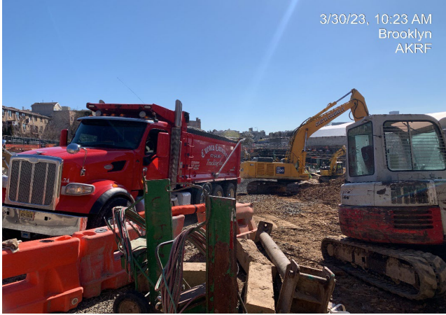
Photograph 2 - Exporting soil/fill to Bayshore facility, view facing southeast.
