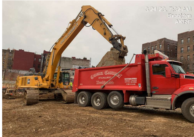
Photograph 1 - Exporting soil/fill to the Bayshore Soil Management facility, view facing southwest.
