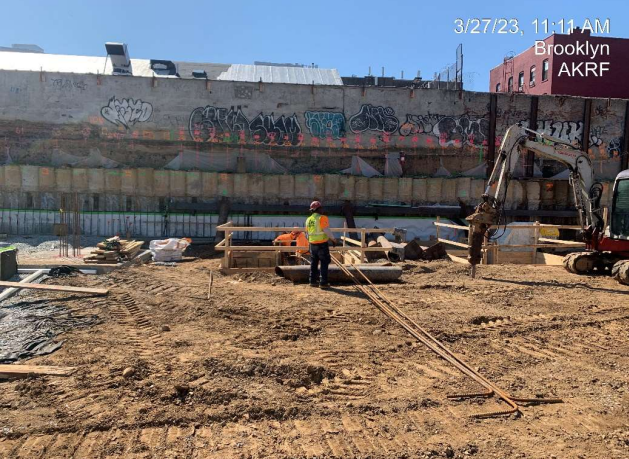
Photograph 3 - Installing rebar for footings, view facing west.
