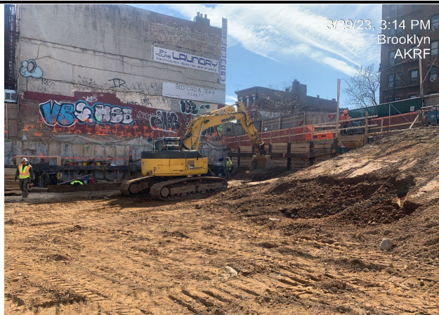
Photograph 3 - Installing lagging and welding for SOE, view facing southwest.
