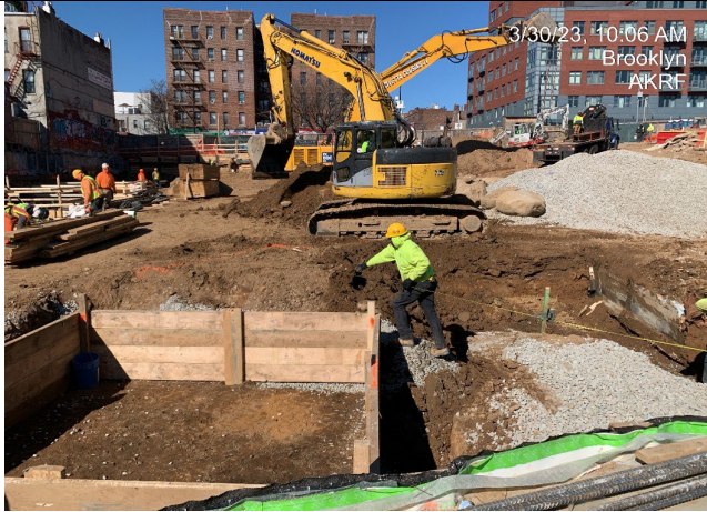
Photograph 1 - Installing concrete forms for foundation elements, view facing west.
