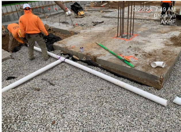
Photograph 2 - Installation of SSDS piping in Grid 14, view facing southwest.
