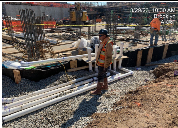
Photograph 2 - Installing SSDS components in Grid 9, view facing southeast.
