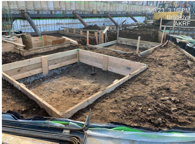
Photograph 2 - Installation of concrete forms for footings, view facing south.
