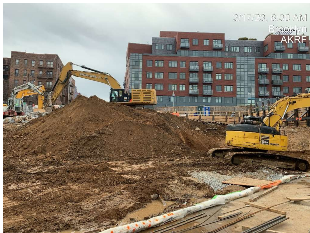
Photograph 3 - Excavating and stockpiling soil/fill, view facing west.
