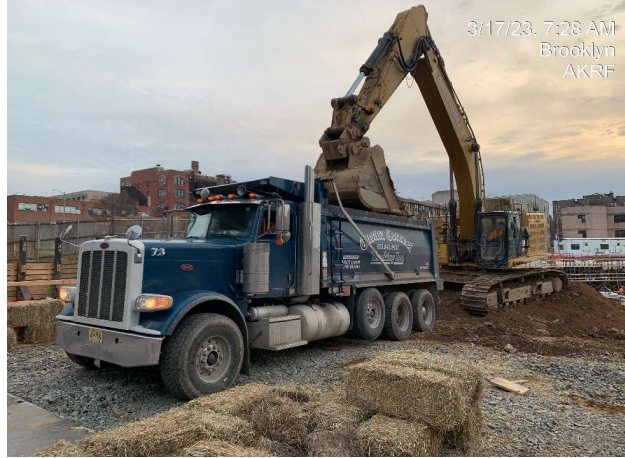
Photograph 1 - Exporting soil/fill to IRRC facility, view facing northeast.
