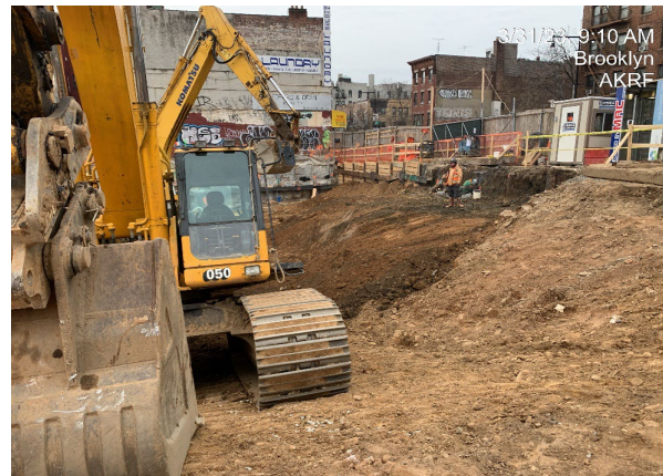
Photograph 2 - Welding of rakers and excavation associated with SOE, view facing south.
