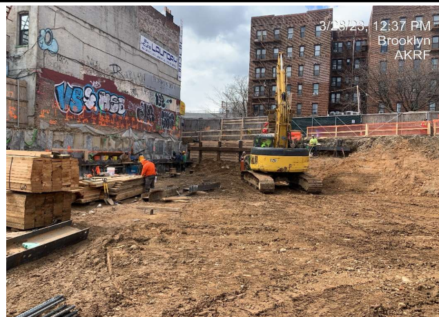
Photograph 3 - Installing lagging and welding for SOE, view facing west.
