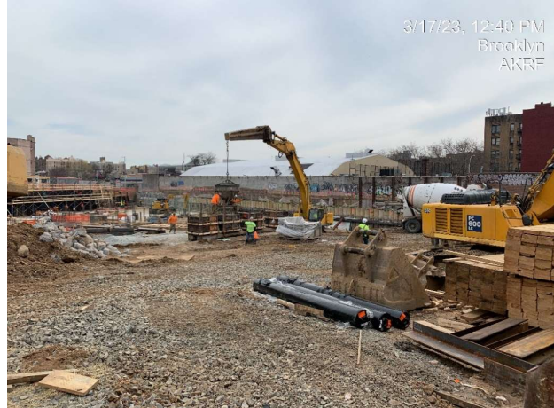
Photograph 2 - Pouring concrete for heelblocks, view facing southeast.
