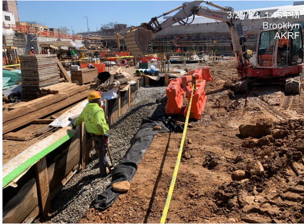
Photograph 1 - Installing SSDS components in grid 5, view facing south.
