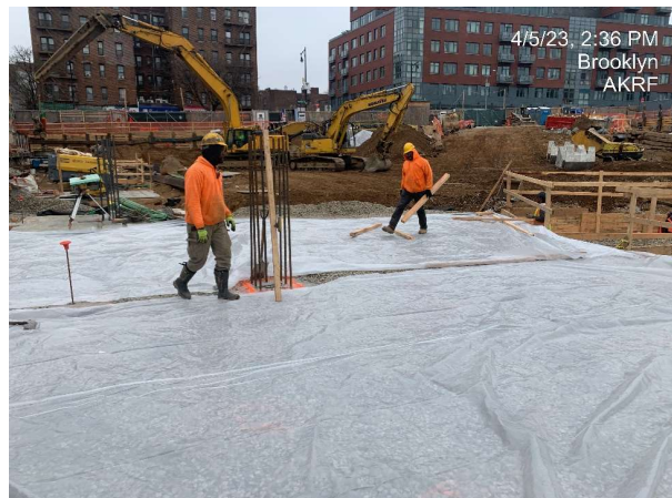
Photograph 2 - Laying poly sheeting over the SSDS GPA layer prior to pouring the mud slab, view facing northwest.
