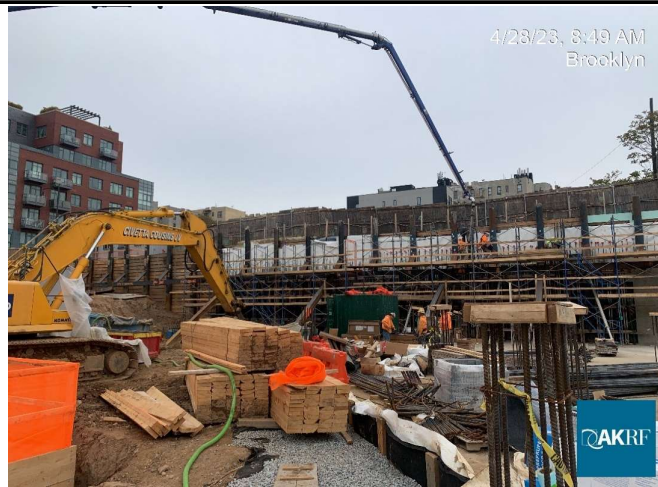
Photograph 1 - Pouring concrete for northern wall, view facing northwest.
