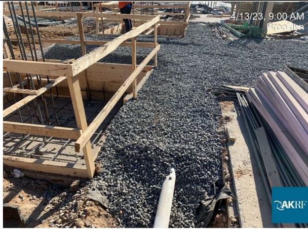
Photograph 1 - Installed subgrade SSDS piping in Grid 9.
