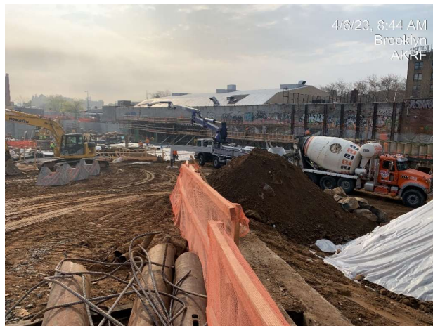
Photograph 3 - Pouring concrete for the southern wall, view facing southwest.
