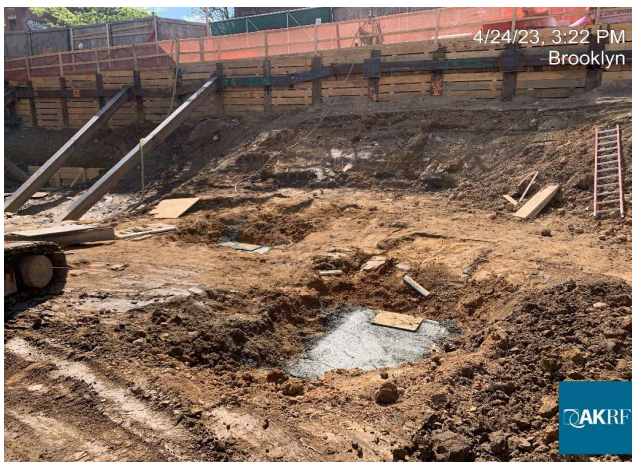
Photograph 3 - Excavated area and poured concrete for the heelblocks, view facing southeast.
