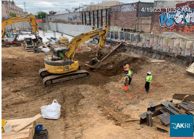
Photograph 2 - Installing heelblocks and rakers for SOE, view facing southeast.
