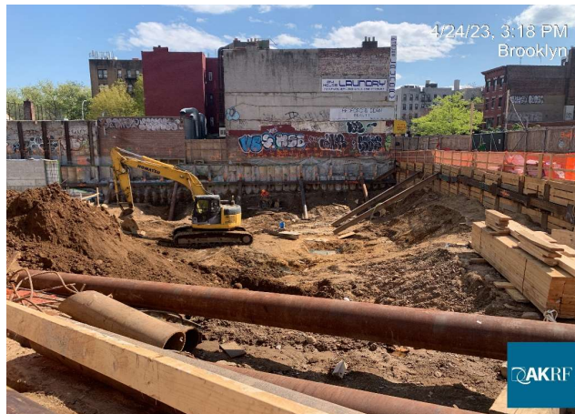
Photograph 2 - Excavation for heelblocks, view facing south.
