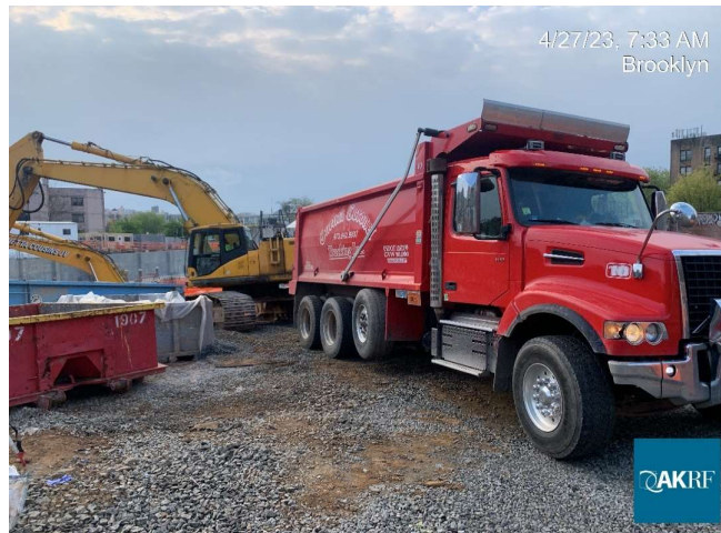
Photograph 1 - Loading soil on to trucks for disposal, view facing south.
