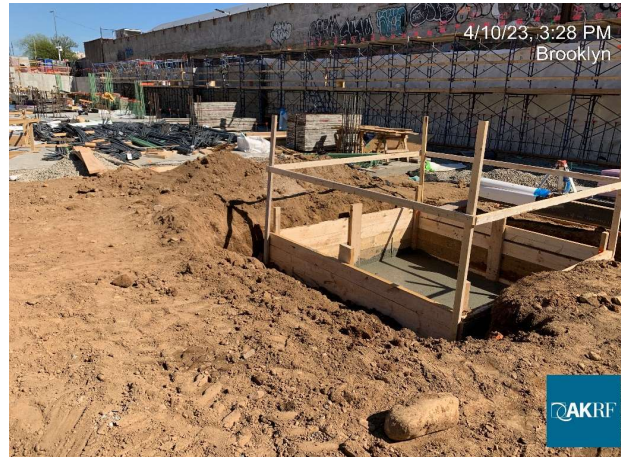
Photograph 1 - Installed foundation footings, view facing southeast.
