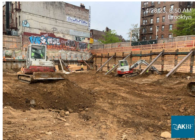
Photograph 2 - Installation of SOE, view facing southwest.
