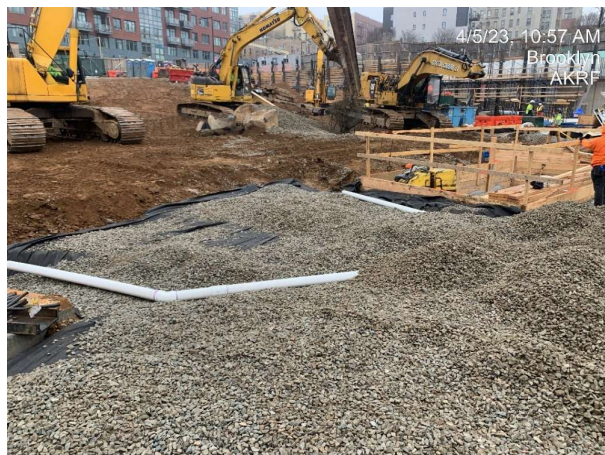
Photograph 3 - Installing portions fo the SSDS system, view facing northwest.
