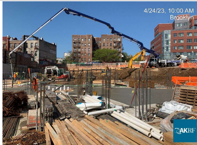
Photograph 1 - Pouring concrete for the foundation slab, view facing west.
