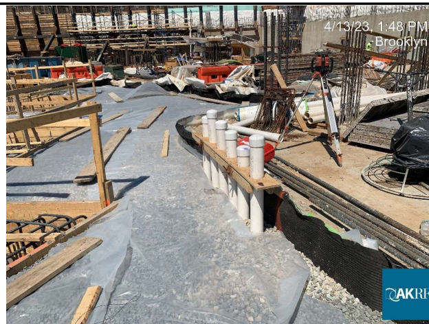
Photograph 3 - Preparation for installation of concrete mud slab in Grid 9, view facing northeast.
