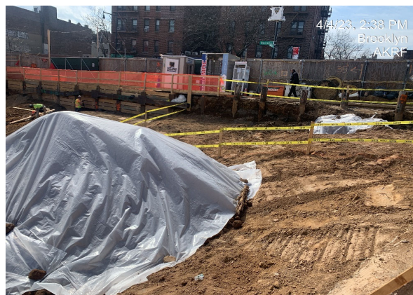
Photograph 3 - Covered petroleum contaminated stockpile and covered USTs, view facing west.
