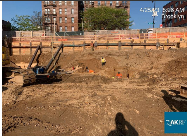
Photograph 1 - Installation of SOE, view facing west.
