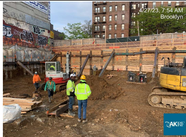
Photograph 2 - Installation of SOE, view facing west.
