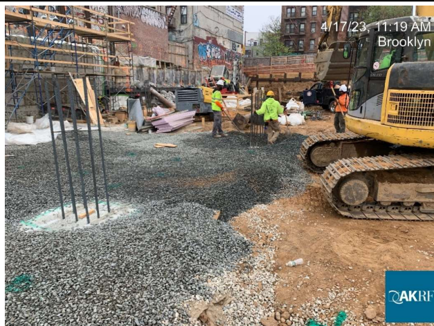
Photograph 3 - Installing GPA layer of SSDS system, view facing west.
