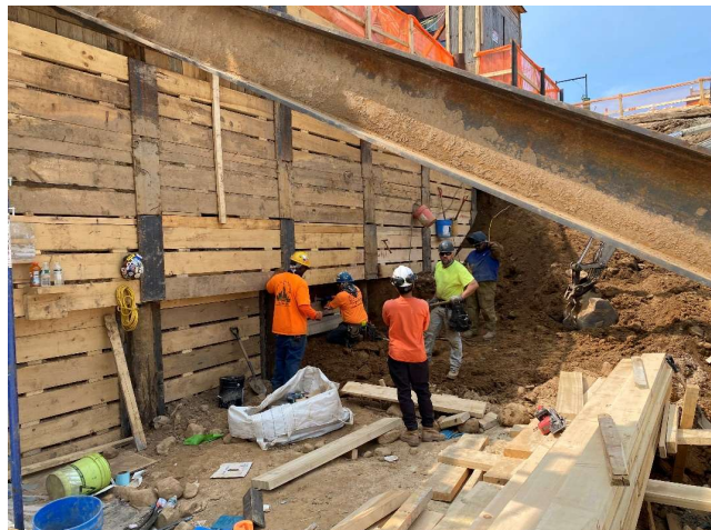
Photograph 2 - Installation of SOE, view facing northeast.
