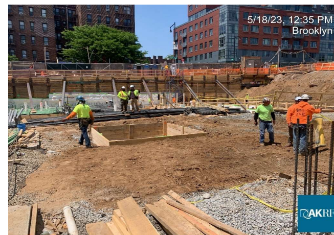
Photograph 3 - Installed foundation footing Grid 12, view facing west.
