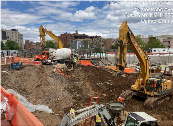
Photograph 1 - Pouring concrete for heel blocks as part of the SOE, view facing northeast.
