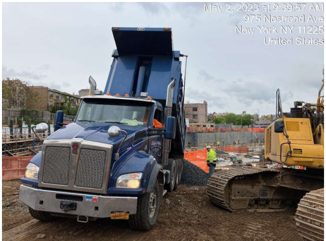
Photograph 3 - Unloading GPA stone, view facing southeast.
