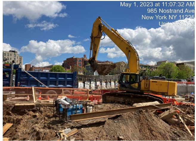
Photograph 2 - Loading soil on to trucks for disposal, view facing northeast.
