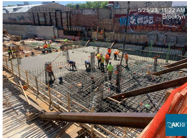
Photograph 2 - Pouring concrete for the slab, view facing west.
