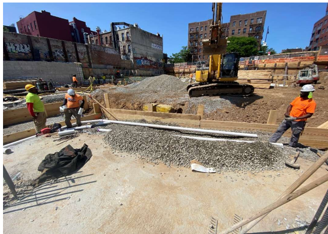
Photograph 3 - Installed SSDS piping in Grid 8, view facing southwest.
