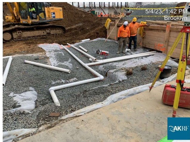
Photograph 3 - Installation of SSDS piping, view facing northeast.
