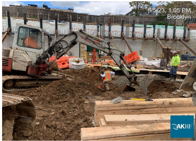
Photograph 1 - Excavation for foundation footings, view facing north.
