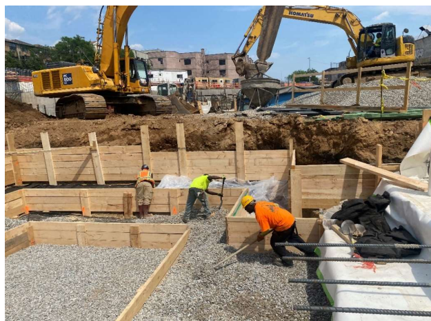
Photograph 3 - Installation of stepped mat slab area, view facing east.
