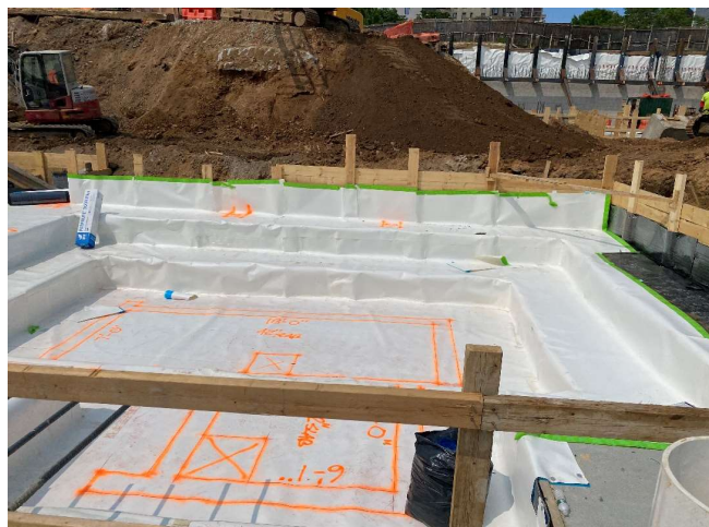
Photograph 3 - Installed vapor barrier/waterproofing at the stepped mat slab area, view facing east.
