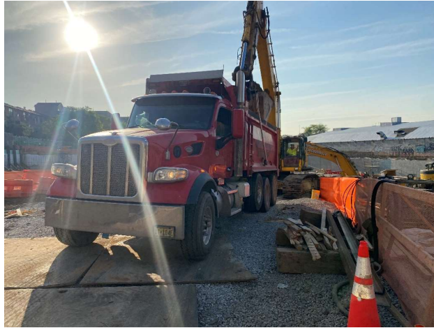
Photograph 1 - Loading soil on to trucks for off-site disposal, view facing southwest.
