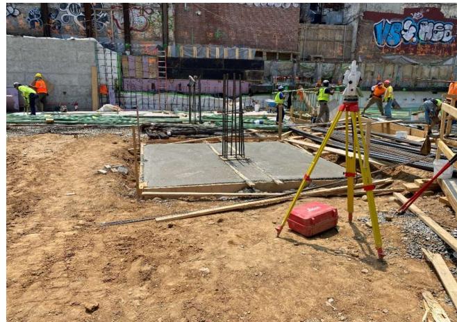
Photograph 2 - Concrete poured for footing installation in Grid 8
