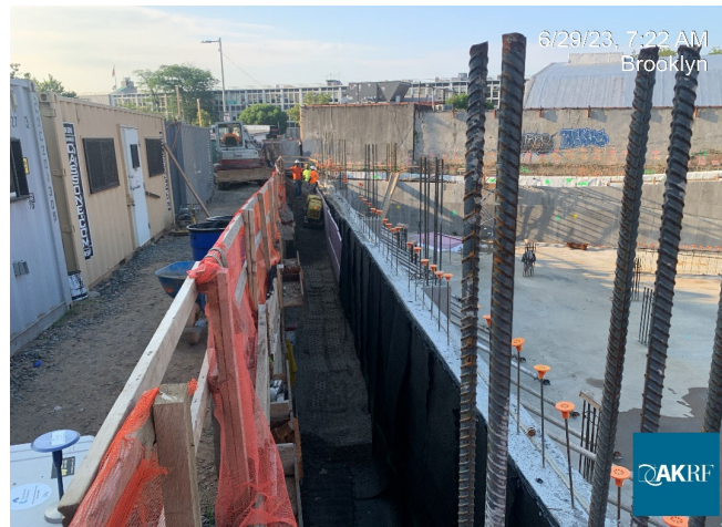
Photograph 1 - Backfill behind SE wall Grid 15, view facing south.
