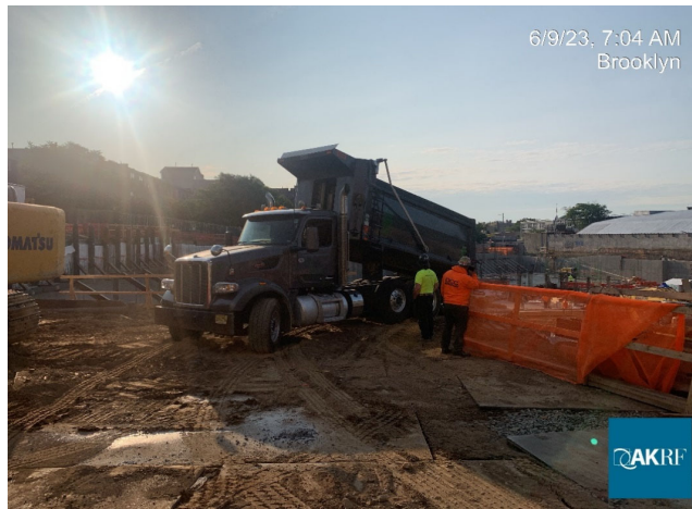
Photograph 1 - Unloading GPA stone in Grid 3, view facing east.
