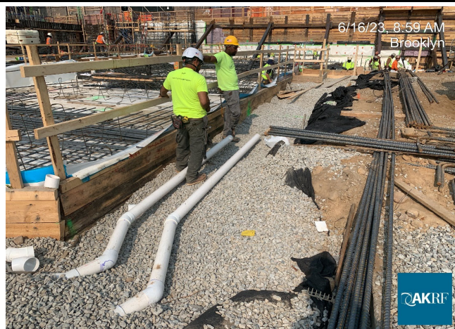
Photograph 3 - Installation of SSDS components, view facing west.
