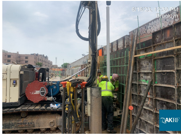
Photograph 1 - Eastern Environmental drilling well for SVE system, view facing east.
