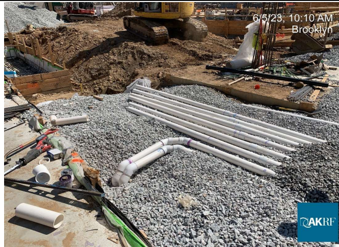
Photograph 1 - Installation of SSDS Grid 12.
