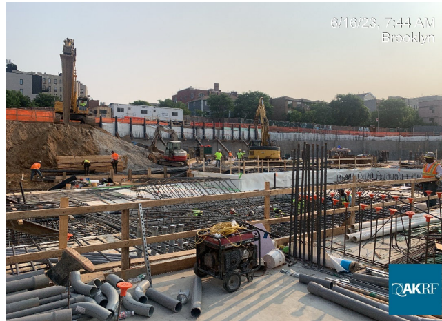
Photograph 2 - Rebar installation in Grids 8 and 9, view facing northeast.
