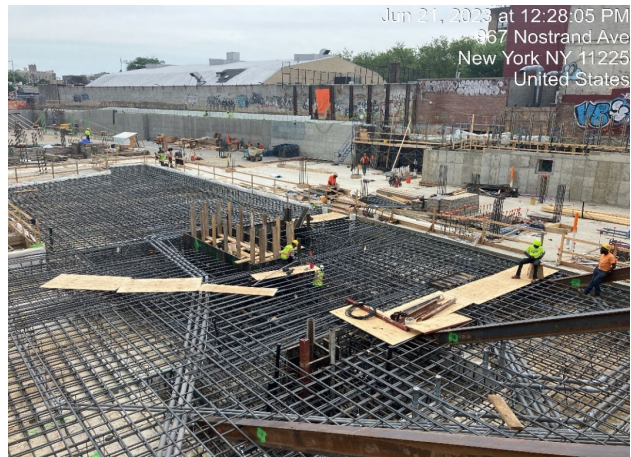
Photograph 2 - Installing rebar in Grids 8 and 9, view facing southeast.
