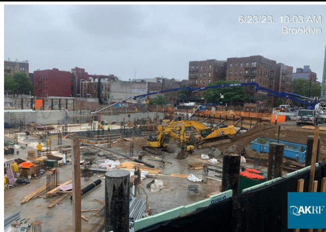
Photograph 3 - Pouring concrete for mat slab section in Grid 7, 8, and 9, view facing southeast.
