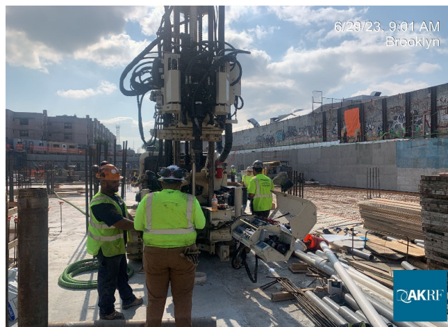
Photograph 3 - Eastern Environmental drilling SVE well , view facing southeast.
