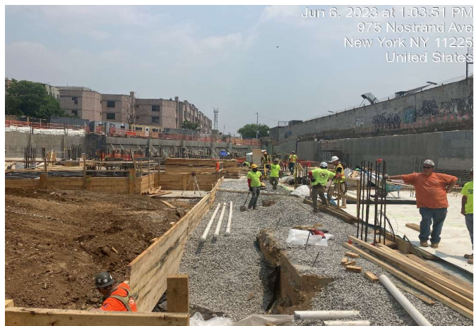
Photograph 1 - Installation of SSDS in Grid 8, view facing east.
