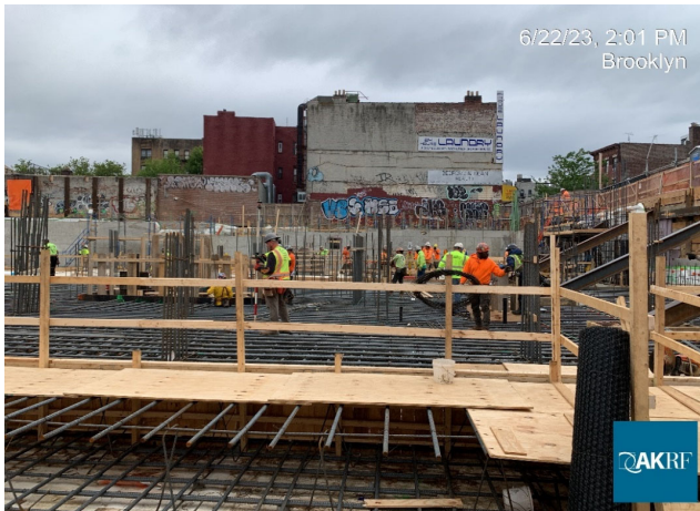
Photograph 2 - Installing rebar in Grids 7 and 8, view facing south.
