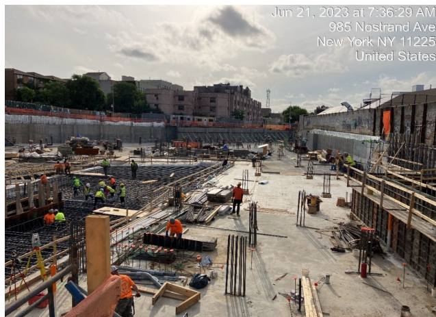
Photograph 3 - Installing rebar in Grids 8 and 9, view facing east.
