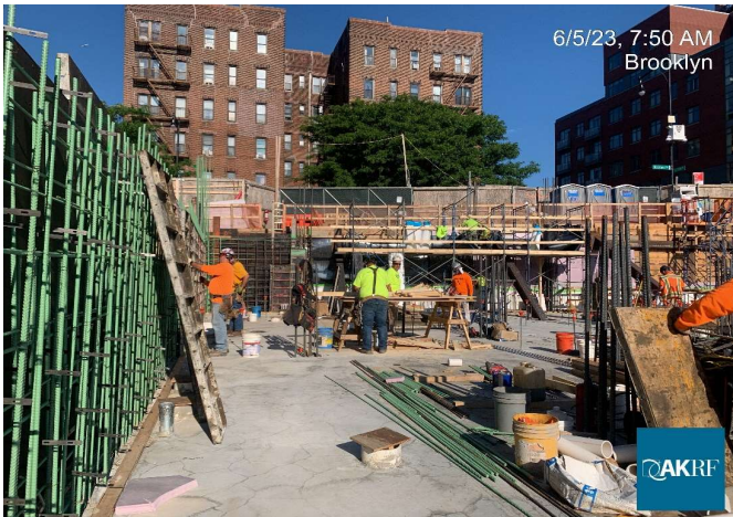
Photograph 3 - Installation of concrete forms Grid 11, view facing west.
