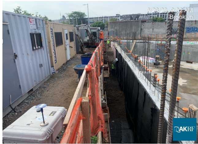
Photograph 1 - Backfilling behind SE wall in Grid 15, view facing south.
