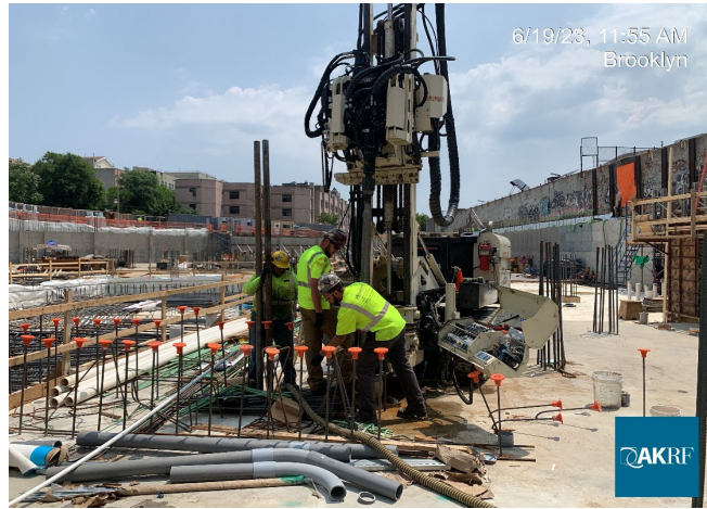
Photograph 1 - Eastern Environmental drilling monitoring point for SVE system.
