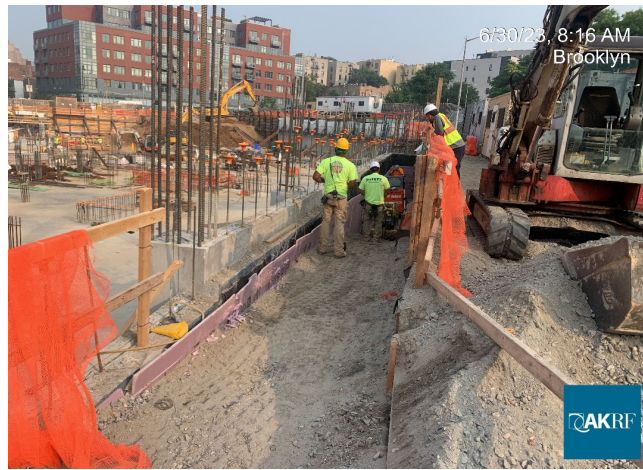
Photograph 1 - Backfilling behind SE wall Grid 15, view facing north.
