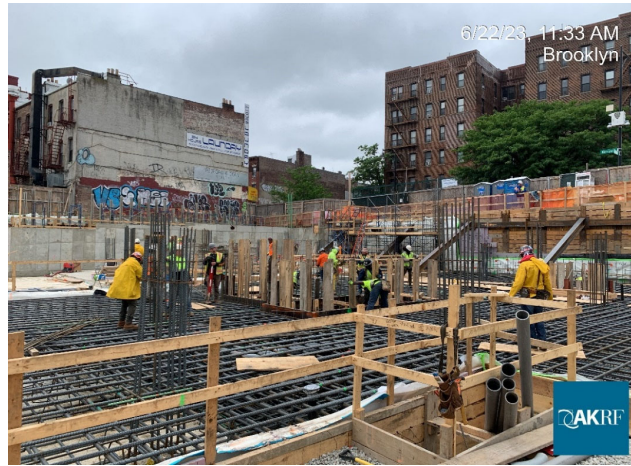
Photograph 1 - Installing rebar in Grids 7 and 8, view facing southeast.
