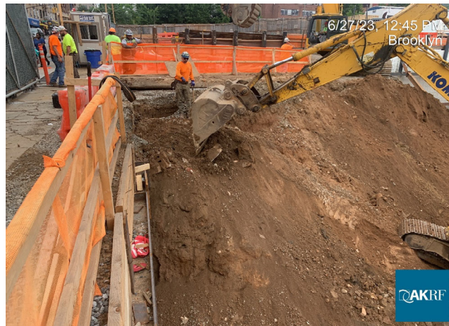
Photograph 2 - Excavation for SOE in Grid 3, view facing north.
