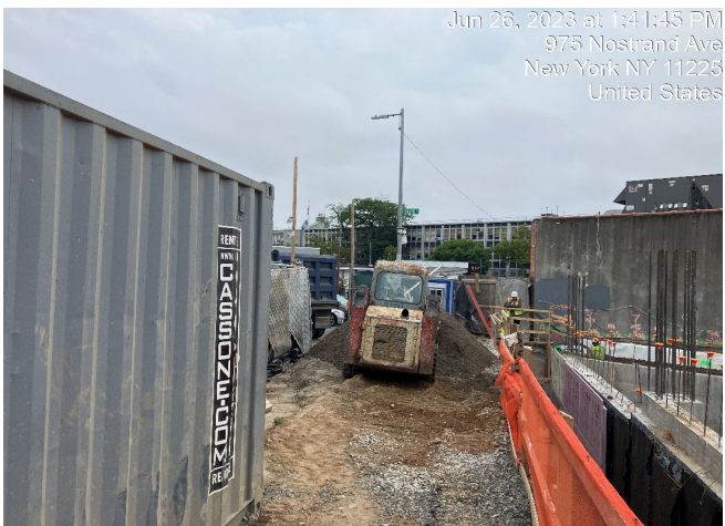
Photograph 3 - Using imported DGA for backfilling behind the foundation walls.
