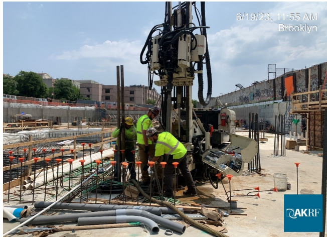
Photograph 1 - Eastern Environmental drilling monitoring point for SVE system.
