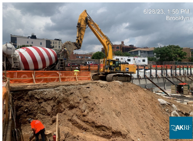
Photograph 3 - Pouring concrete for heelblocks Grid 3, view facing northwest.
