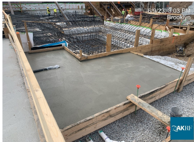
Photograph 2 - Concrete poured for the mud slab in Grid 12, view facing northwest.
