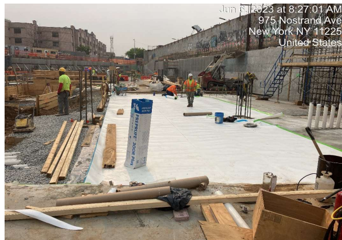
Photograph 2 - Installation of waterproofing in grid 12, view facing east.
