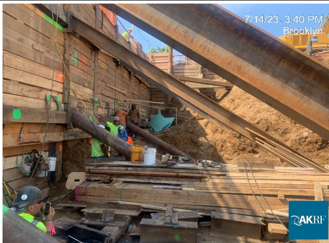
Photograph 3 - SOE installation, view facing north.
