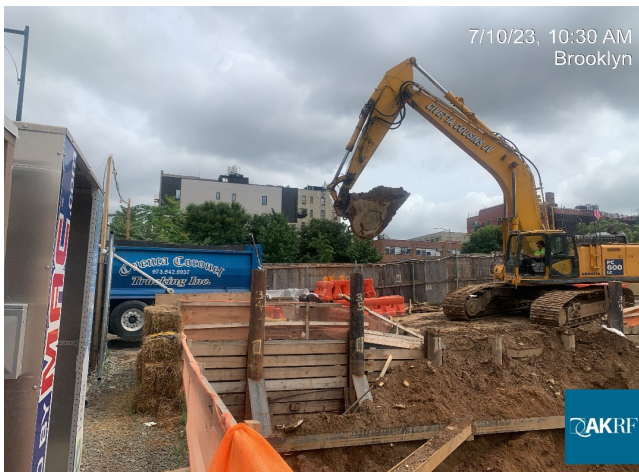
Photograph 3 - Loading soil/fill on to trucks for off-site disposal, view facing north.
