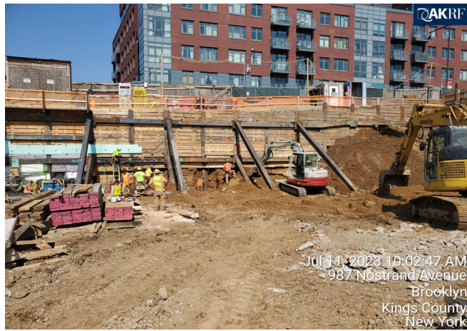
Photograph 1 - Installation of SOE in Grid 3, view facing west.
