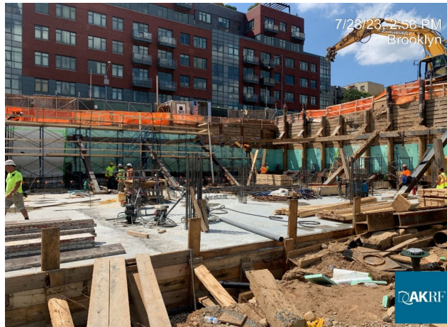
Photograph 2 - Installing insulation, view facing northwest.
