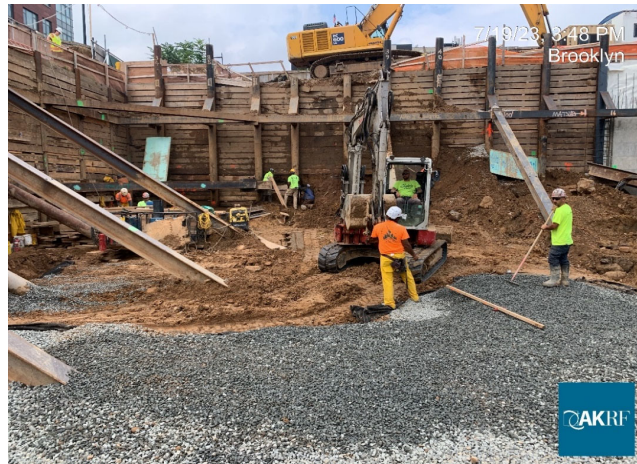
Photograph 2 - Installation of SOE Grid 1, view facing north.
