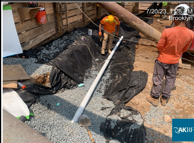
Photograph 3 - Installation of SSDS components in Grid 3, view facing north.
