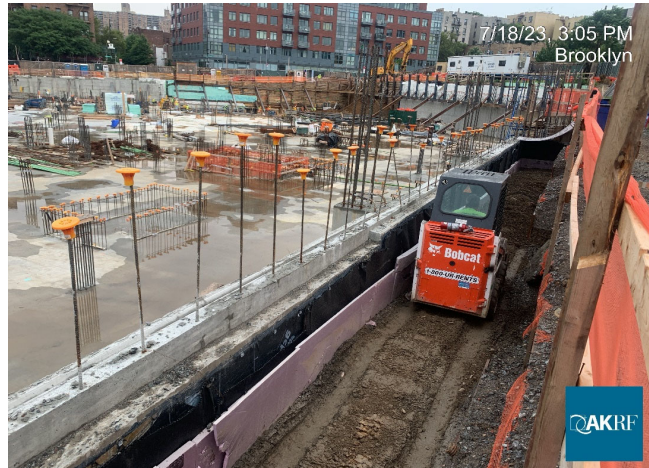
Photograph 2 - Backfilling behind foundation walls in Grid 15, view facing northwest.
