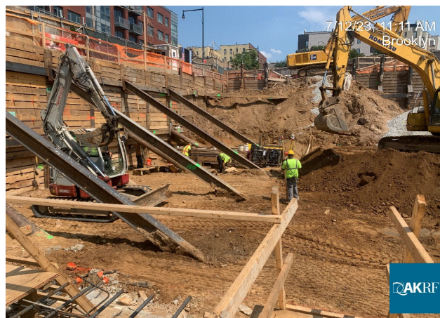
Photograph 3 - Grading and SOE installation, view facing Northwest.
