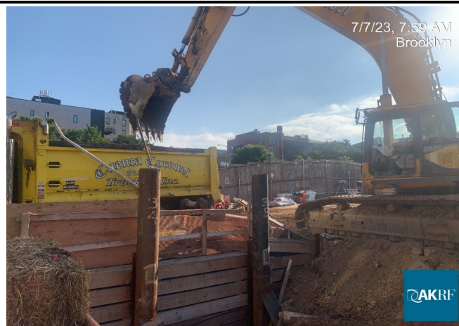
Photograph 3 - Loading soil/fill on to trucks for off-site disposal, view facing southeast.
