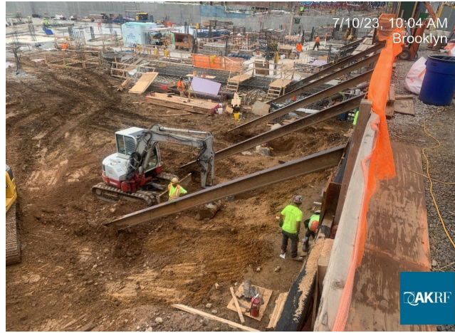
Photograph 1 - Installation of SOE in Grid 3, view facing southwest.
