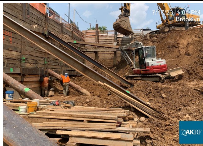
Photograph 3 - SOE installation, view facing north.
