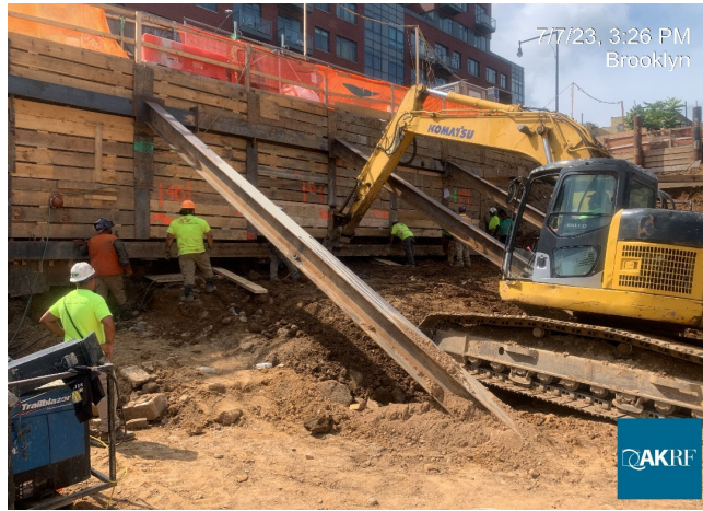
Photograph 1 - Installation of SOE in Grid 3, view facing northwest.
