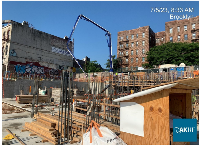
Photograph 1 - Pouring concrete for western foundation wall in Grid 11, view facing southwest.
