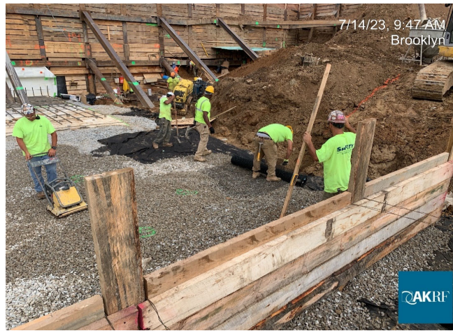
Photograph 1 - Installation of SSDS components, view facing northwest.
