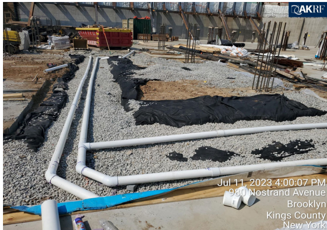
Photograph 2 - Installation of SSDS pipes, view facing north.
