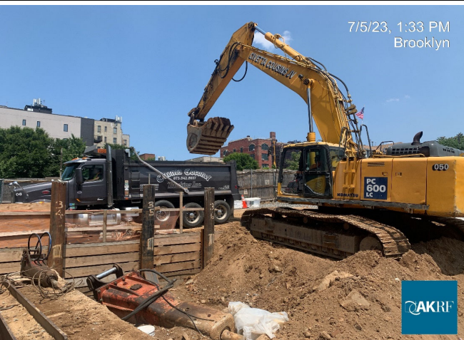
Photograph 3 - Loading soil/fill on to trucks for off-site disposal, view facing northeast.
