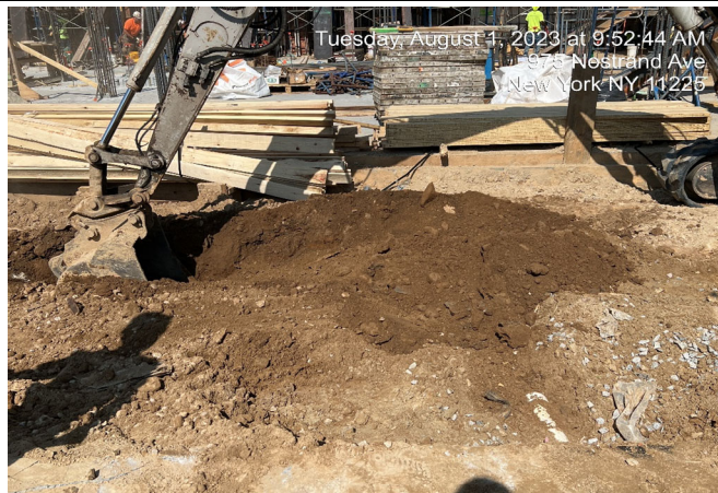
Photograph 2 - Excavation for SSDS trench in Grid 4, view facing west.
