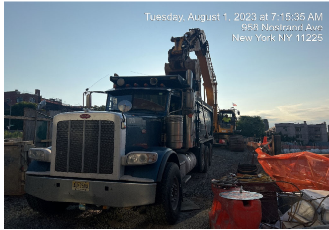
Photograph 1 - Loading soil onto trucks for export, view facing east.
