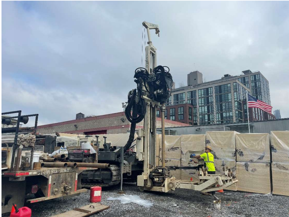
Photo 1: View of AARCO advancing soil boring SB15 (facing north).
