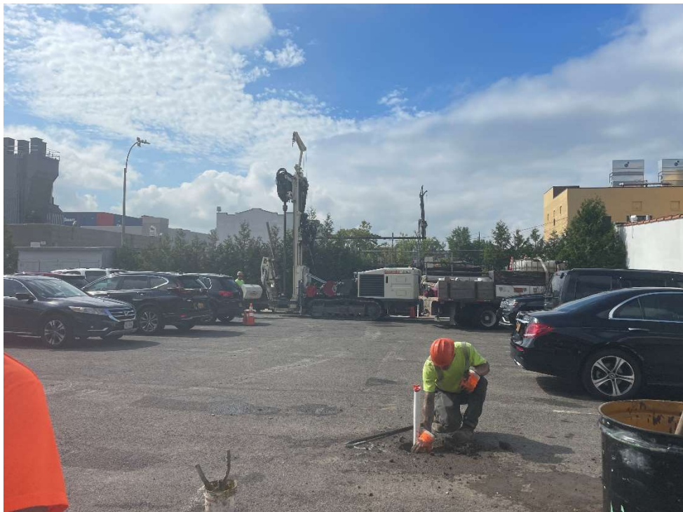
Photo 2: AARCO installing monitoring well MW14 (facing west).
