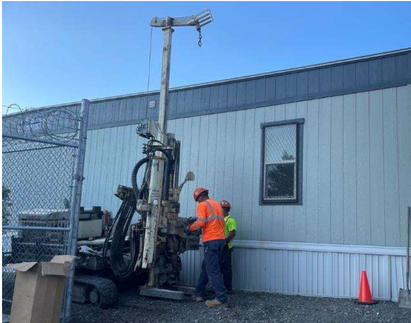
Photo 1: AARCO advancing soil boring SB05 (facing south).
