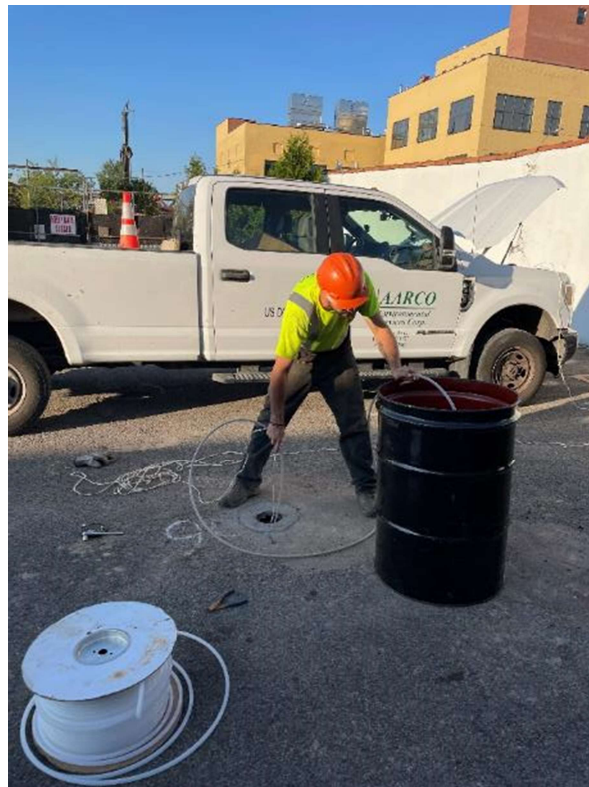
Photo 2: AARCO developing monitoring well MW06 (facing northwest).
