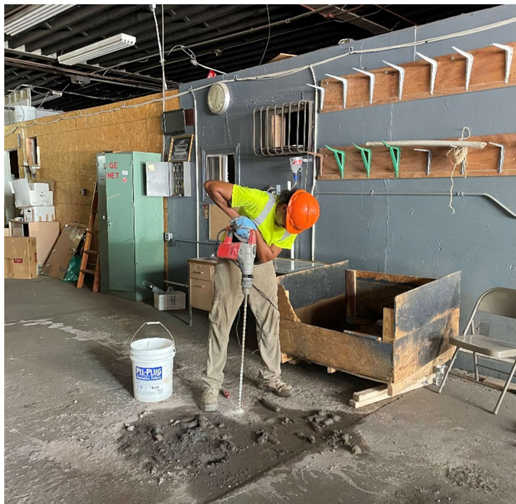
Photo 2: AARCO installing sub-slab vapor point SSV19 (facing west).
