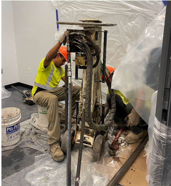
Photo 1: AARCO advancing soil boring SB08 (facing north).
