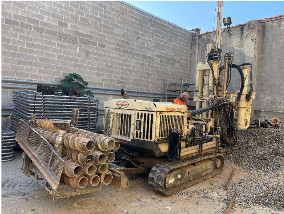
Photo 1: AARCO advancing soil boring SB18 (facing south).
