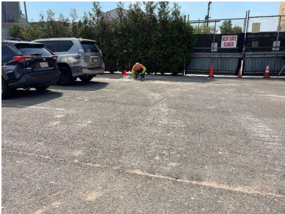
Photo 2: AARCO installing soil vapor point SV07 (facing south).
