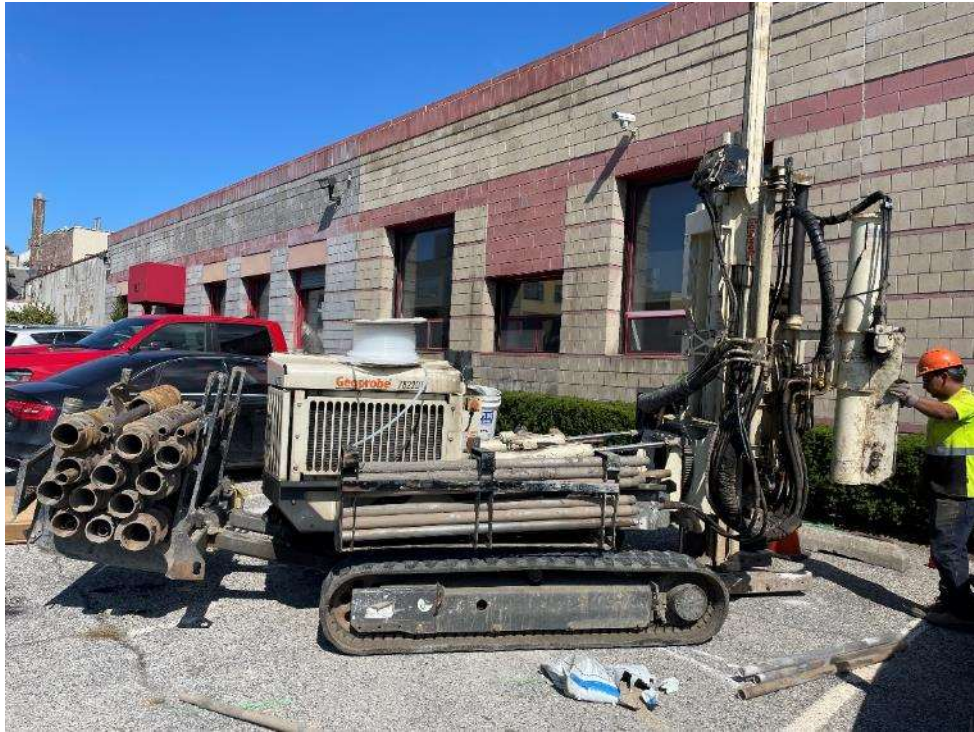
Photo 1: AARCO advancing step off of soil boring SB14 (facing north).
