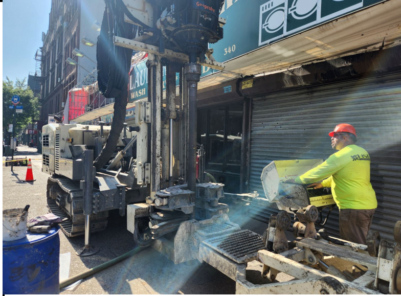
Photo 1: View of the drill rig setup at SB-19/MW-5.
