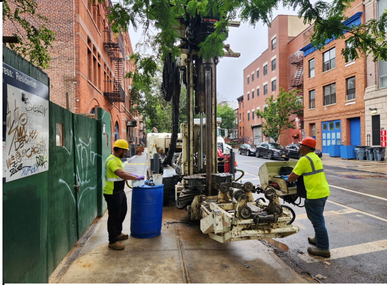
Photo 1: View of the drill rig setup at SB-18/MW-4.
