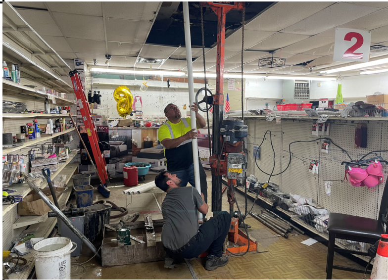
Photo 2: View of the installation of monitoring well MW-31.
