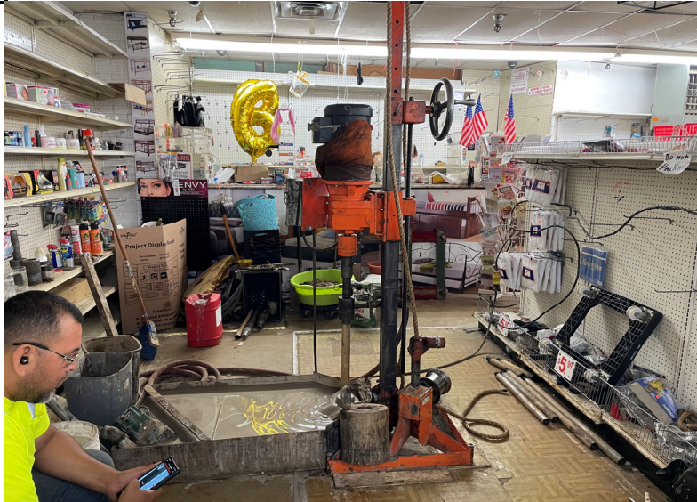
Photo 2: View of the drill rig setup at MW-3S.
