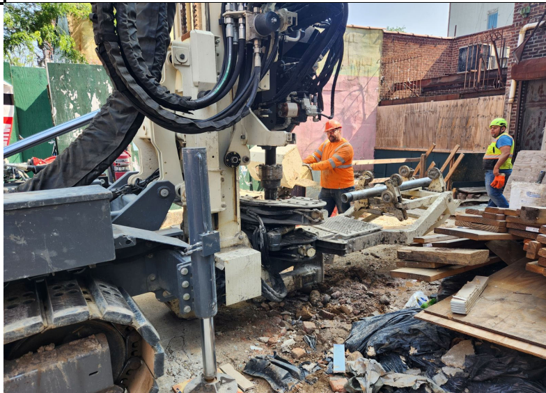
Photo 2: View of the MW-1 installation setup.
