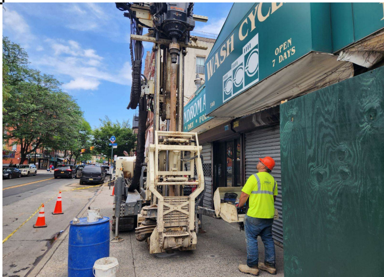
Photo 2: View of drill rig setup at SB-19/MW-5.
