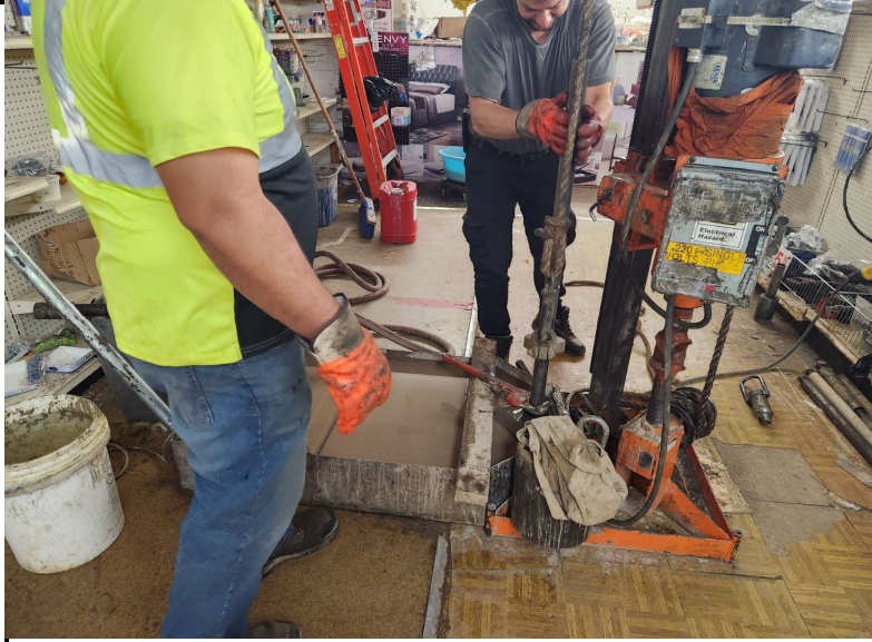
Photo 1: View of the drill rig setup at location SB-17.
