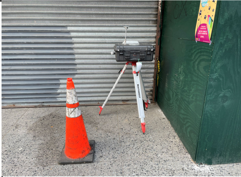
Photo 1: View of the downwind CAMP station setup.
