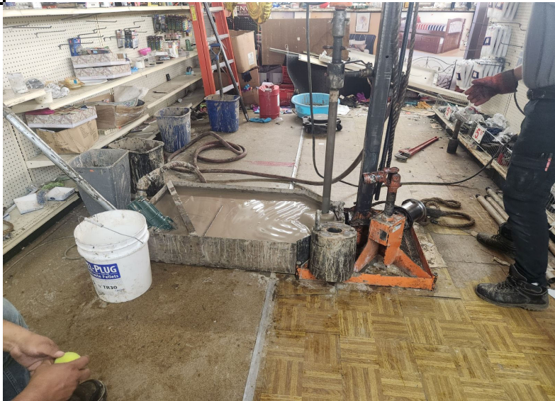
Photo 2: View of the drill rig setup at location SB-17.
