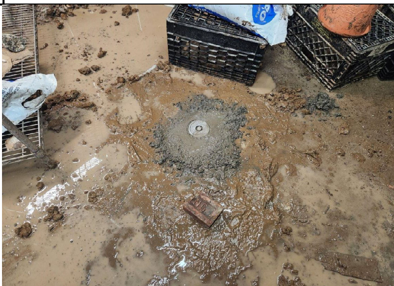
Photo 2: View of MW-3S following installation.
