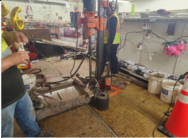
Photo 1: View of the drill rig setup at SB-17.
