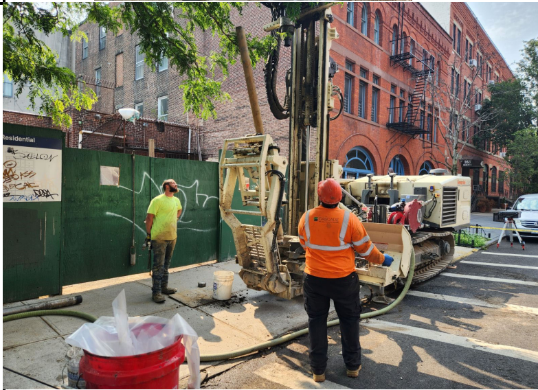
Photo 2: Setting up to install soil boring SB-18.
