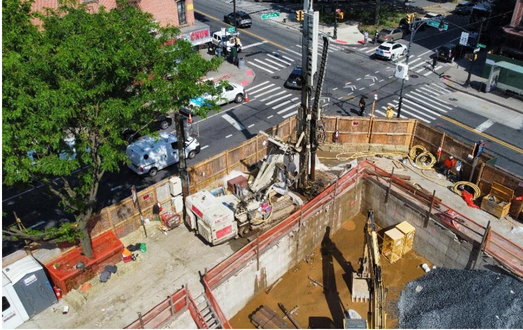
Photo 1: View of soldier pile installation, facing northwest.
