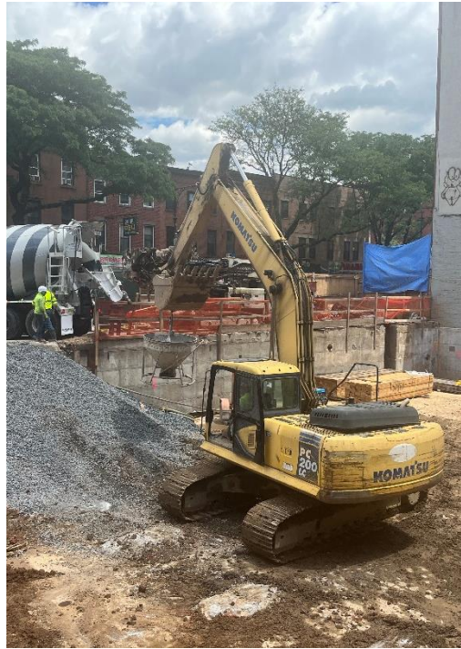
Photo 1: View of contractor delivering concrete for SOE installation, facing northwest.
