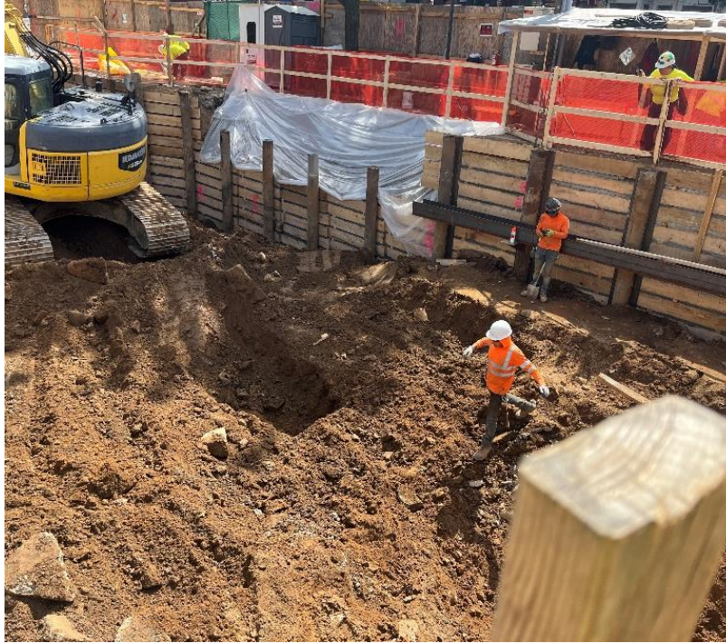
Photo 3: View of the contractor excavating for heel block, facing southwest.
