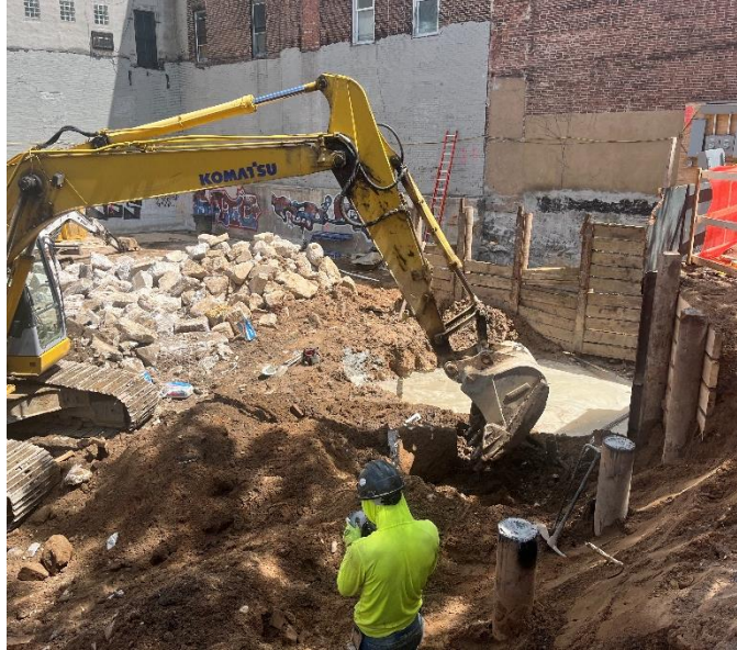
Photo 3: View of the contractor excavating for lagging activities, facing southeast.
