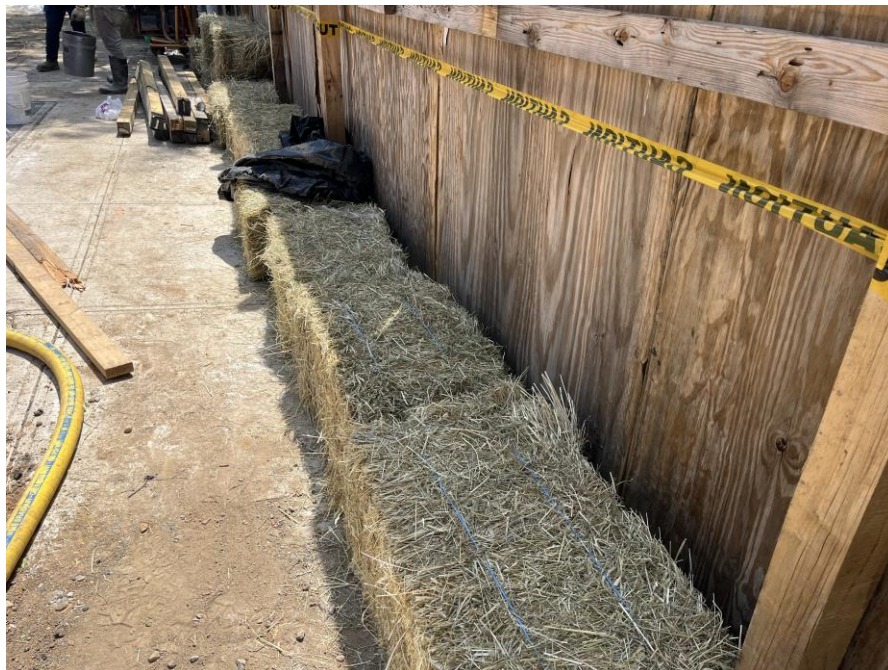
Photo 2: View of hay bales installed for erosion and sediment control along perimeter of the Site, facing south.
