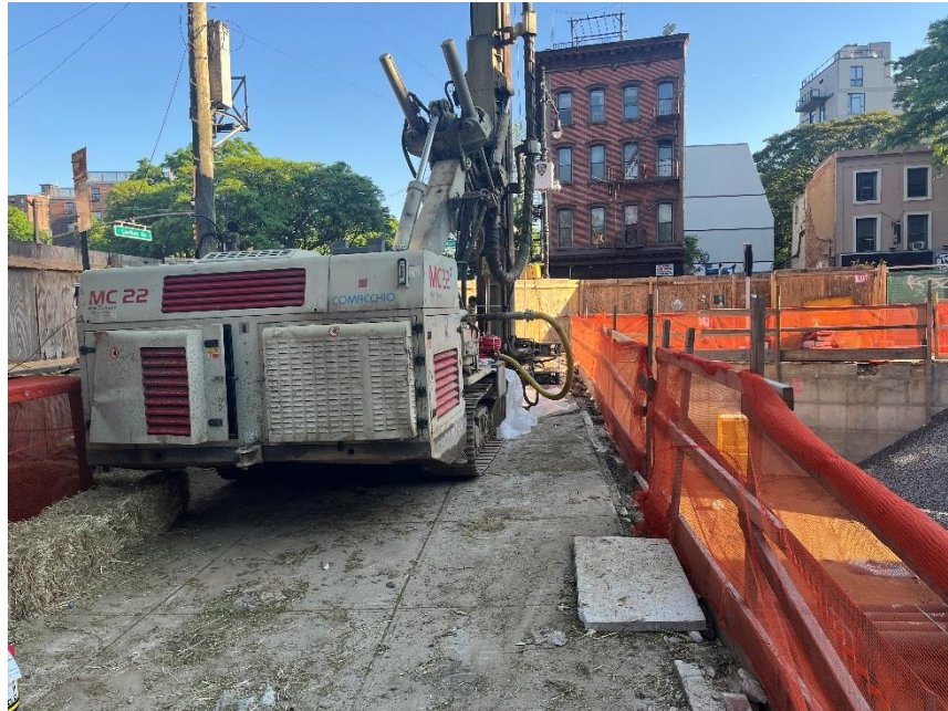
Photo 1: View of installation of soldier piles, facing north.
