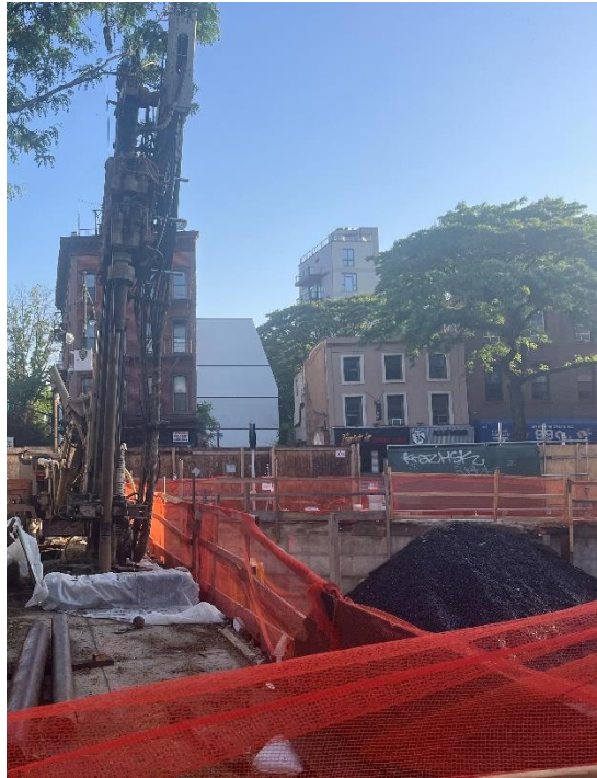
Photo 1: View of contractor installing soldier piles on the western portion of site, facing north.
