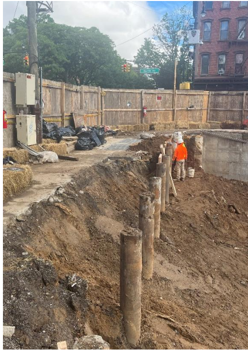
Photo 1: View of SOE, lagging activities along the western portion of site, facing north.
