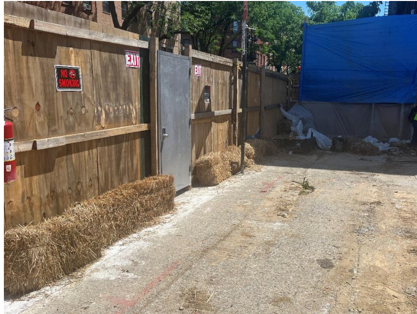
Photo 1: View of Site conditions and hay bales installed for erosion and sediment control along perimeter of the Site, facing northeast.
