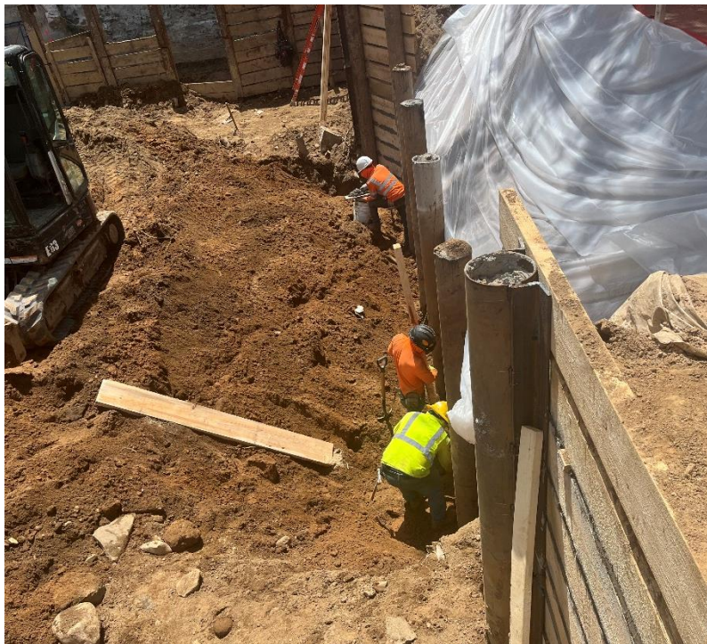
Photo 2: View of lagging along the western portion of site, facing south.
