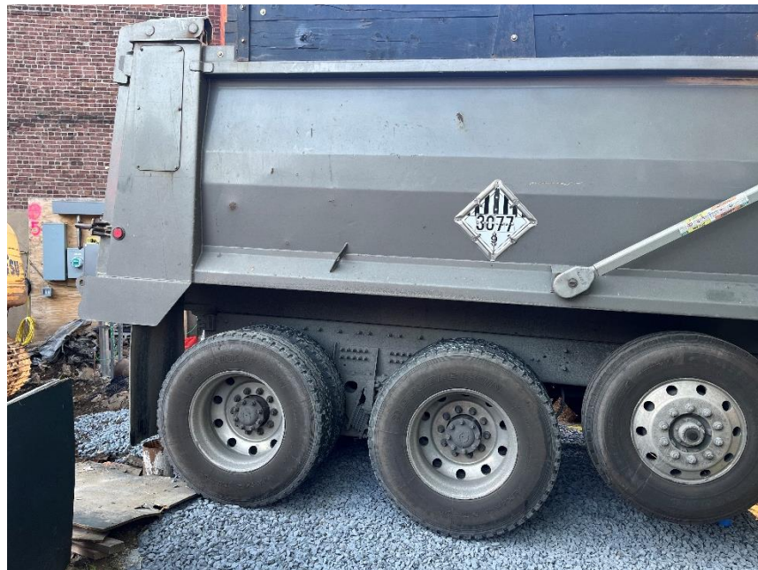
Photo 2: View of tri-axle truck backing onto site on stabilized construction entrance, facing south.
