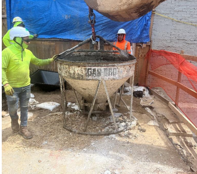
Photo 3: View of the contractor pouring concrete into SOE piles, facing southwest.
