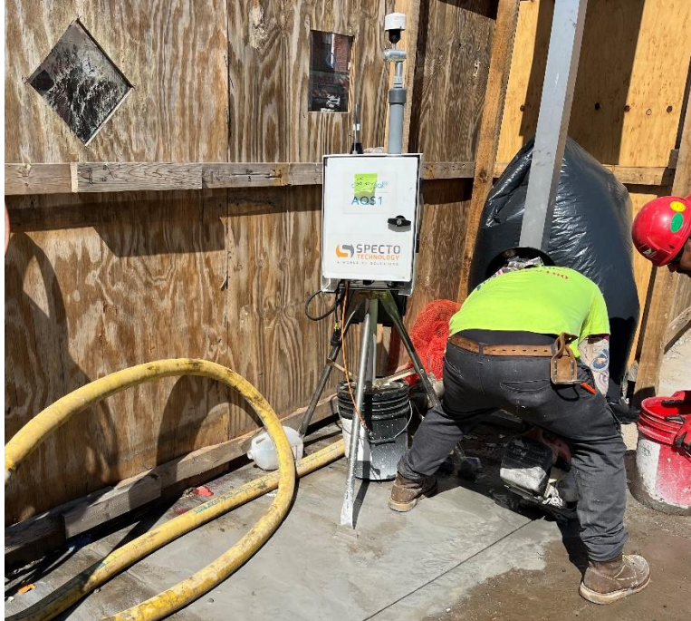
Photo 3: View of contractors saw cutting concrete and using water for dust suppression near CAMP Station 3, facing northeast.
