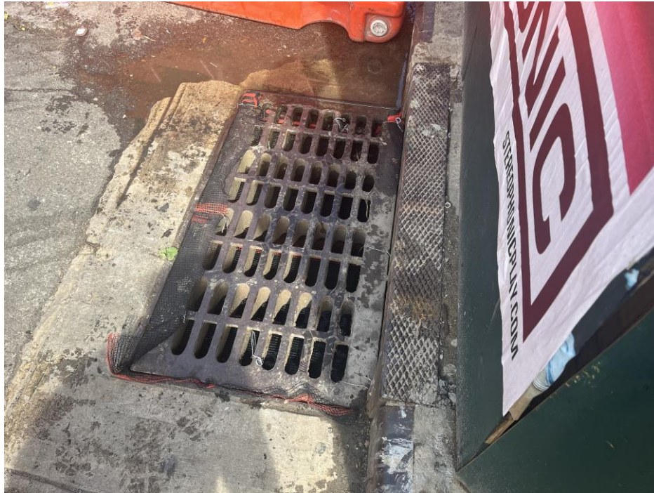
Photo 1: View of filter fabric installed in catch basin along Myrtle Avenue, facing east.
