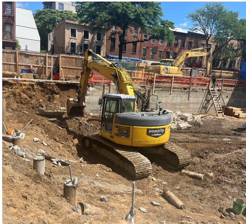
Photo 2: View of removal of northwest foundation wall, facing northeast.
