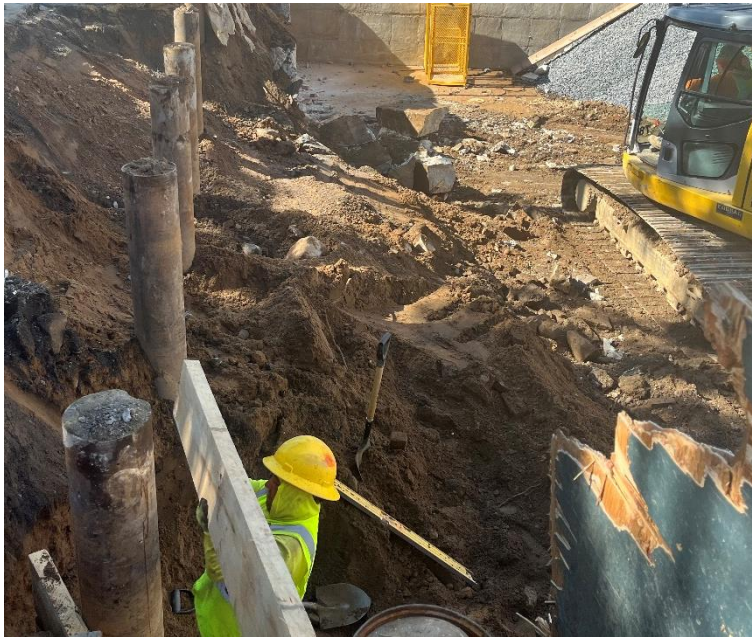
Photo 4: View of contractor installing SOE, facing north.
