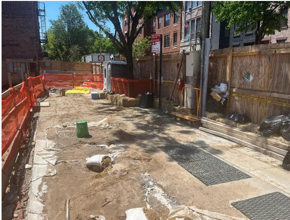
Photo 4: View of Site conditions and hay bales installed for erosion and sediment control along perimeter of the Site, facing south.
