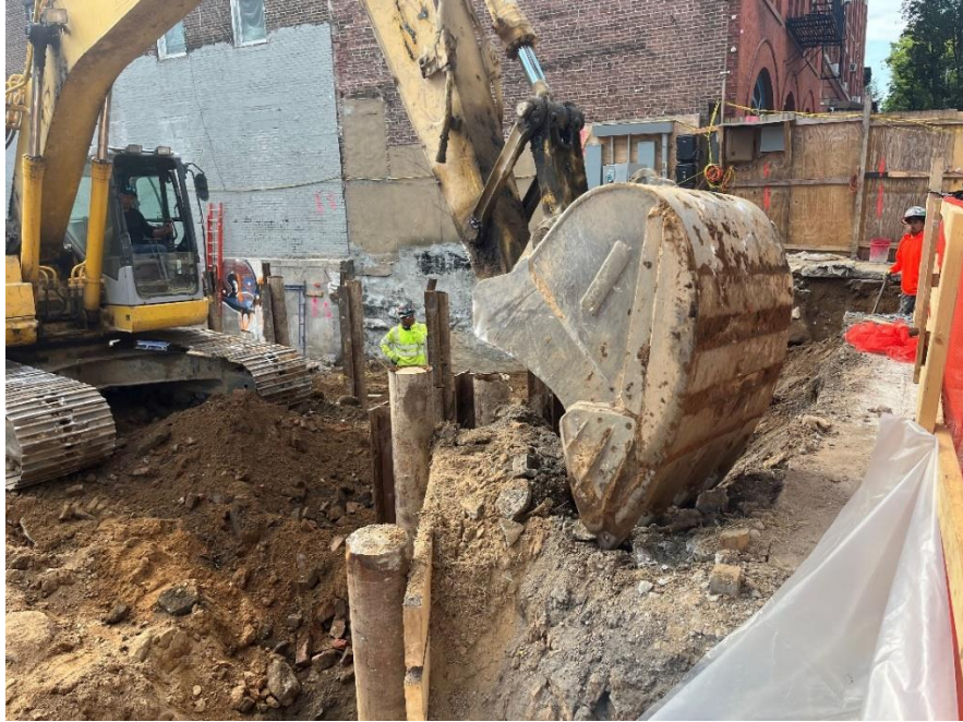
Photo 3: View of contractor excavating behind existing lagging in the western portion of the site, facing southeast.
