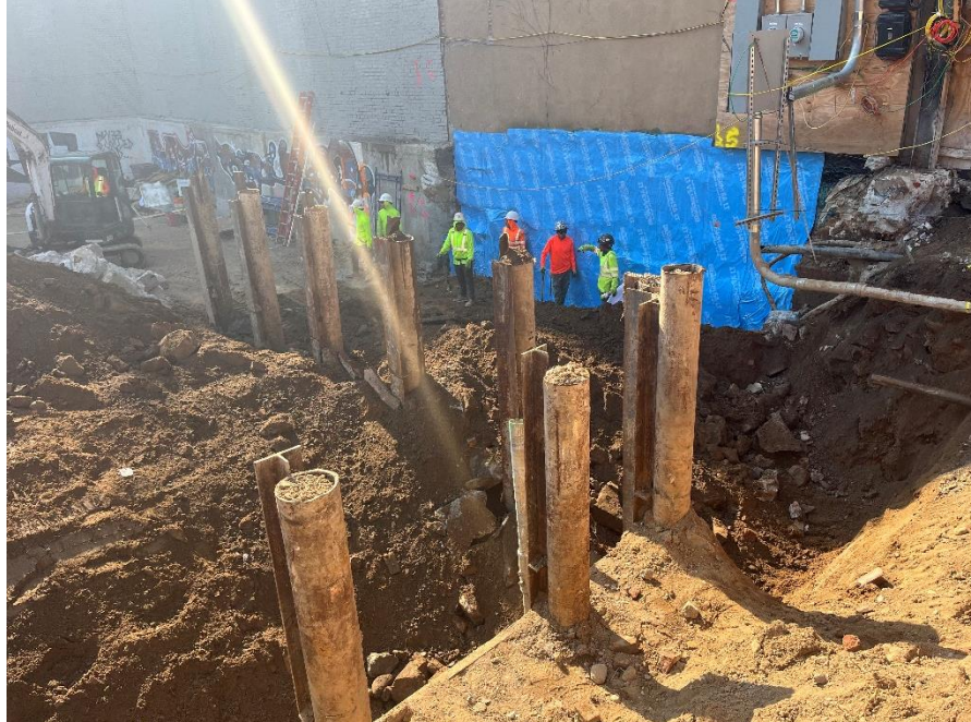
Photo 3: View of contractor applying waterproofing to the south adjacent property wall, facing southeast.
