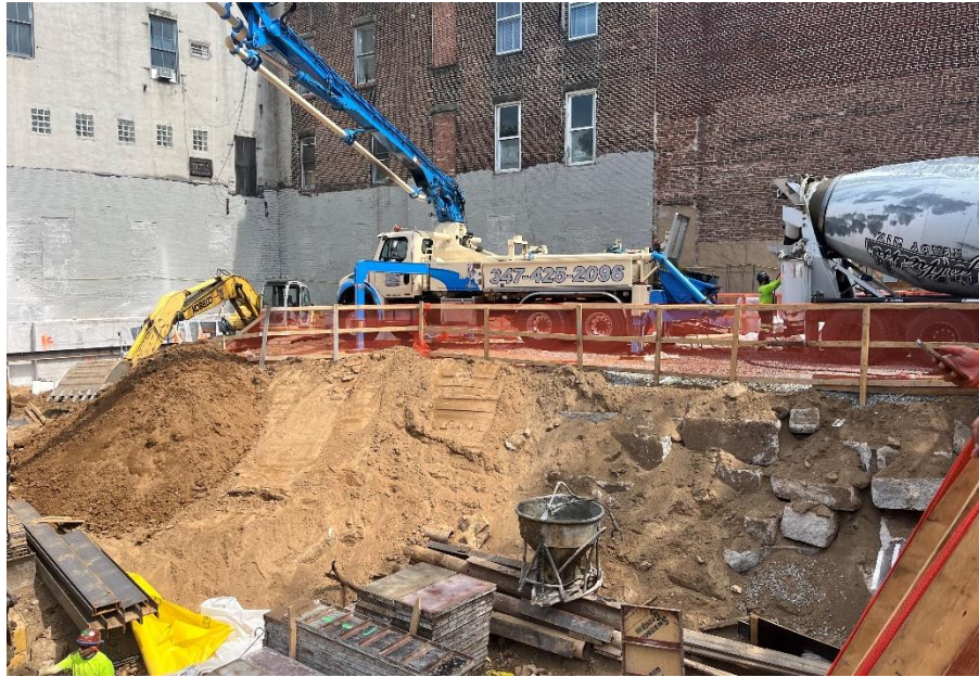
Photo 1: View of contractor preparing to pour concrete for SOE, facing southeast.
