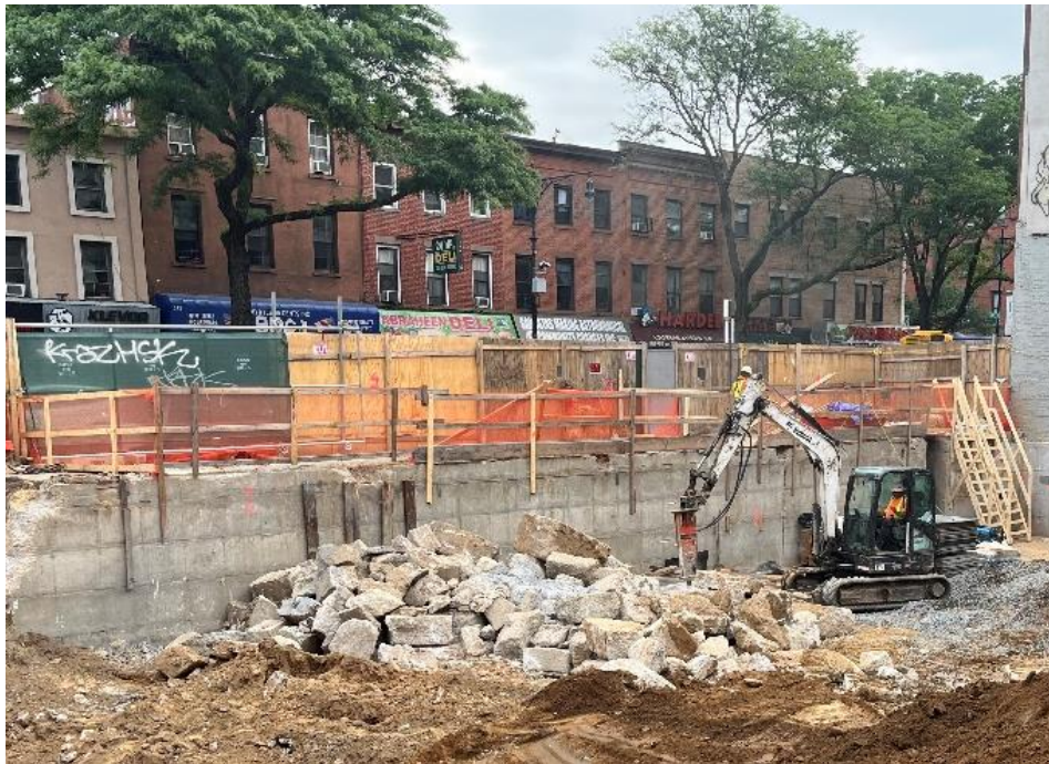
Photo 2: View of contractor breaking down concrete, facing northeast.
