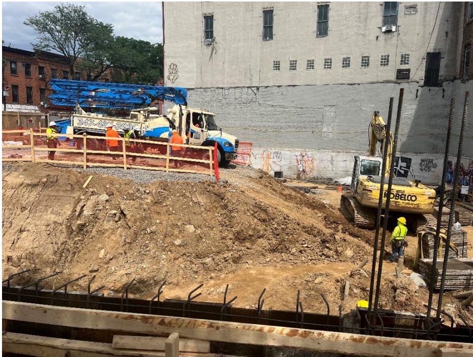
Photo 4: View of Site conditions and contractor prepping for concrete pour of foundation elements, facing east.
