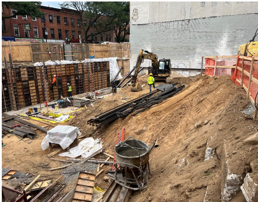
Photo 4: View of Site conditions and contractors installing SOE, facing northeast.
