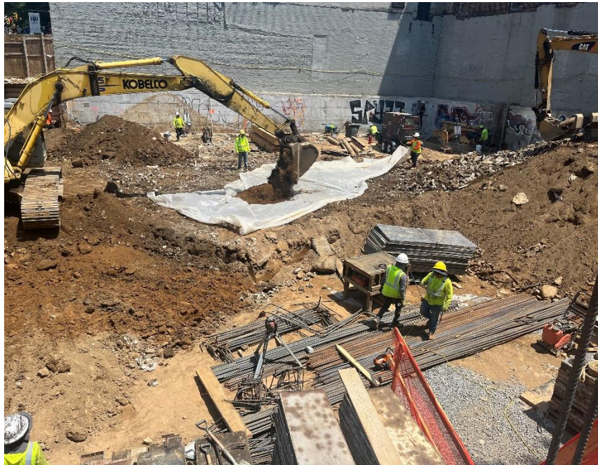
Photo 4: View of contractor stockpiling soil on poly, facing southeast.
