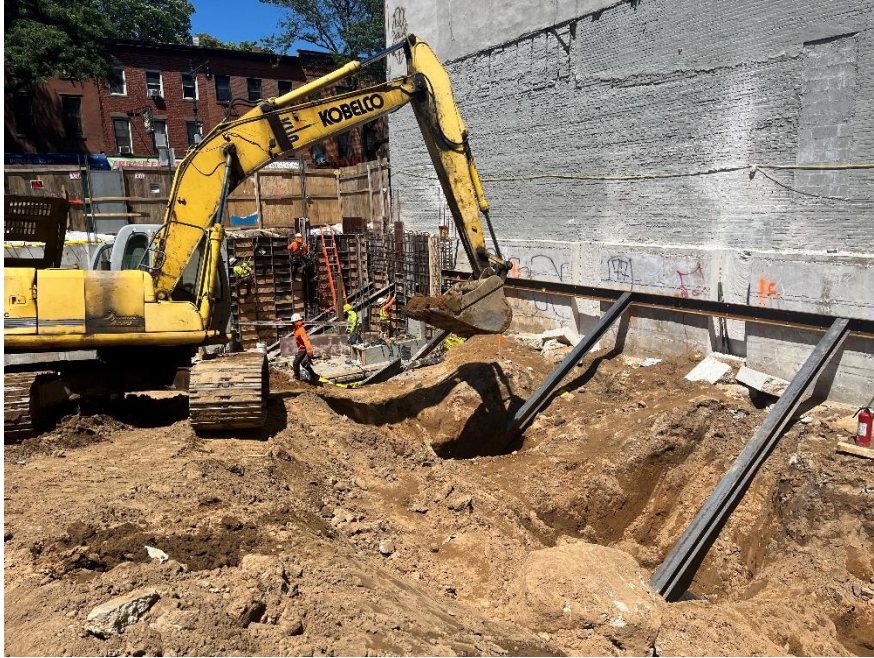
Photo 3: View of contractor installing SOE in northeastern portion of Site, facing northeast.
