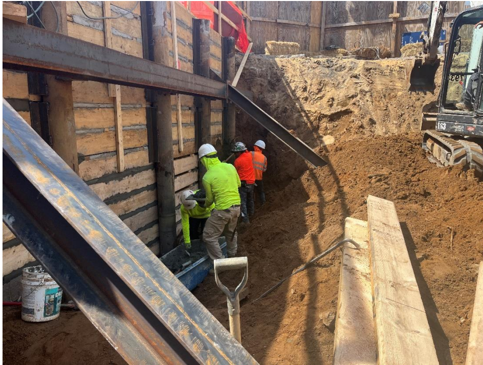
Photo 1: View of contractor installing lagging in western portion of site, facing north.
