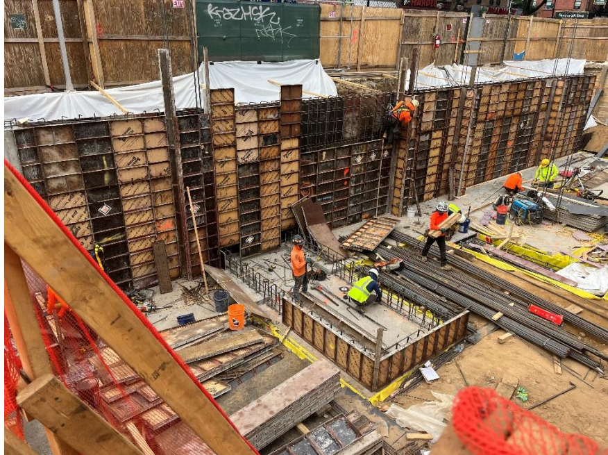
Photo 3: View of contractor installing SOE in northern portion of Site, facing northeast.
