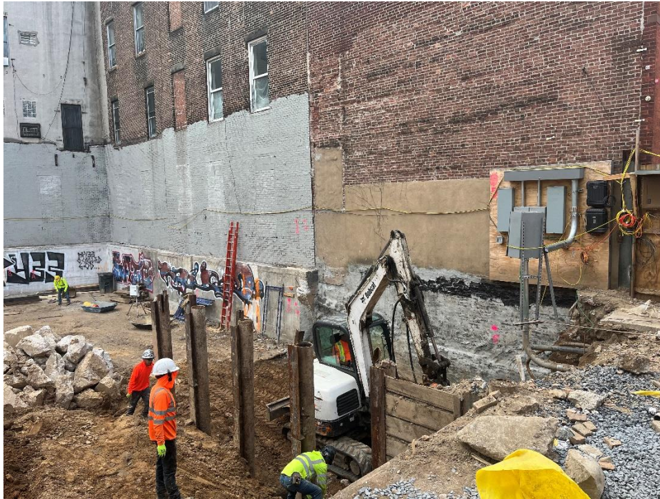
Photo 1: View of CAMP Station 1 and contractor removing existing lagging, facing southeast.
