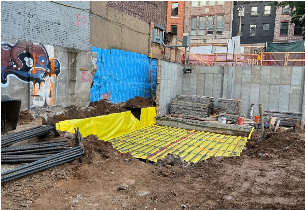
Photo 3: View of installation of building foundation elements and composite cover system, facing southwest.
