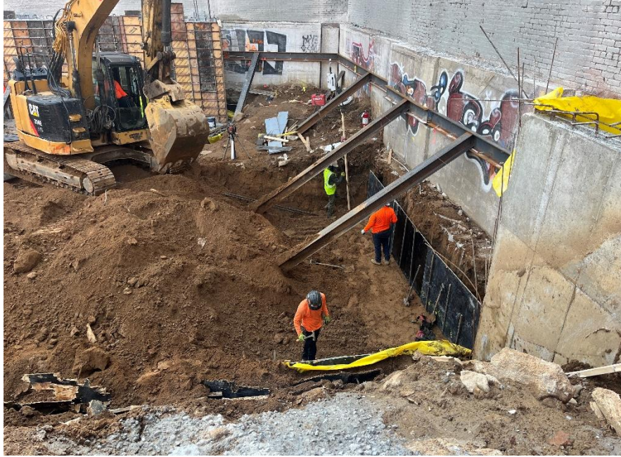
Photo 3: View of contractor preparing to install footing along southern portion of Site, facing east.
