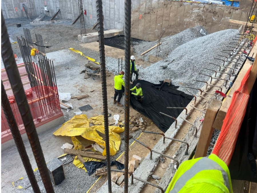
Photo 3: View of contractor installing geotextile fabric, facing southeast.
