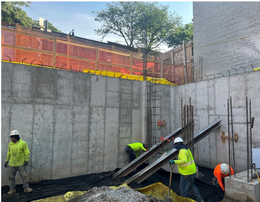
Photo 2: View of contractor installing geotextile fabric, facing northeast.
