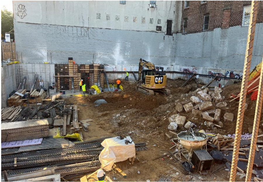
Photo 1: View of Site conditions and contractor installing SOE along eastern portion of Site, facing southeast.
