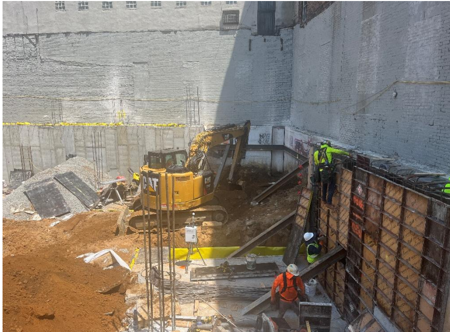
Photo 3: View of contractor preparing for footing and installing SOE along southern portion of Site, facing east.
