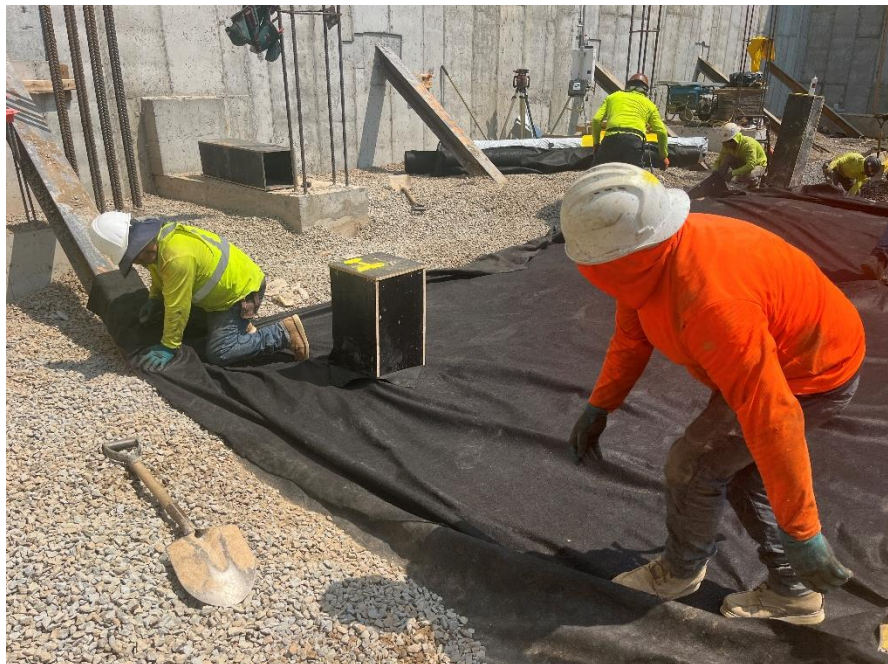
Photo 4: View of contractor installing geotextile fabric, facing southeast.
