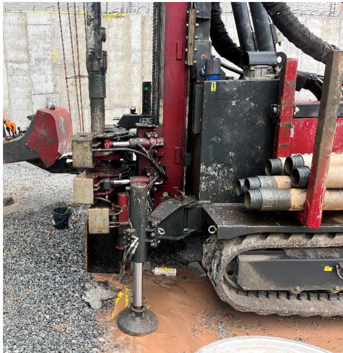
Photo 2: View of contractor installing injection well IW-08, facing south.
