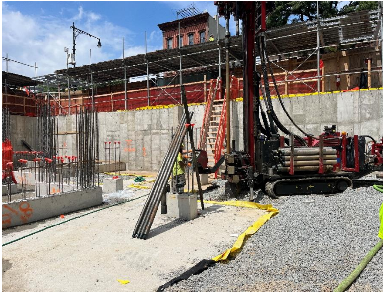
Photo 1: View of contractor installing injection well IW-02, facing north.
