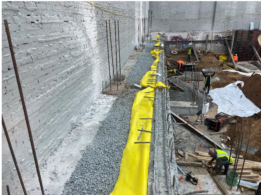
Photo 2: View of #57 Stone behind SOE Wall along eastern portion of Site, facing south.
