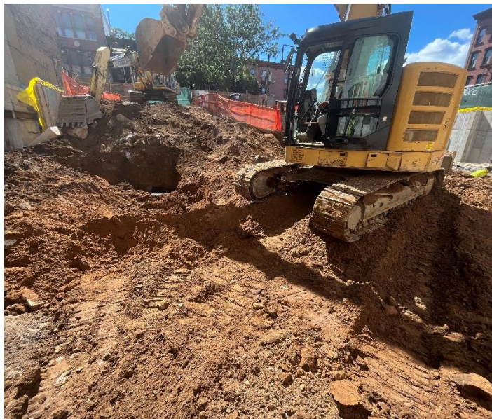
Photo 4: View of contractors grading Site soils along southern portion of Site, facing west.
