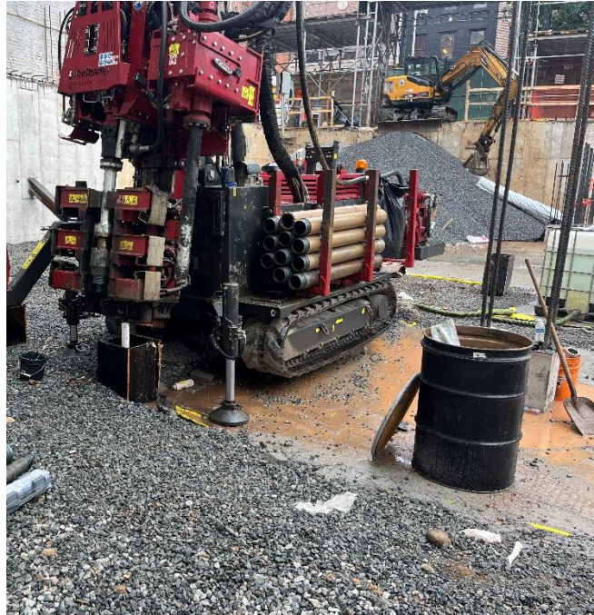
Photo 3: View of contractor installing injection well IW-08, facing west.
