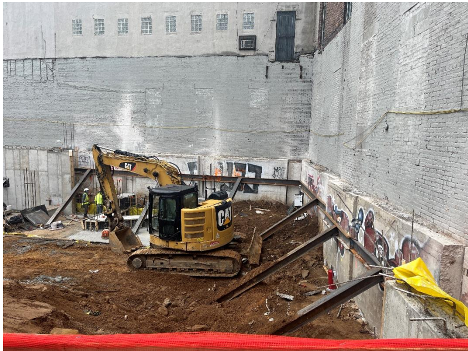
Photo 2: View of contractor preparing for SOE installation along southern portion of Site, facing east.
