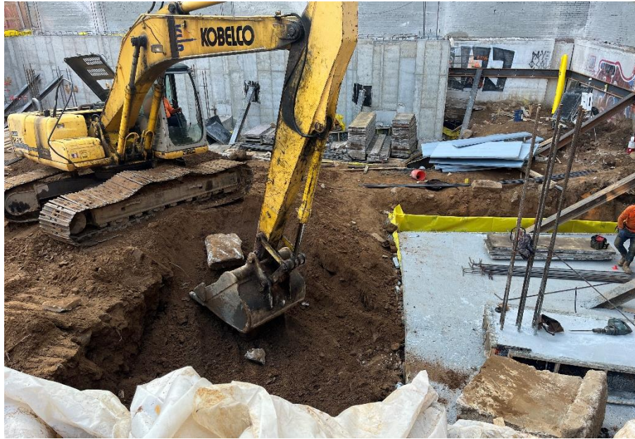
Photo 1: View of contractor preparing for SOE installation, facing east.
