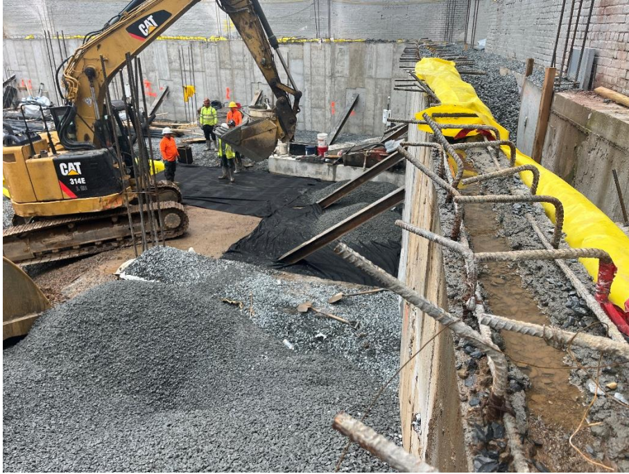
Photo 1: View of contractor installing geotextile fabric, facing east.
