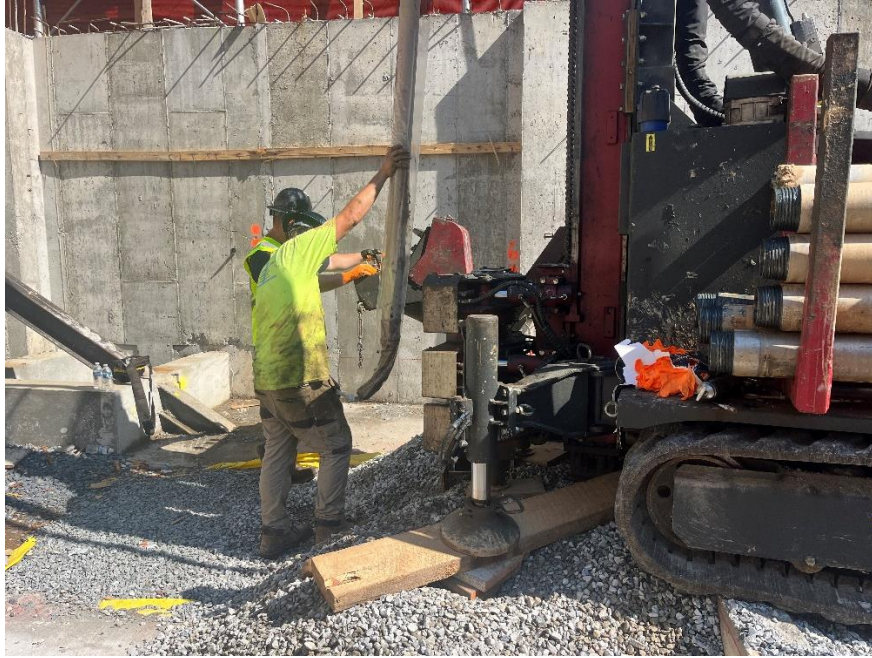
Photo 1: View of contractor beginning installation of injection well IW-01, facing north.
