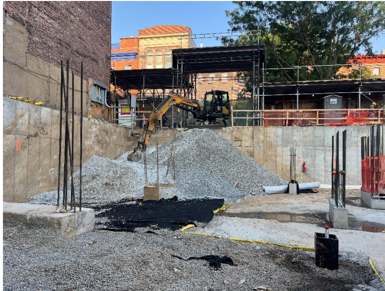
Photo 1: View of Site conditions, facing west.
