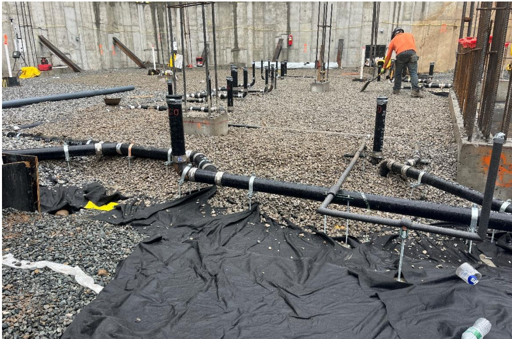
Photo 2: View of the contractor installing the SSDS, facing south.
