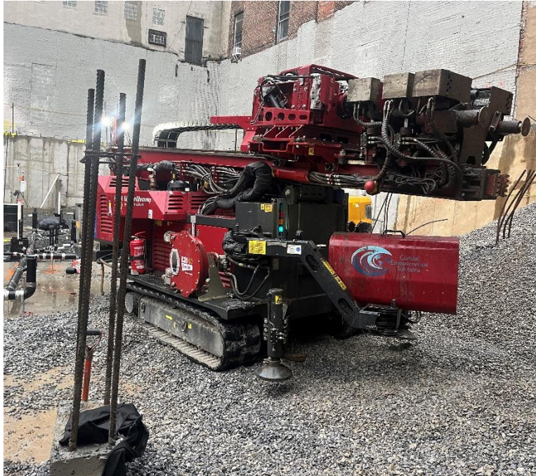
Photo 3: View of contractor preparing to install Injection Well IW-06, facing southeast.
