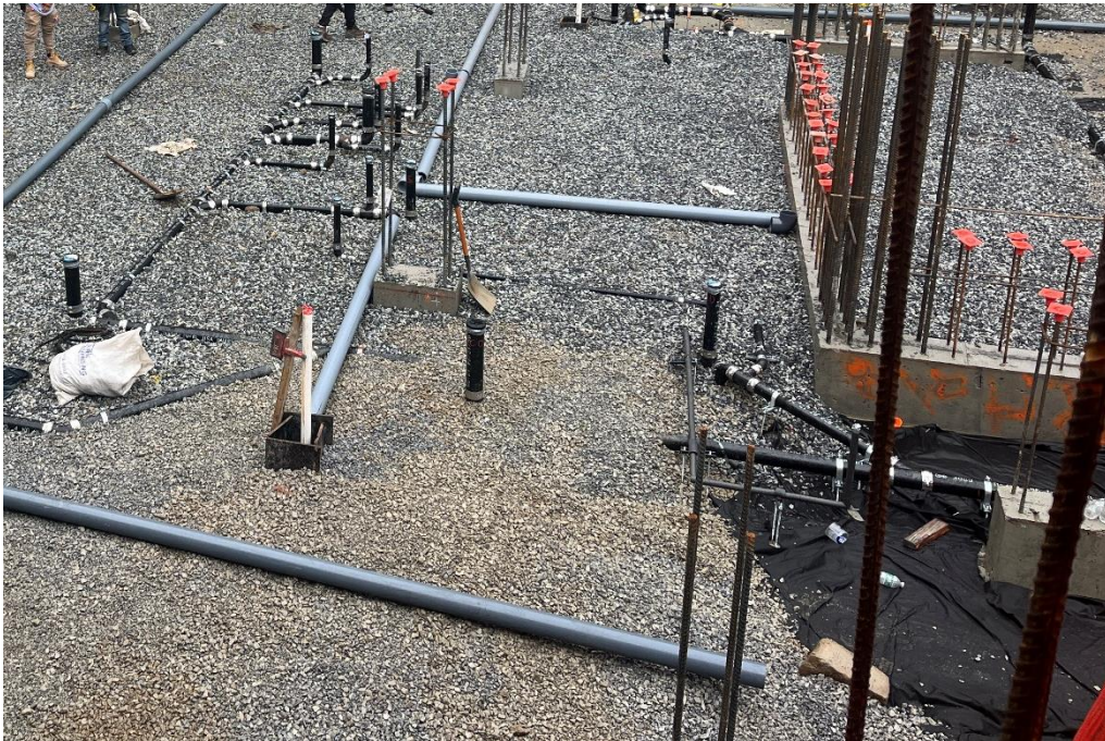
Photo 1: View of SSDS piping being laid out for installation, facing south.
