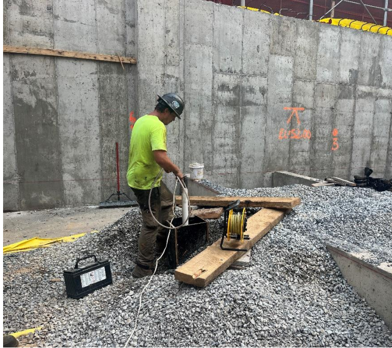
Photo 3: View of contractor developing IW-04, facing north.
