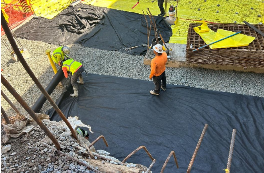
Photo 1: View the contractor installing the SSDS, facing east.
