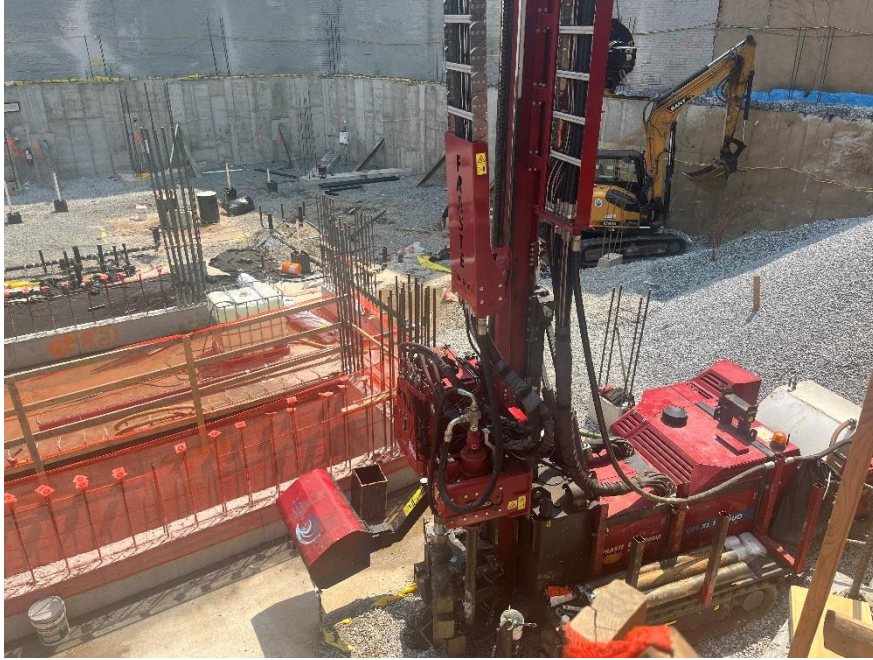
Photo 1: View of contractor installing injection well IW-04, facing southeast.
