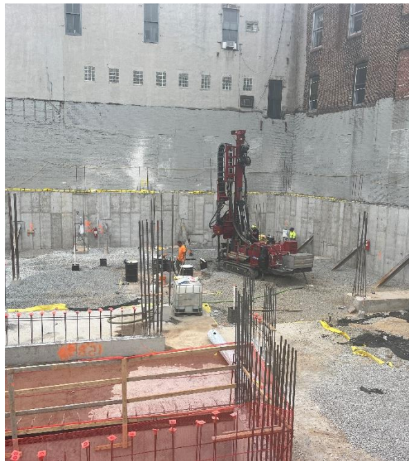
Photo 4: View of Site conditions, facing east.
