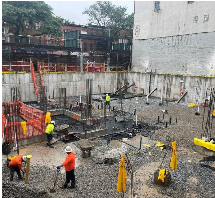
Photo 3: View of the contractor installing the SSDS layer, facing northeast.
