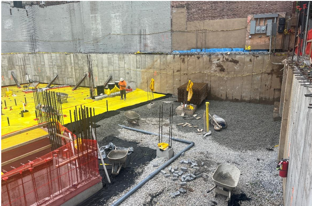
Photo 2: View of the SSDS layer during installation, facing south-southwest.
