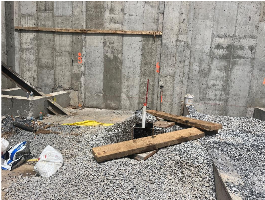
Photo 2: View of IW-01 installed, facing north.
