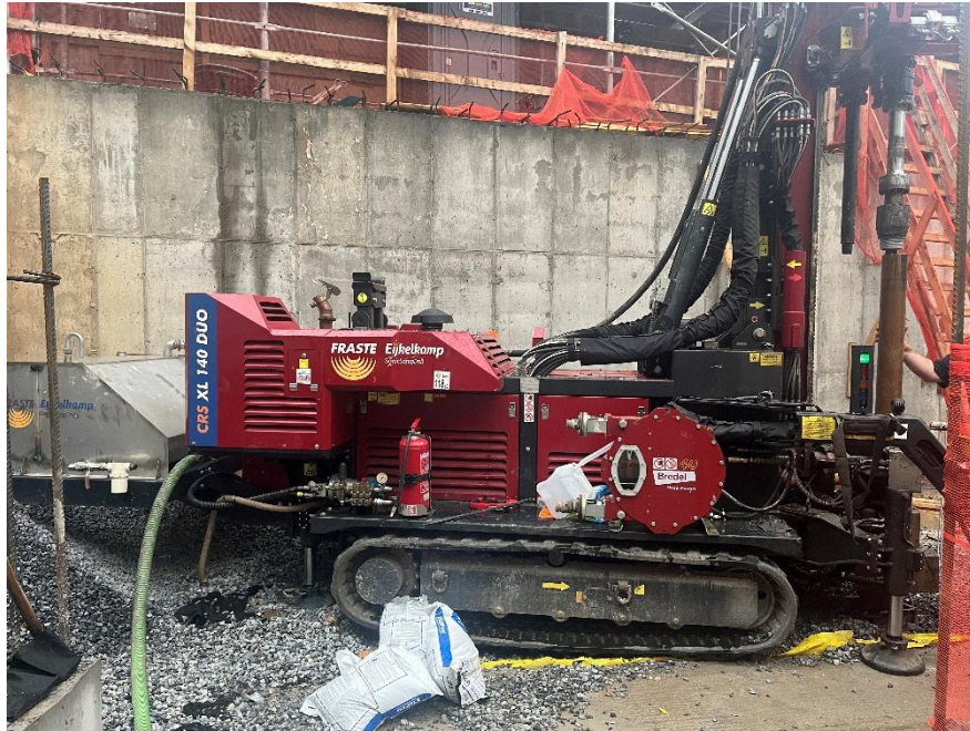
Photo 1: View of contractor installing injection well IW-04, facing west-northwest.
