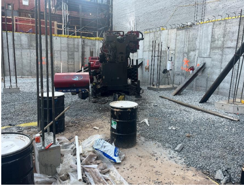
Photo 1: View of contractor re-installing monitoring well MW-6, facing northeast.
