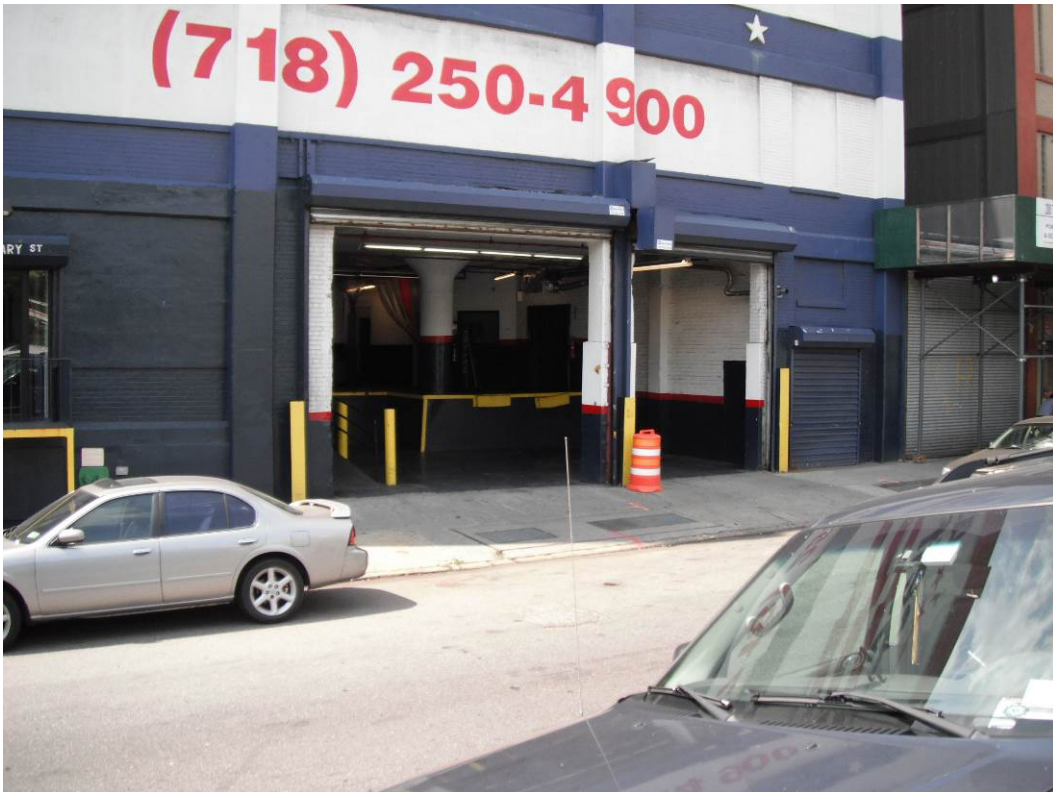
Photograph 6: View of the northern entrance of the subject site, facing south.
