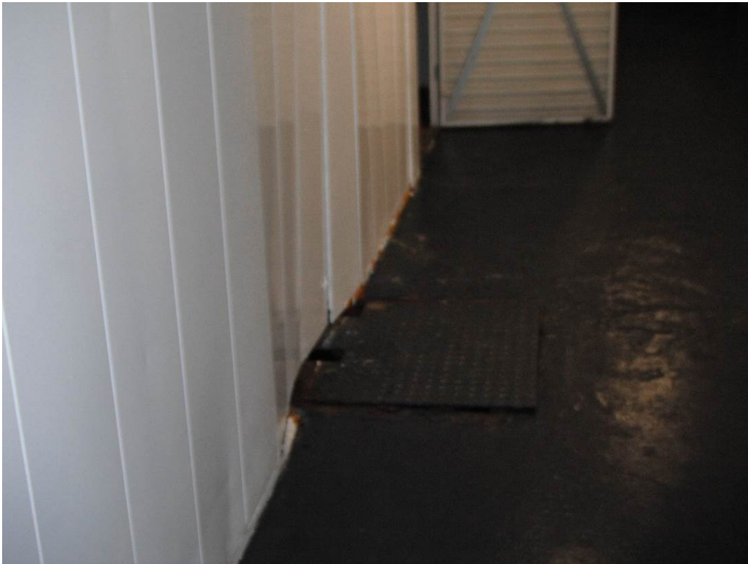
Photograph 8: View of the sump on the north side of the basement.
