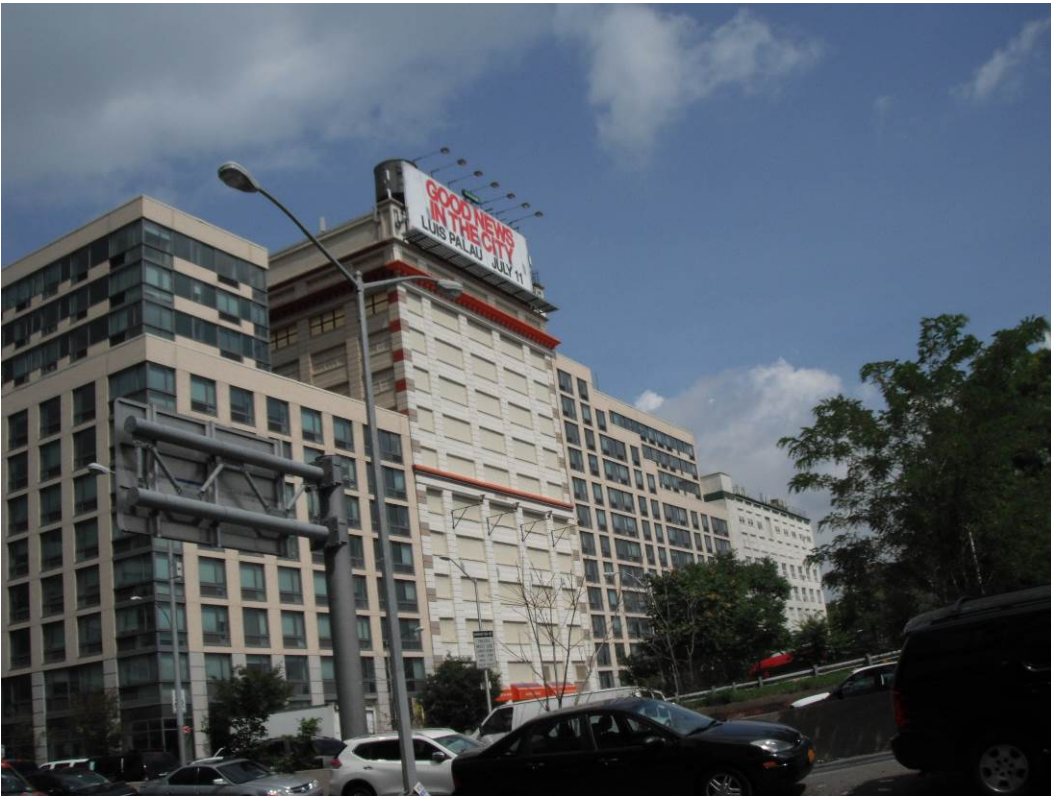
Photograph 9: View of Tillary Street and the property to the north of the subject site, facing north.
