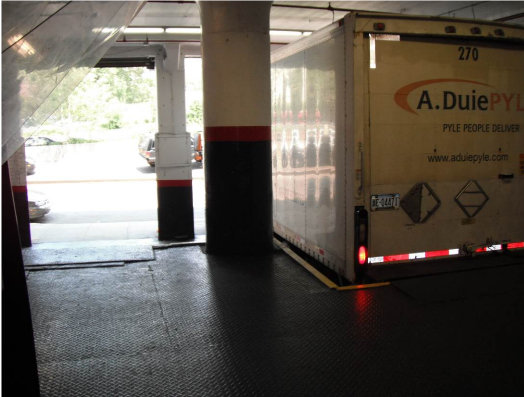
Photograph 5: View of the loading dock at the front gate entrance, facing north.
