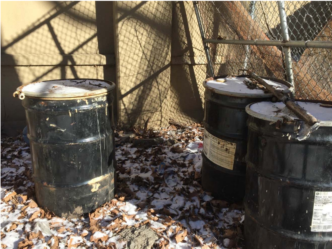
Photograph 9: View of three (3) 55-gallon metal drums located along the southern boundary of the site.
