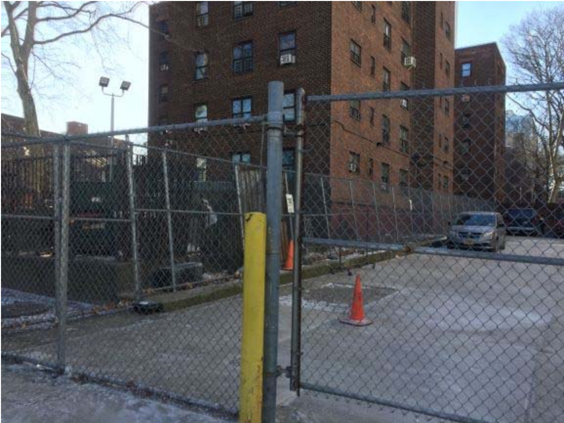
Photograph 2: View of the subject property adjacent south of Tillary Street, facing southeast. Note the area of uneven patched concrete in the foreground.
