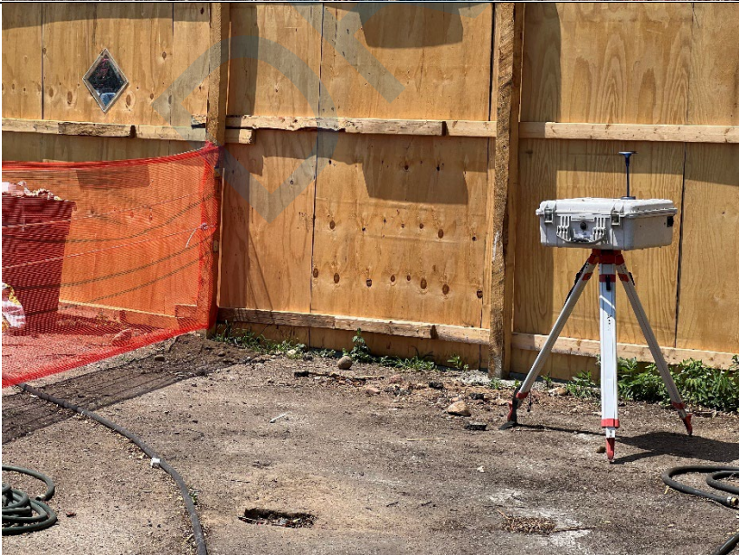
Photo 4: Looking east; view of the upwind CAMP station.
