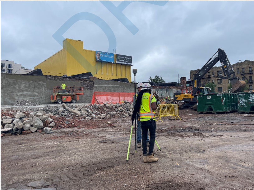
Photo 4: Looking southeast; view of Fehringer Surveying PC performing gaging location data.
