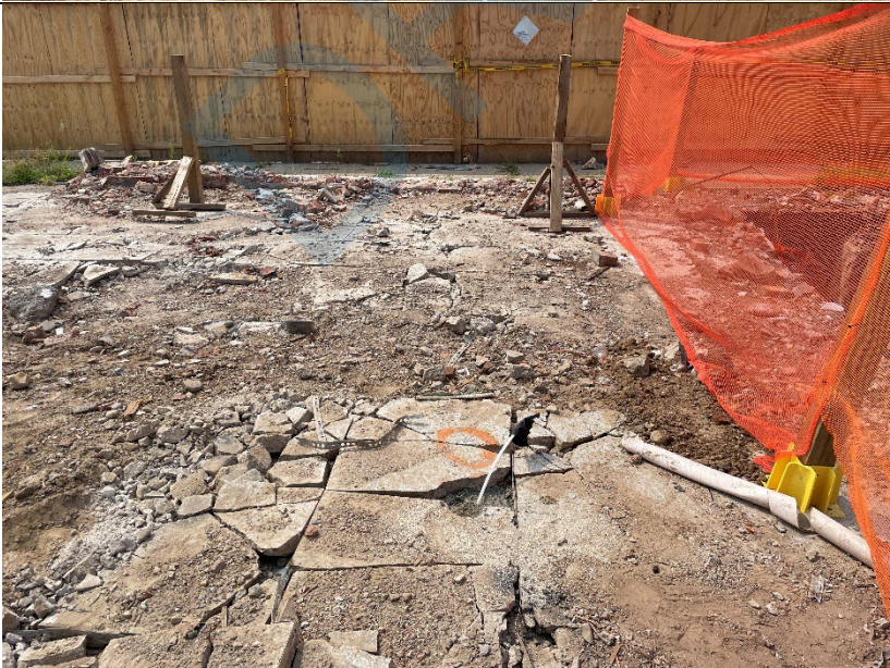
Photo 4: Looking south; view of RXSB-1 positioned outside the southwest basement exclusion zone.
