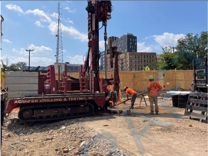
Photo 1: Looking east; ADT coring through at RXSB-11.
