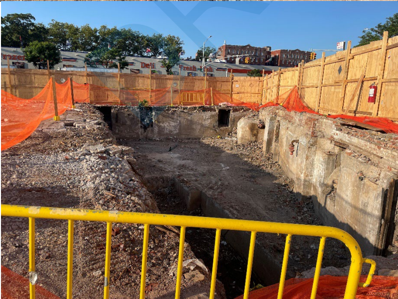
Photo 2: Looking south; view of fenced off basement area in the southwest corner of the site.
