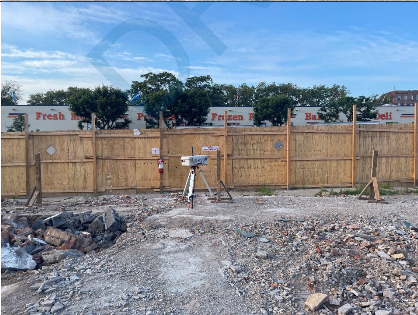
Photo 4: Looking south; view of the downwind CAMP station.
