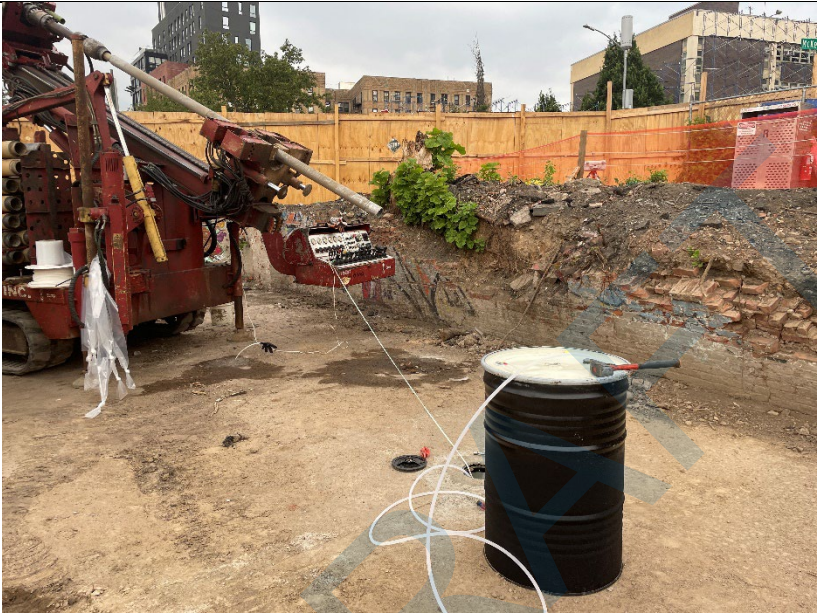
Photo 3: Looking northwest; view of ADT developing MW-2.
