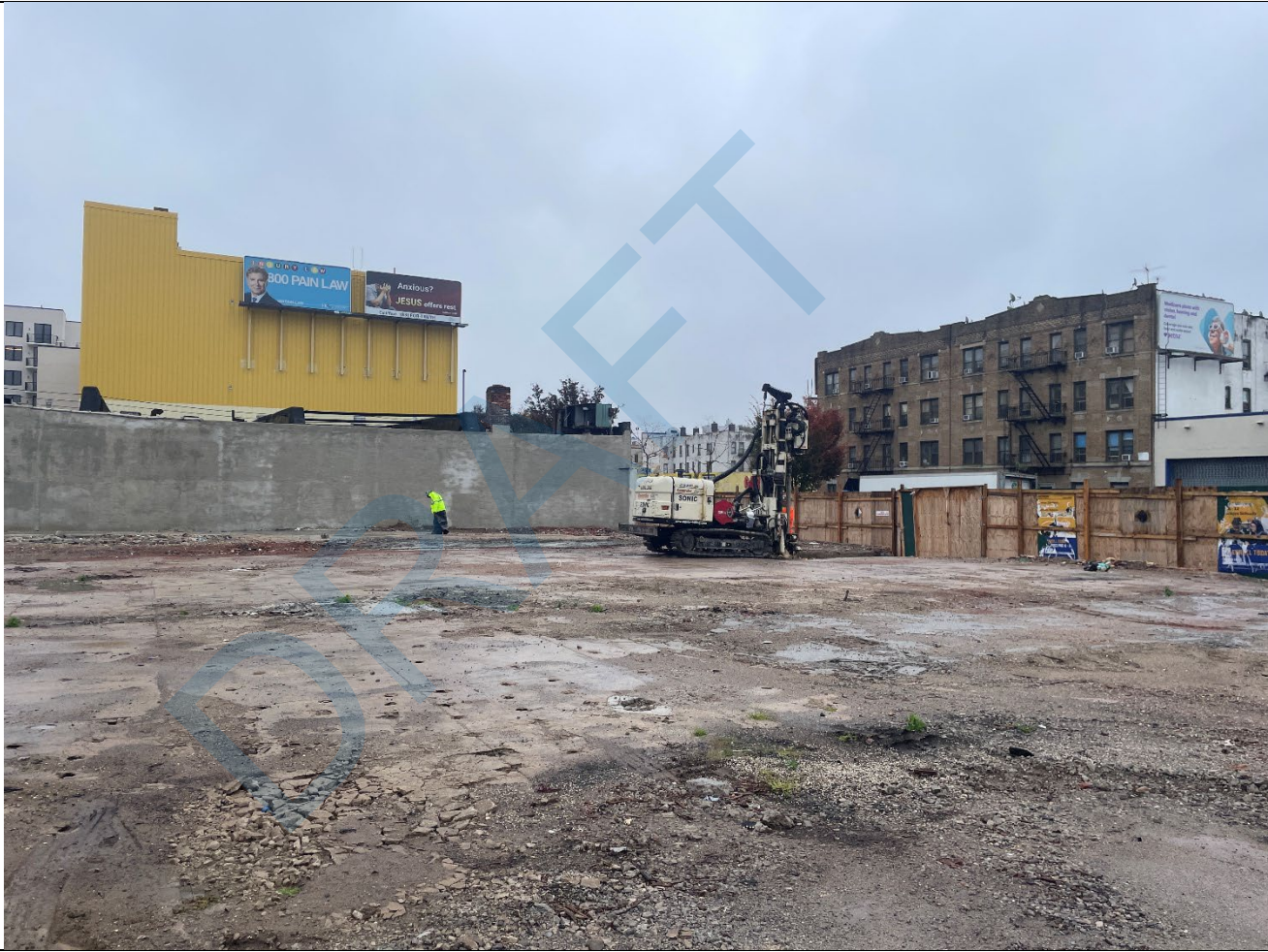
Photo 2: Looking southeast; view of ADT sonic drill at SRI-12.
