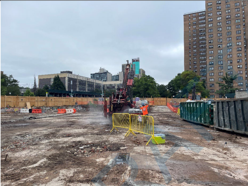
Photo 3: Looking northwest; view of ADT demobilizing following completion of work.
