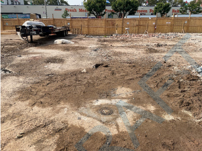
Photo 2: Looking south; view of manhole for MW-3.
