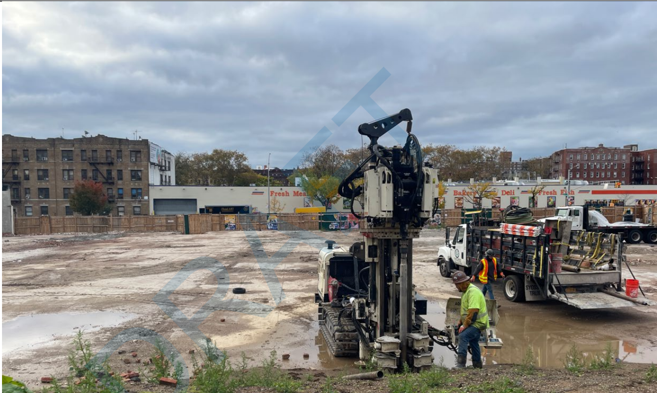
Photo 4: View of drilling operations.
