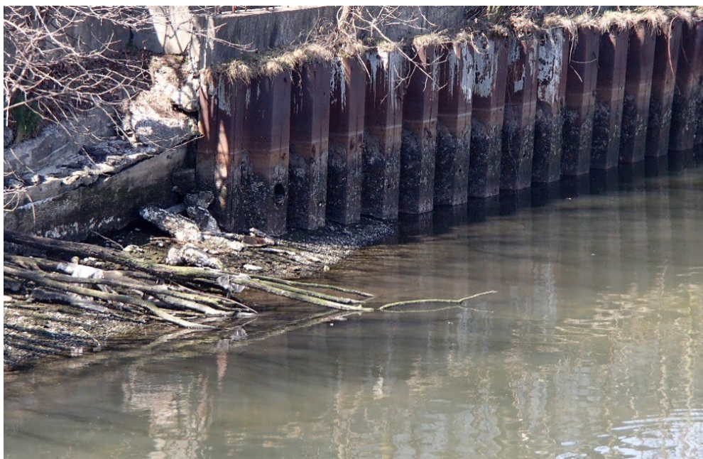
Photograph 8: Outfall pipe in bulkhead.
