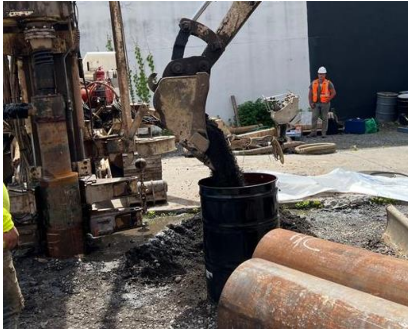
Photo 1: Allstate 12 excavating temporary sump and placing soil/fill into drums (facing east)
