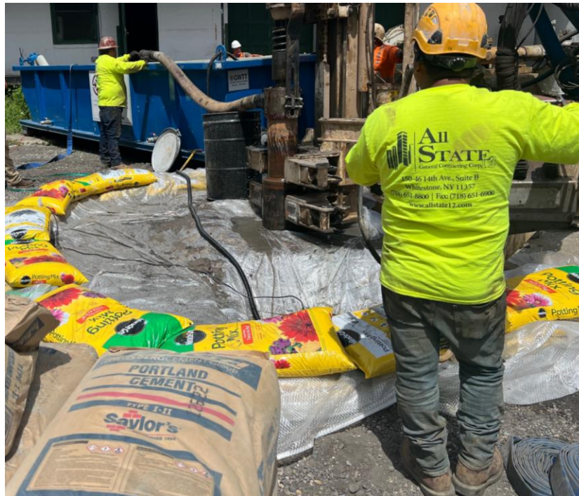
Photo 2: Polyethylene sheeting-lined sump at P-1 and settling tank (facing north)
