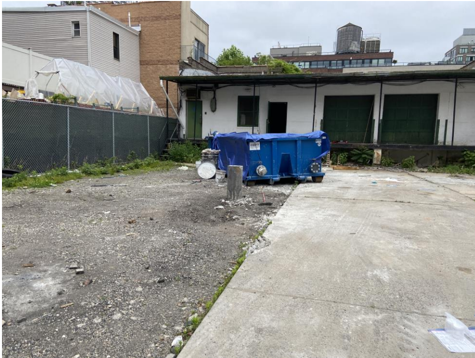
Photo 1: Settling tank in the southern part of the site (facing north)
