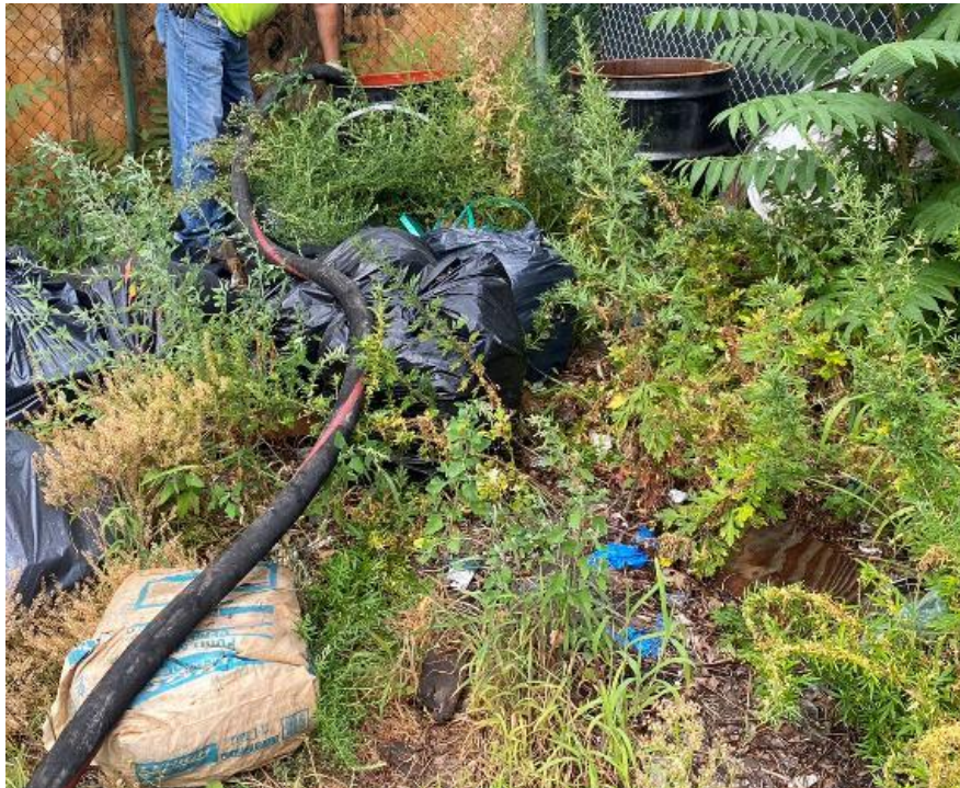
Photo 2: Liquid being pumped from a 55-gallon drum into a vacuum truck for offsite disposal (facing southwest)
