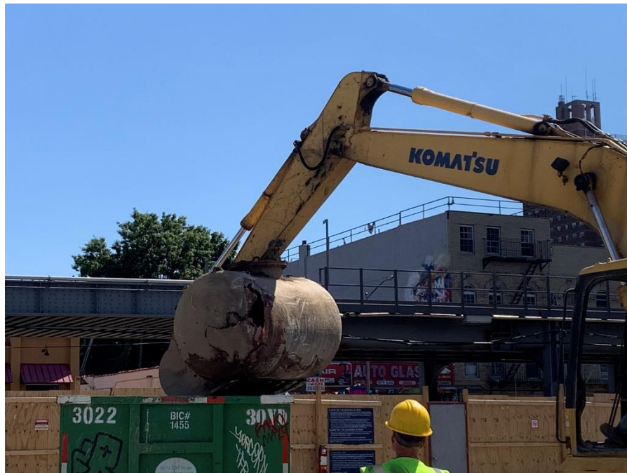
Photo 2: View of Contractor removing a 550-gallon UST, facing south
