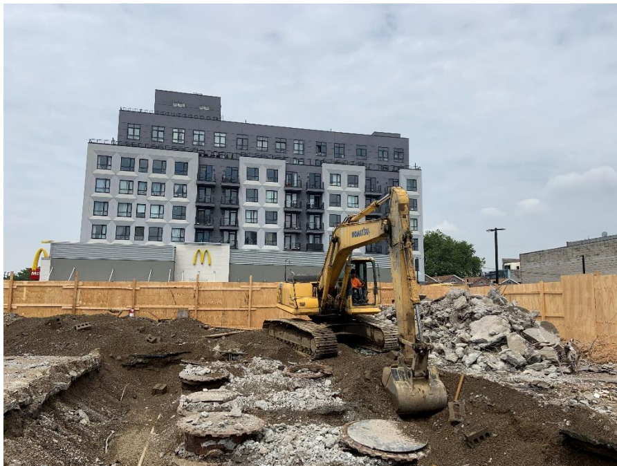
Photo 2: View of contractor exposing the underground storage tanks, facing west.
