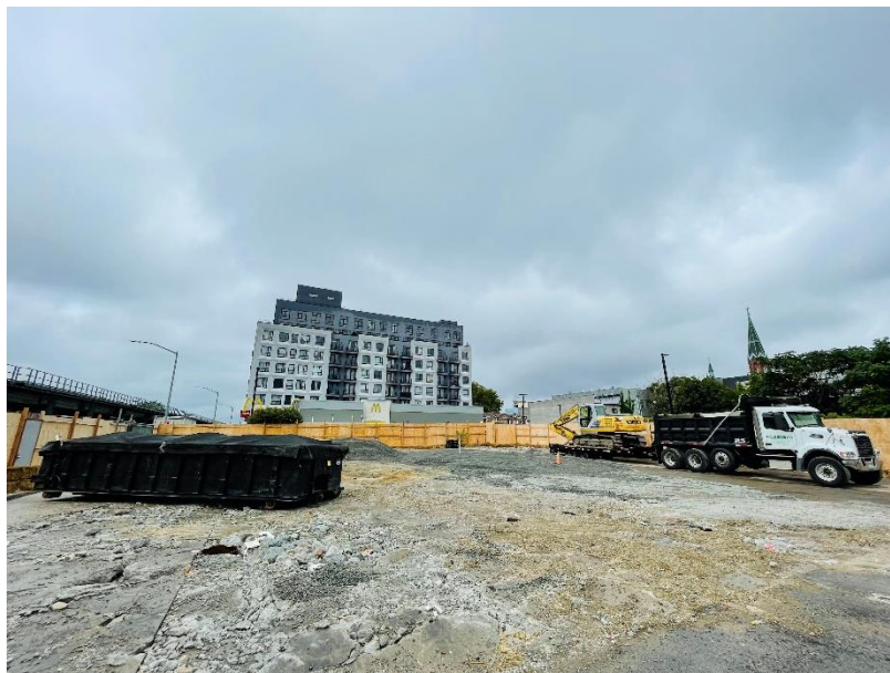
Photo 2: View of site after backfilling activity, facing West.
