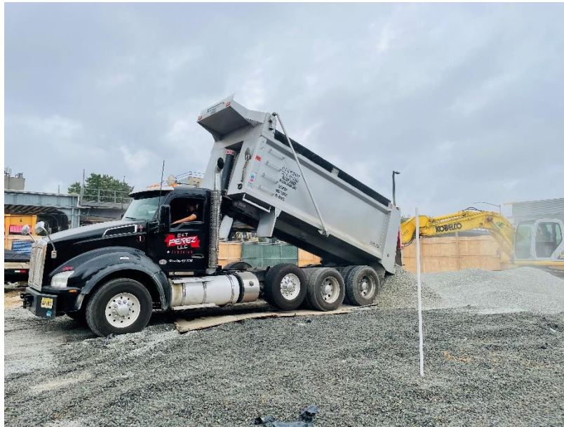
Photo 1: View of truck loading off stone to the site, facing Southwest.
