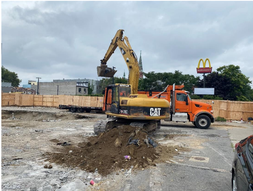
Photo 1: View of contractor loading soil for disposal, facing north.
