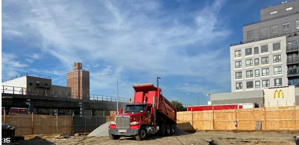
Photo 1: View of crushed stone unloading, facing southwest
