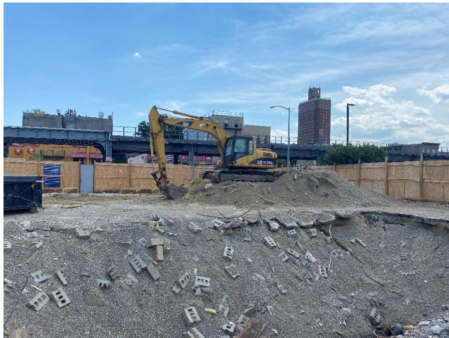
Photo 2: View of the contractor consolidating the stockpile, facing southwest.
