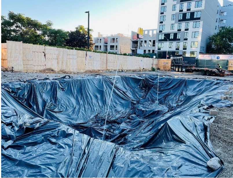
Photo 1: View of UST excavation area before backfilling, facing Northeast.
