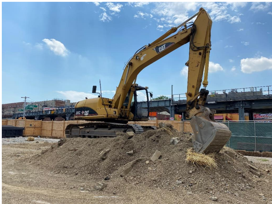
Photo 2: View of the contractor consolidating the stockpile, facing southeast.
