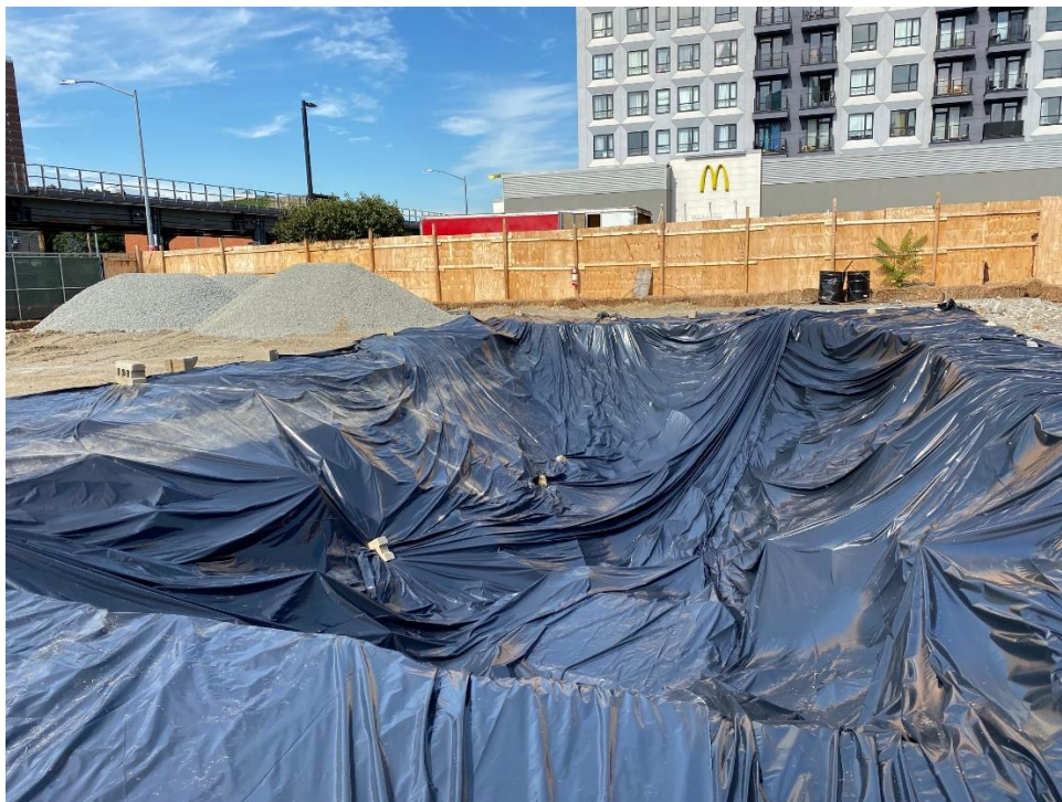
Photo 2: View of poly-lined excavation and background stone stockpile, facing southwest.
