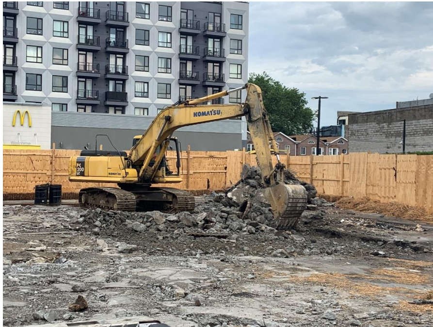
Photo 1: View of contractor removing concrete slab, facing northwest.
