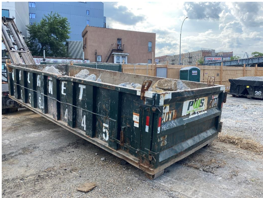
Photo 2: View of Planet Waste removing concrete debris dumpster, facing southeast.
