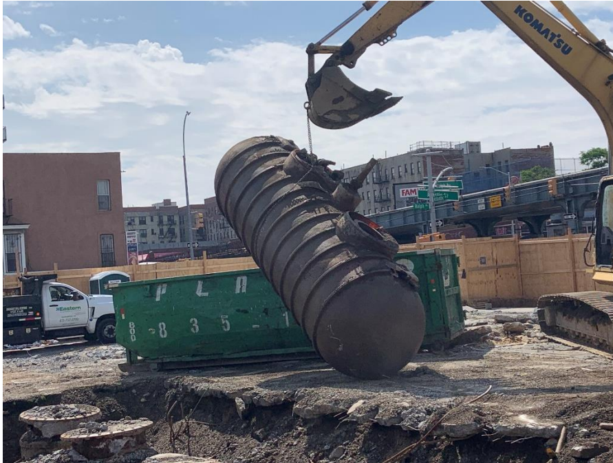
Photo 1: View of contractor removing a 4,000-gallon UST, facing southeast.
