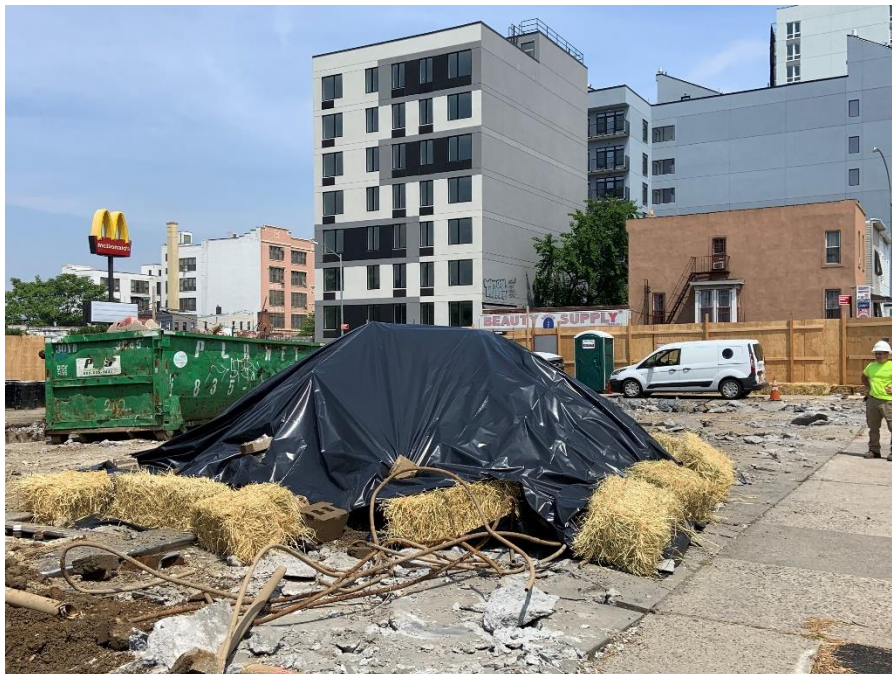
Photo 2: View of stockpile covered with polyurethane sheeting and surrounded with hay bales, facing east.
