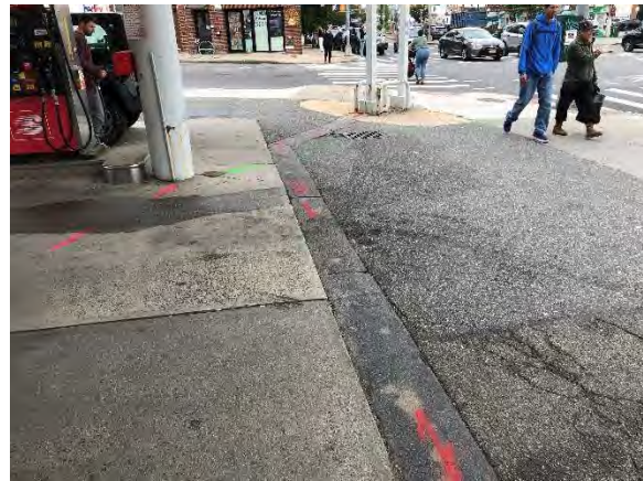
Photo an electric line(red), a storm line(green) and also an unknown line(pink).
