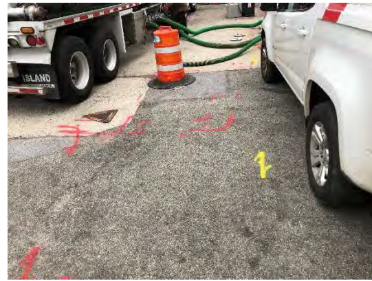
Photo of a gas line(yellow) and several electric lines(red)
