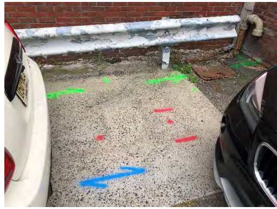
Photo of electric service line(red), water service line(blue), and sewer line(green) being fed from the street
