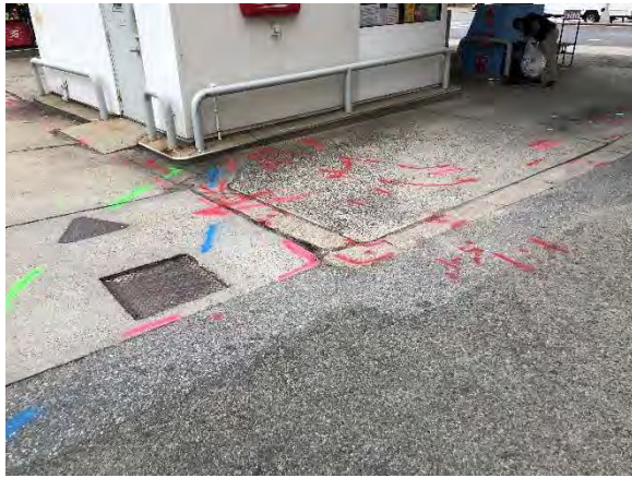
Photo of multiple electric lines(red) along with a water line(blue) and sewer line(green).
