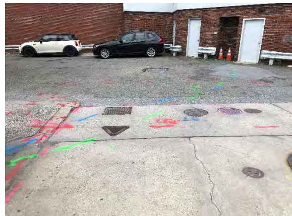
Photo of electric(red), water(blue), and sewer lines(green) running between the buildings
