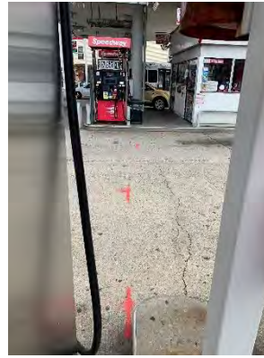
Picture 2: ELECTRICAL LINES GOING TO THE PUMPS.
