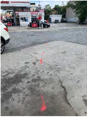
Picture 1: ELECTRICAL LINES FROM DIESEL TANK GOING BACK TO THE MAIN BUILDING.
